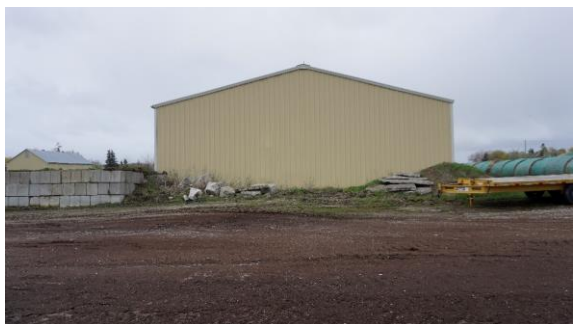
Photo 83: East outbuilding, east elevation looking west
