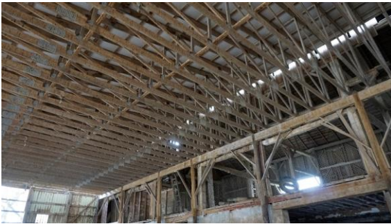
Photo 73: Addition wood framing with steel braces
