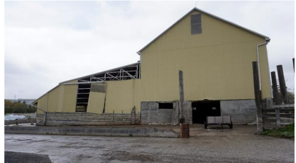
Photo 63: East elevation looking west
