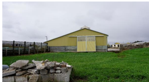
Photo 75: Cattle outbuilding, east elevation looking west
