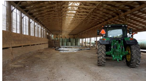
Photo 79: Cattle outbuilding, interior looking east
