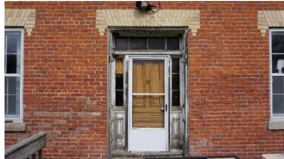
Photo 6: Front façade central entrance
