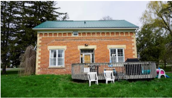
Photo 5: Front façade looking north
