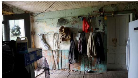
Photo 36: Rear addition looking south
