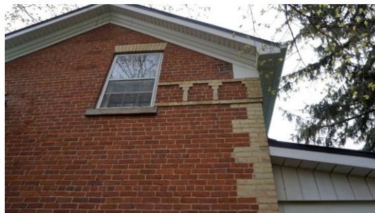
Photo 12: North elevation rear tail window
