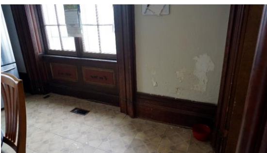
Photo 25: Front kitchen wood mouldings and panelling
