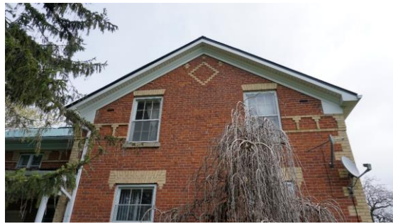
Photo 14: West elevation of gabled end
