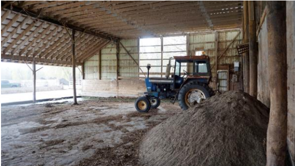
Photo 71: Addition looking southwest
