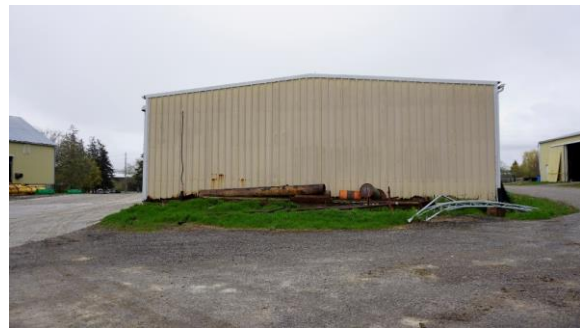
Photo 93: East elevation looking west
