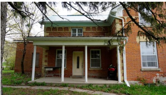
Photo 15: West elevation rear tail porch
