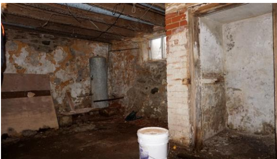
Photo 53: Basement looking southwest
