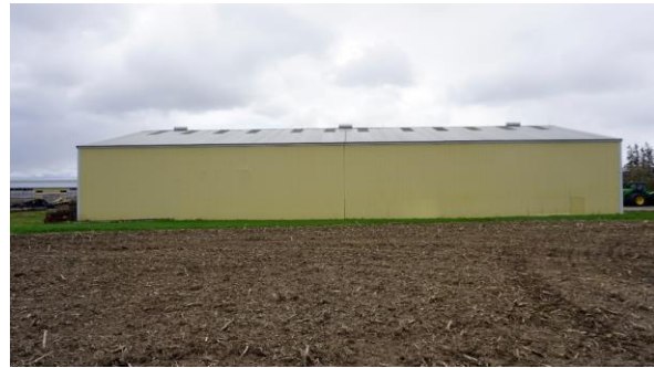
Photo 87: West outbuilding, north elevation looking south
