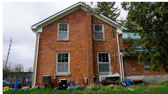
Photo 8: East elevation looking west
