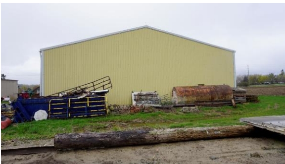
Photo 88: West outbuilding, east elevation looking west
