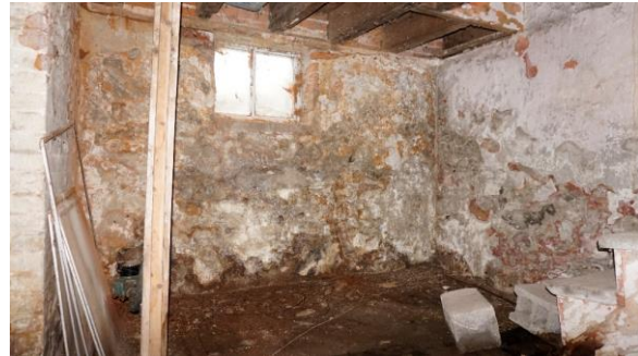
Photo 52: Basement looking northwest
