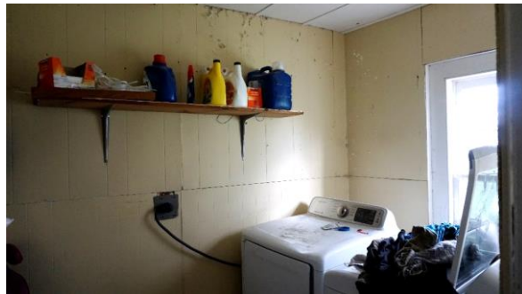
Photo 34: Rear tail laundry room looking northeast
