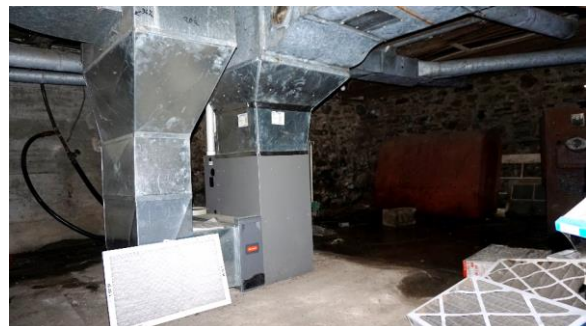
Photo 54: Basement looking southeast
