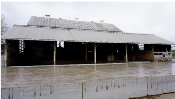
Photo 60: South elevation looking northeast
