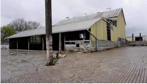
Photo 62: South and east elevations looking north
