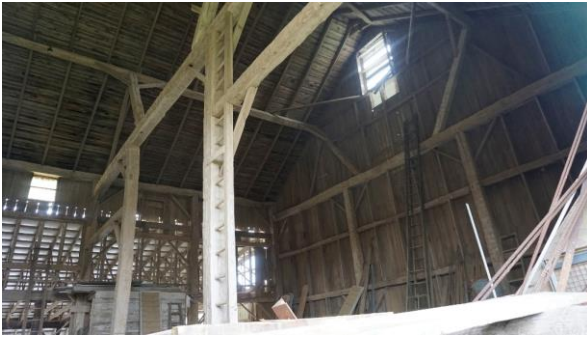
Photo 66: Upper storey looking southwest
