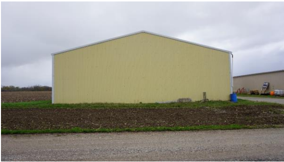
Photo 86: West outbuilding, west elevation looking east
