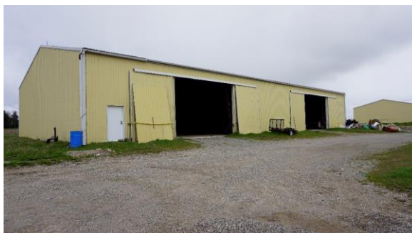
Photo 85: West outbuilding, south elevation looking northeast
