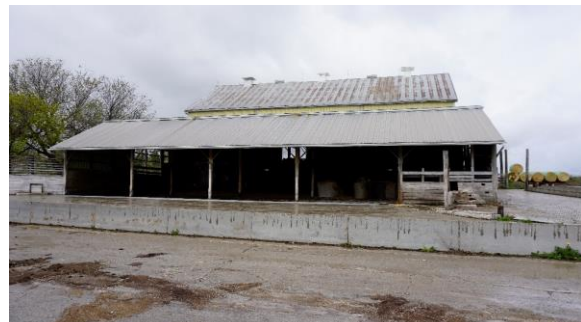
Photo 61: South elevation looking north
