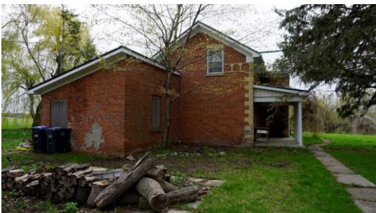
Photo 11: North elevation looking south
