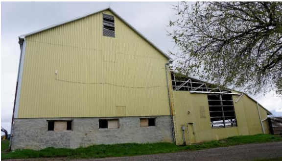
Photo 58: West elevation looking southeast
