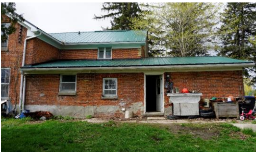
Photo 9: East elevation looking west
