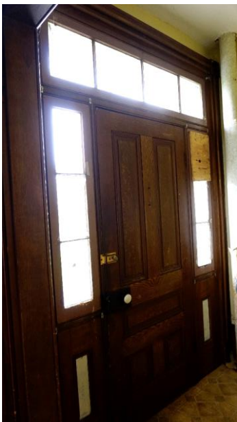
Photo 17: Front entry door
