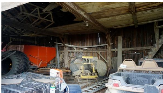
Photo 40: Driveshed interior, centre portion
