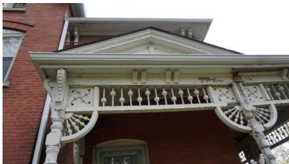
Photo 9: Detail of spindle work on the porch
