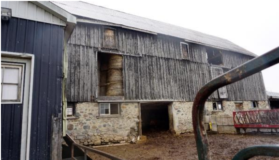
Photo 29: South elevation looking northeast
