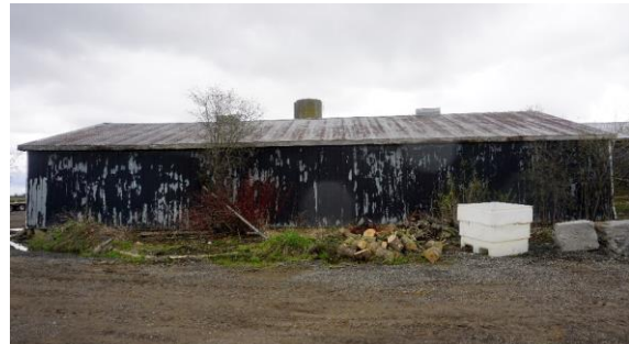
Photo 45: Storage driveshed, north elevation looking south
