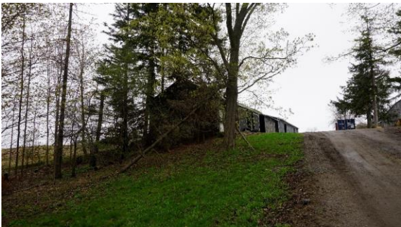
Photo 37: Driveshed west and south elevations looking northeast
