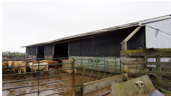
Photo 50: Cattle outbuilding north elevation looking southeast
