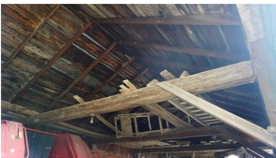
Photo 39: Driveshed interior, centre portion
