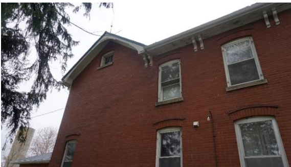
Photo 20: North elevation gabled bay looking southeast
