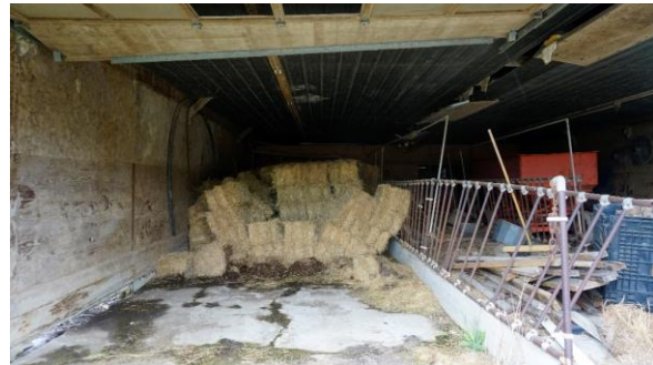
Photo 47: Storage driveshed, interior
