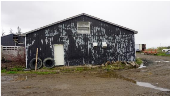
Photo 44: Storage driveshed, east elevation looking west
