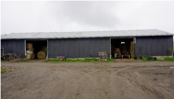
Photo 33: Driveshed south elevation, east portion looking north
