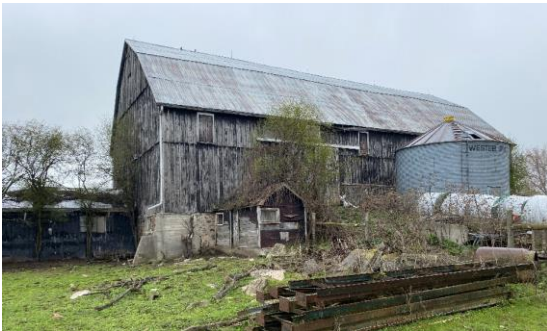
Photo 24: North elevation looking southwest
