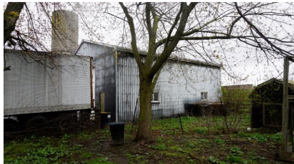
Photo 52: Storage outbuilding, west elevation looking southeast
