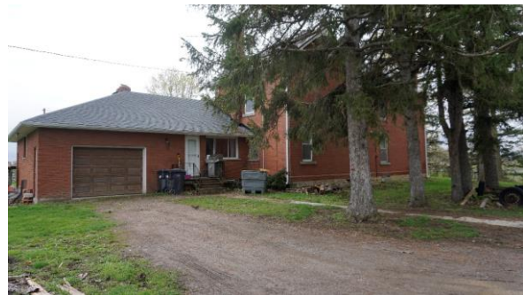
Photo 21: North elevation of addition looking southwest
