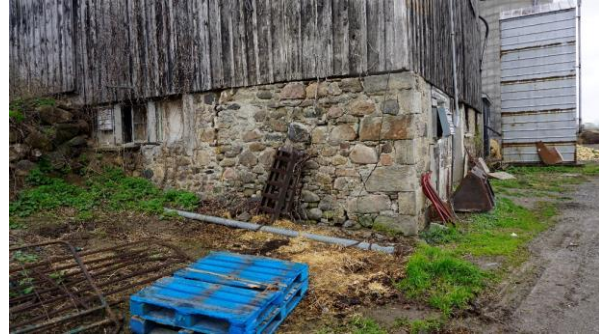
Photo 23: Detail of fieldstone foundation with cut stone corners
