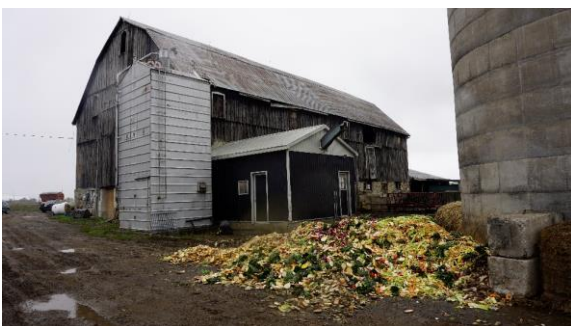
Photo 27: South elevation looking northeast
