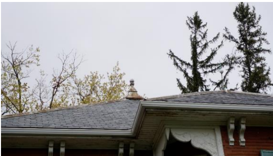
Photo 4: Metal roof finial looking north
