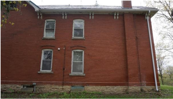
Photo 18: North elevation looking south
