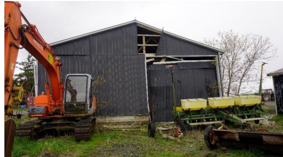
Photo 34: Driveshed east elevation looking northwest
