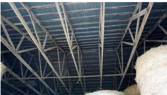
Photo 41: Driveshed interior, east portion
