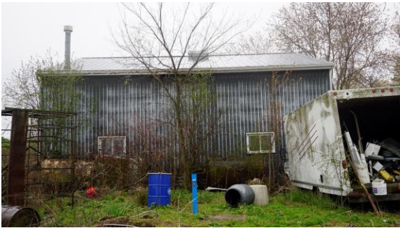
Photo 53: Storage outbuilding, east elevation looking west
