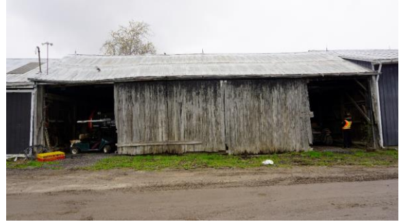
Photo 32: Driveshed south elevation, centre portion looking north
