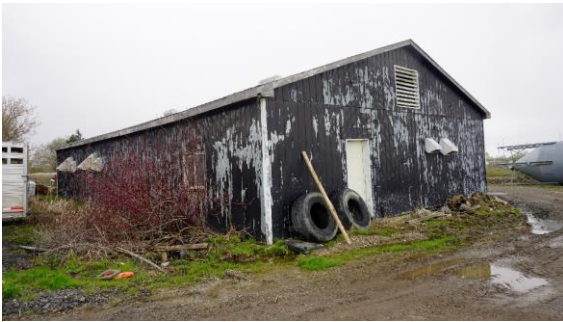
Photo 42: Storage driveshed, south and east elevations looking northwest
