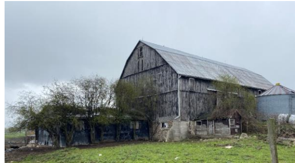
Photo 30: East elevation looking southwest
