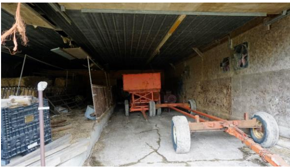
Photo 48: Storage driveshed, interior
