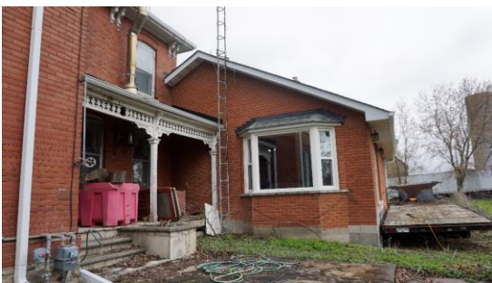
Photo 14: West elevation of addition looking northeast
