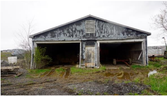
Photo 46: Storage driveshed, west elevation looking east
