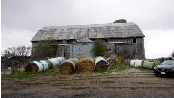
Photo 22: North elevation of the barn looking south
