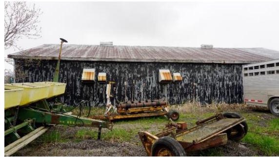
Photo 43: Storage driveshed, south elevation looking north
