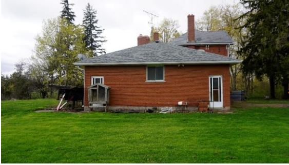
Photo 16: East elevation of addition looking west
