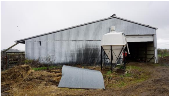
Photo 49: Cattle outbuilding west elevation looking east
