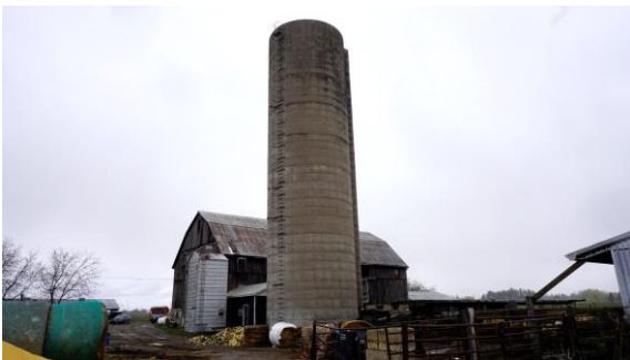
Photo 54: Silo looking northeast
