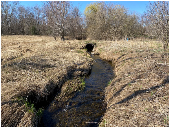
Photo 15: Conditions in Kilamanagh Creek facing upstream with old concrete pipe culvert in the channel and csp draining HDF-KCR-H1 on the north bank. Date: April 14 2023
