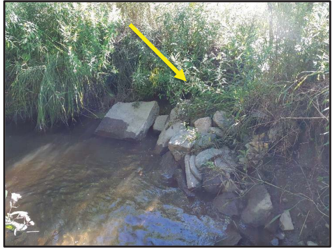
Photograph 10. (Photo Location 10) Downstream view of localized stone bank protection.
