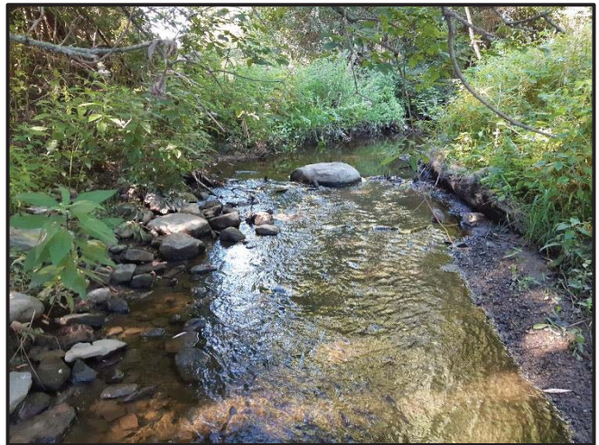
Photograph 4. (Photo Location 4) Upstream view of basal scour along channel bank.
