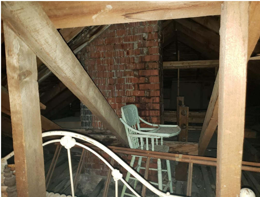
Plate 47: Brick chimney through attic (ASI 2021)
