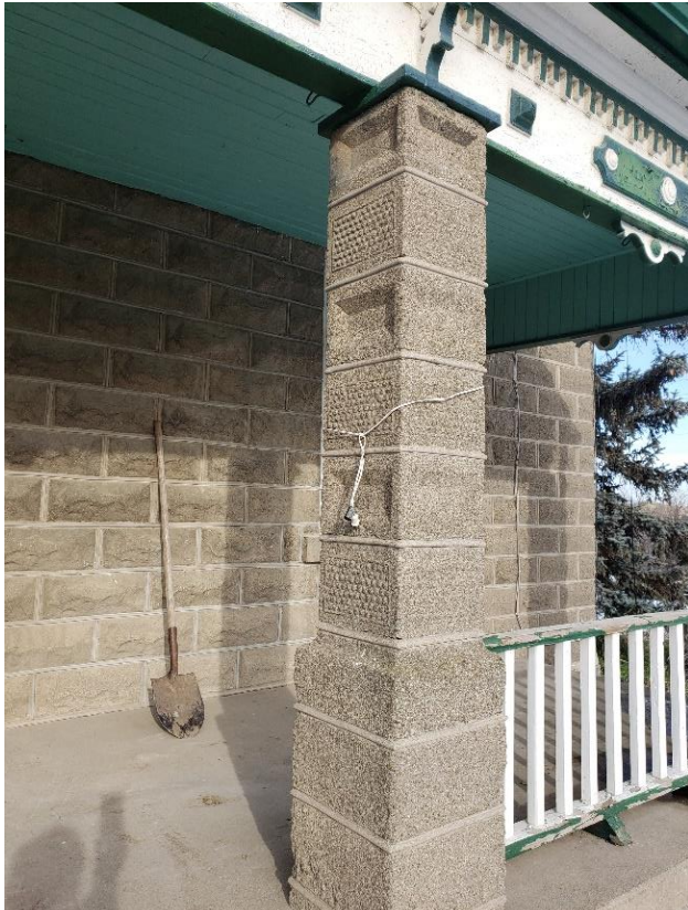
Plate 13: Concrete block column on front (south) elevation (ASI 2021)
