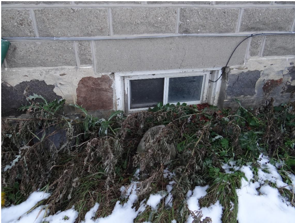
Plate 18: Basement window with concrete lintel and cut stone foundation (ASI 2021)
