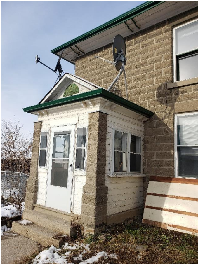
Plate 20: Secondary entrance, with wooden cladding (ASI 2021)
