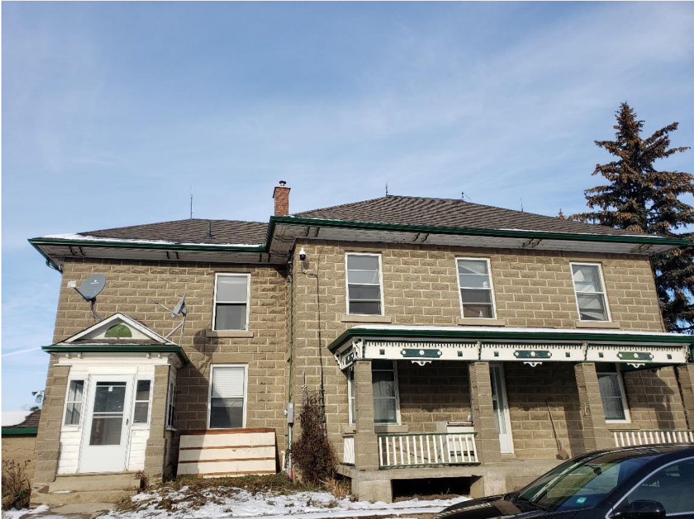
Plate 8: Southern elevation of 12434 Dixie Road (ASI 2021)
