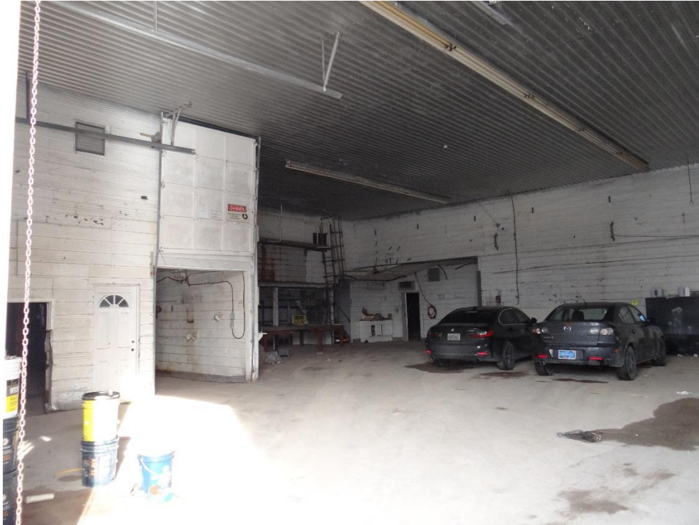
Plate 61: Interior of outbuilding No. 2 (ASI 2021)
