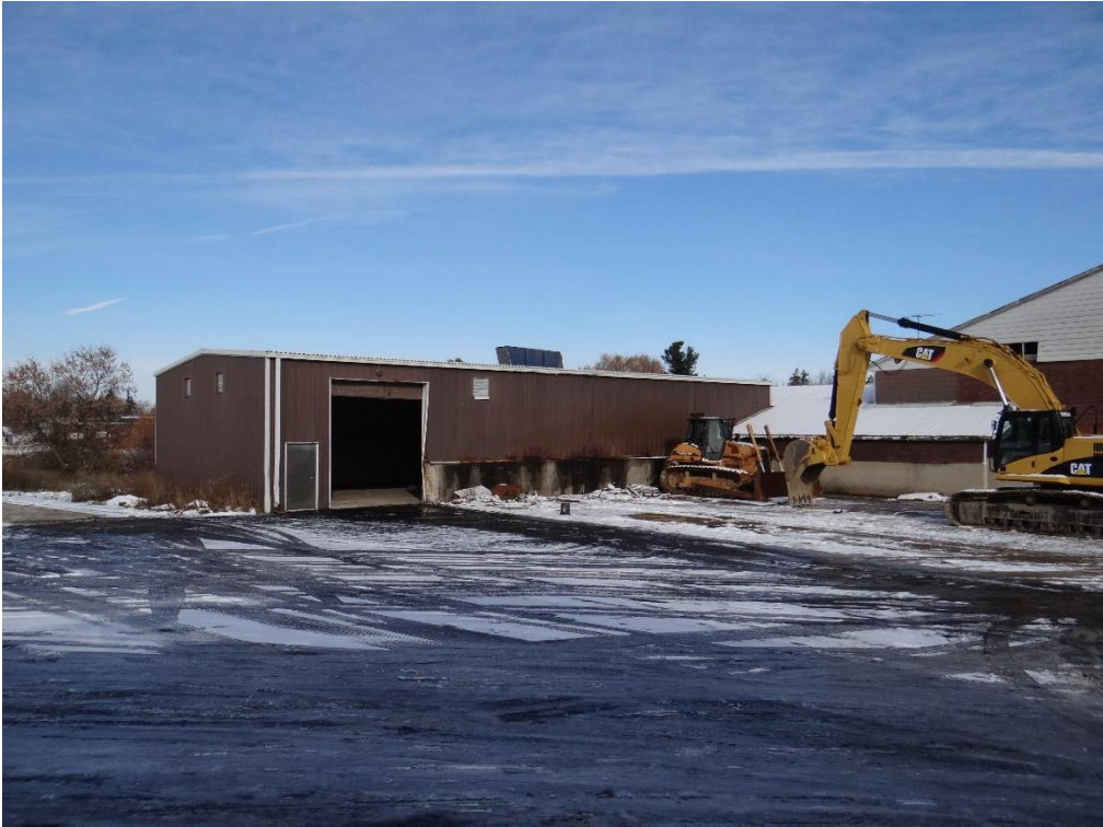
Plate 62: Exterior of outbuilding No. 3 (ASI 2021)
