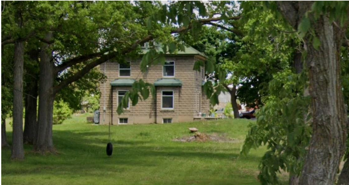
Plate 69: 12511 Winston Churchill Boulevard (Courtesy of Google Streetview 2021)
