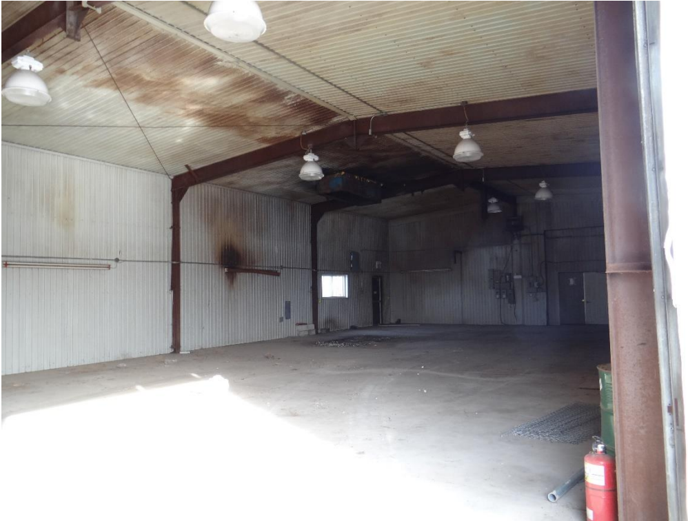
Plate 63: Interior of outbuilding No. 3 (ASI 2021)
