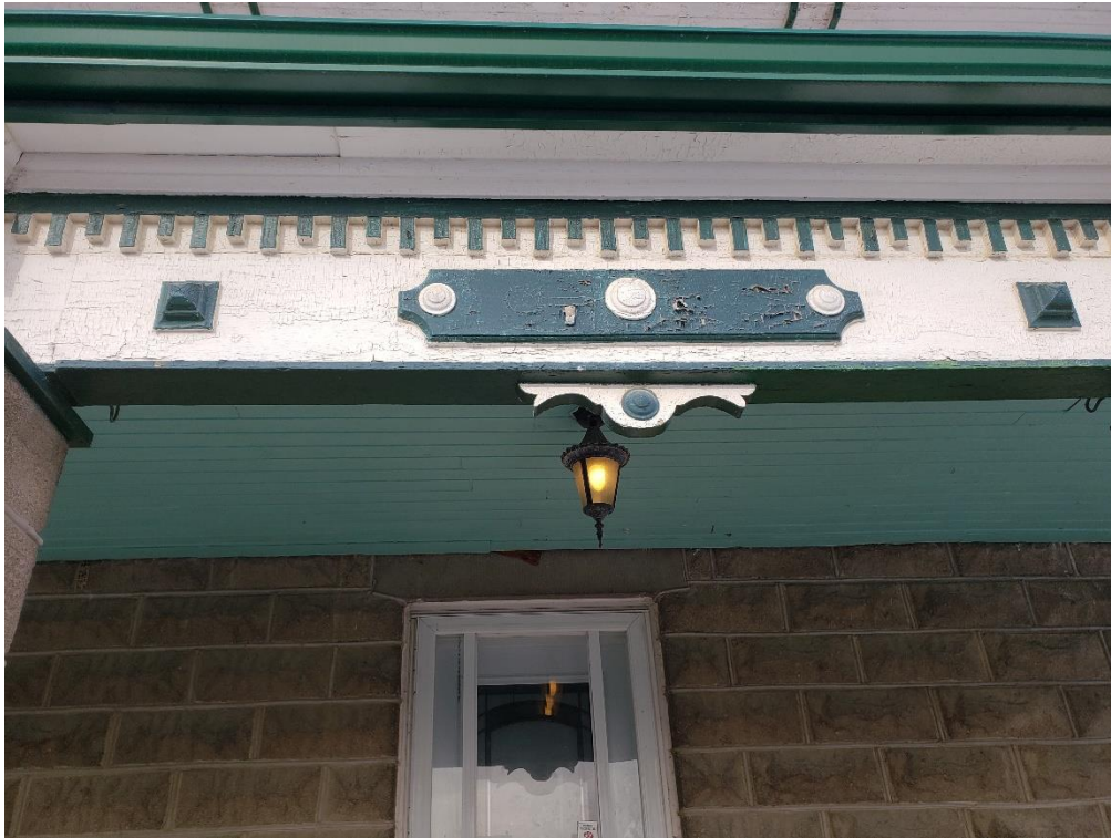
Plate 14: Painted wooden porch detail (ASI 2021)
