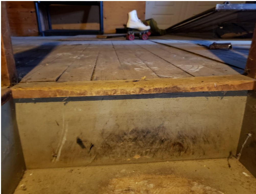
Plate 44: Wood flooring in attic (ASI 2021)
