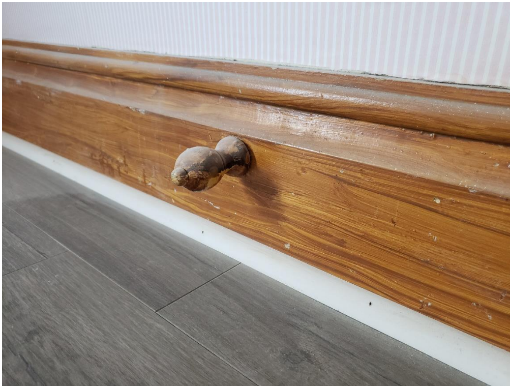
Plate 39: Door stopper mounted to original baseboard in second floor bedroom (ASI 2021)
