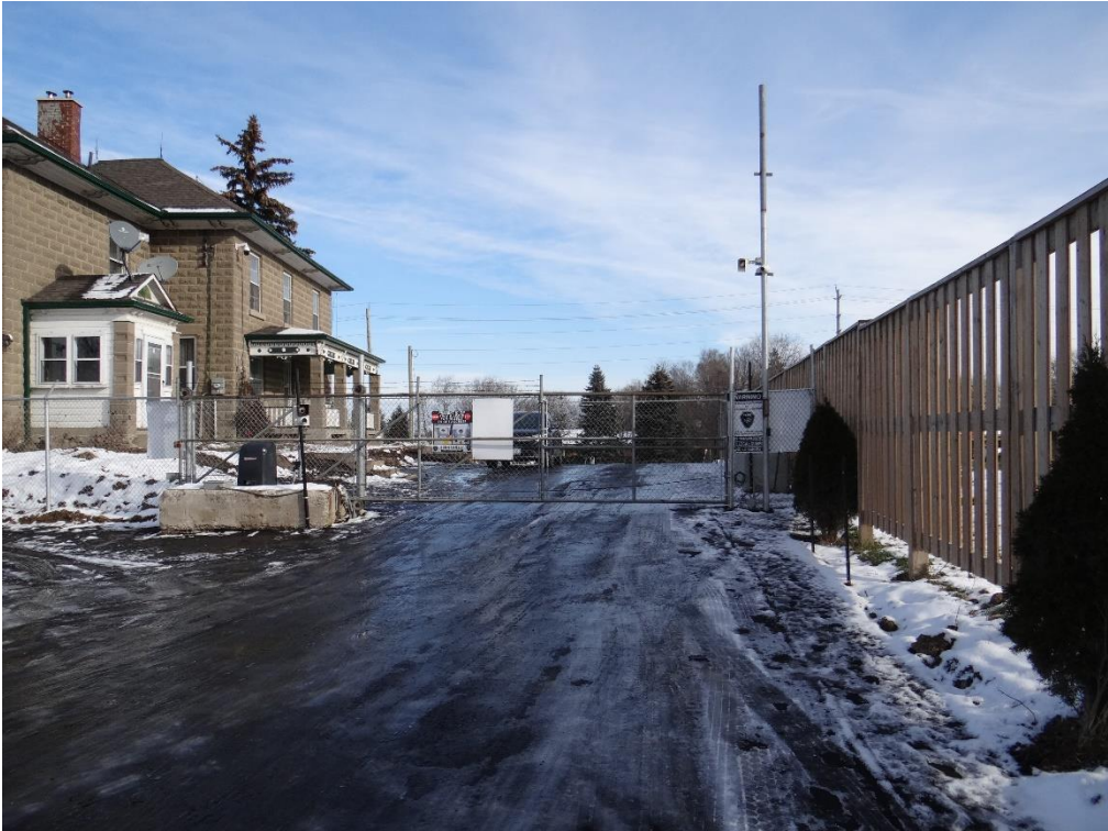
Plate 50: Driveway and access fence, looking east (ASI 2021)
