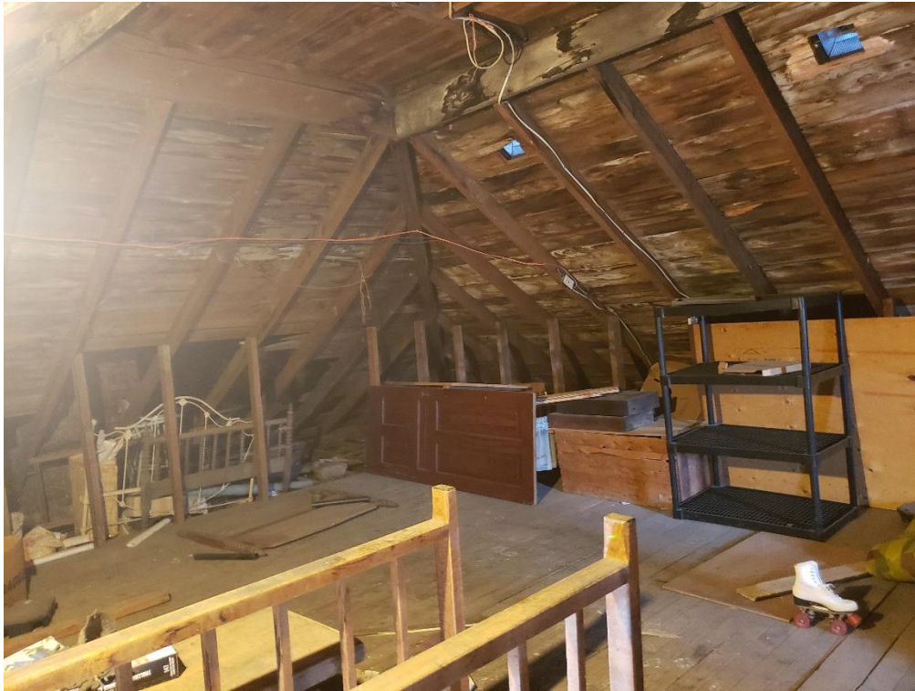
Plate 46: Wood beams supporting hipped roof in attic (ASI 2021)
