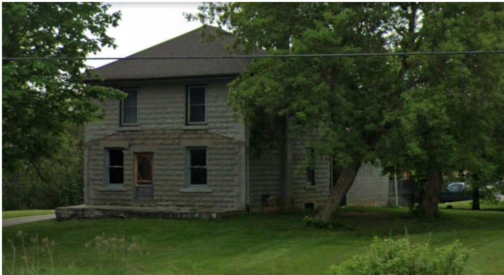
Plate 67: 15826 Regional Road 50 (Courtesy of Google Streetview 2021)
