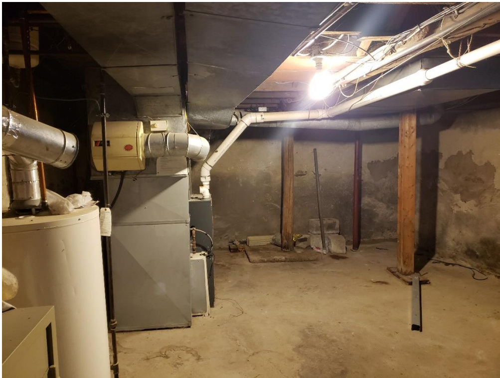
Plate 23: Furnace room in basement (ASI 2021)
