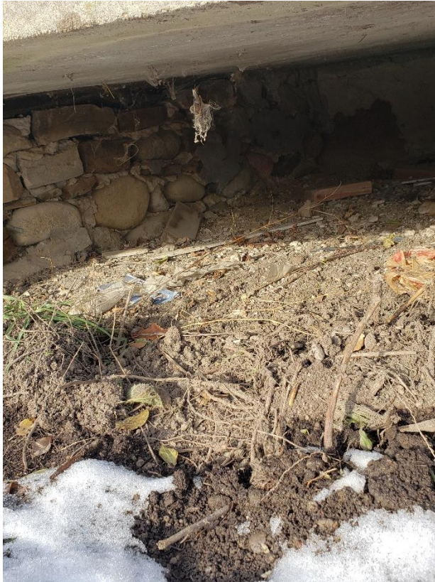
Plate 19: Field stone foundation under porch (ASI 2021)
