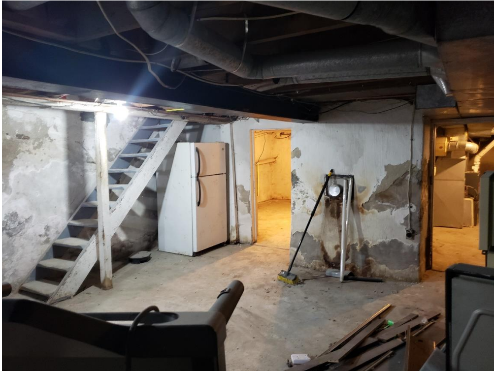
Plate 24: Staircase down to western-most storage room in basement (ASI 2021)
