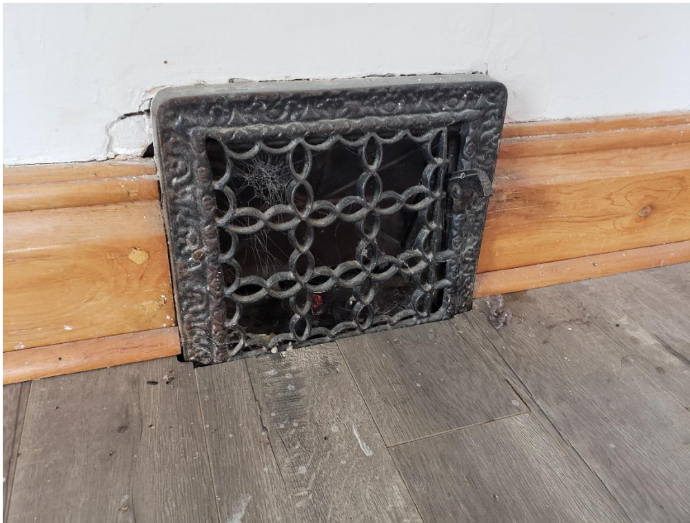
Plate 37: Air vent in second floor bedroom (ASI 2021)
