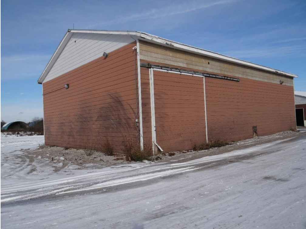
Plate 65: Exterior of outbuilding No. 5 (ASI 2021)
