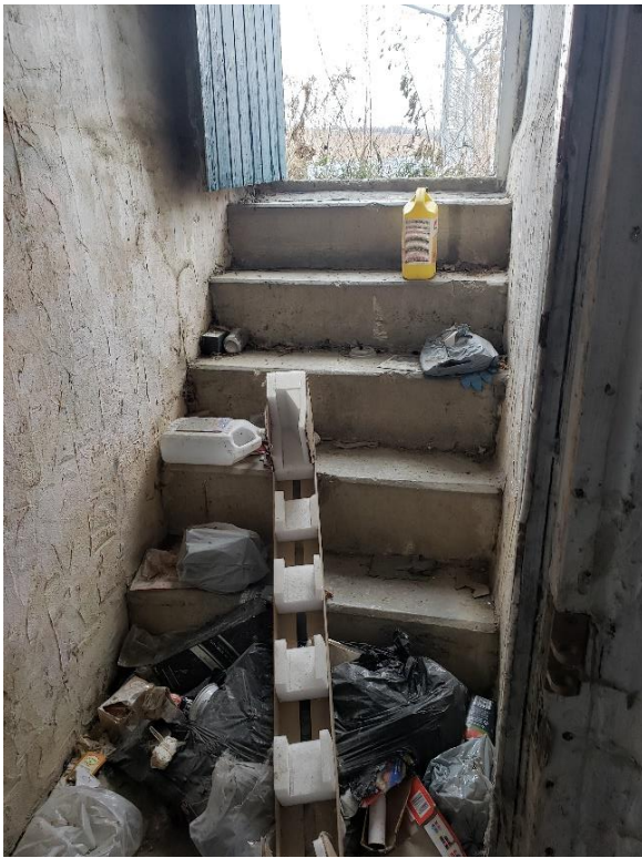
Plate 25: Staircase from basement to exterior (ASI 2021)
