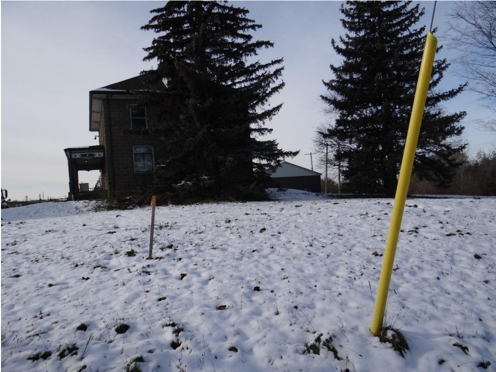
Plate 49: Residence sitting on a slight rise in land, looking west (ASI 2021)
