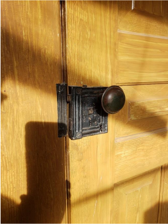
Plate 43: Doorknob and lock on second floor door to attic (ASI 2021)
