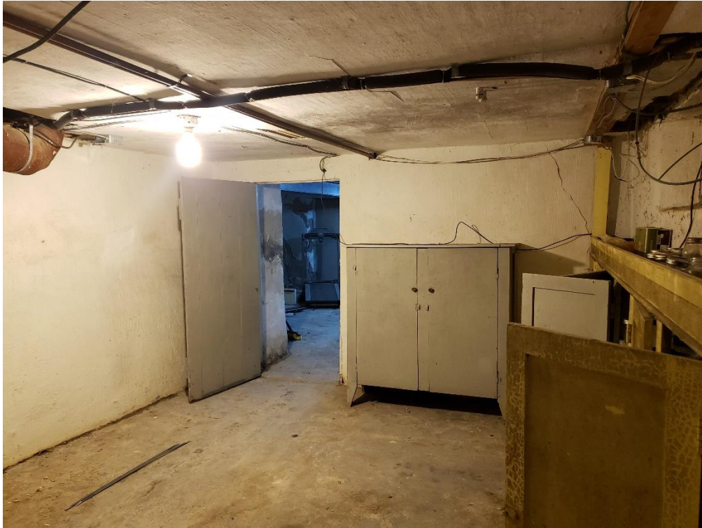
Plate 22: Large storage room in basement (ASI 2021)
