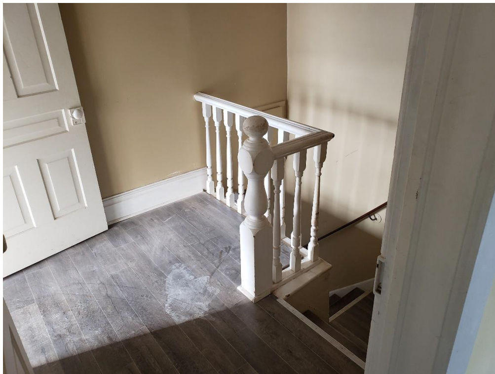
Plate 42: Second floor secondary stairway landing (ASI 2021)
