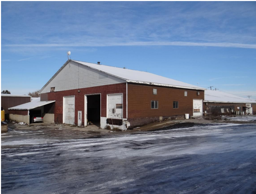
Plate 60: Exterior of outbuilding No. 2 (ASI 2021)
