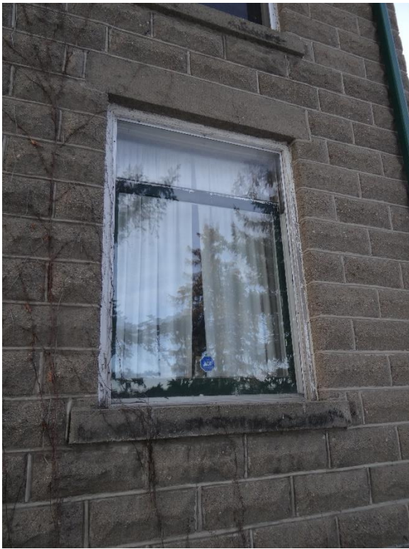
Plate 16: Window with concrete lintel and sill (ASI 2021)
