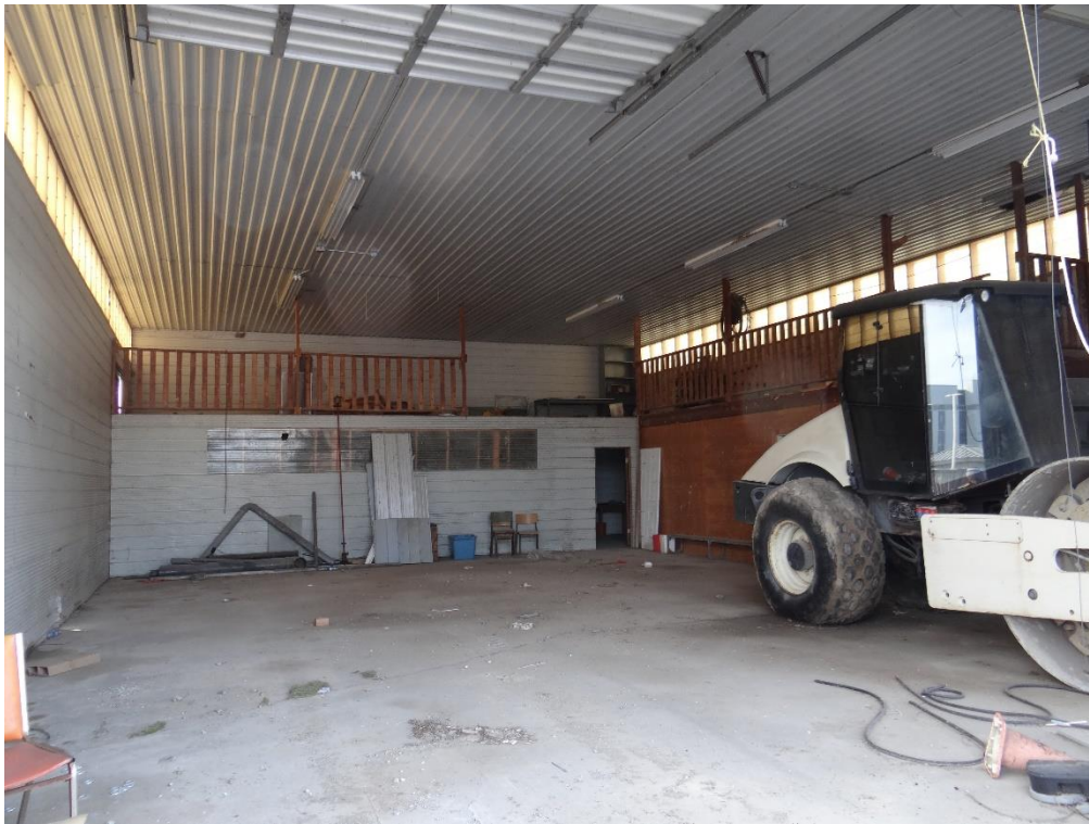
Plate 66: Interior of outbuilding No. 5 (ASI 2021)
