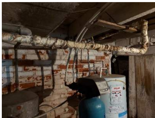
Photograph No. 2 Suspected ACM pipe insulation (Basement of Building A)
