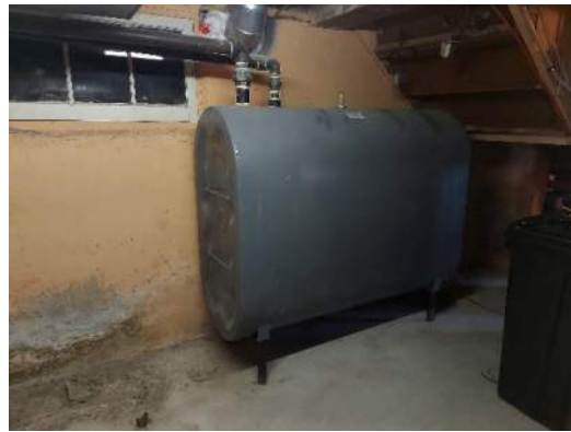
Photograph No. 10 View of the interior AST (Basement of Building B)
