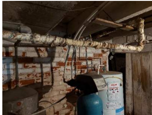
Photograph No. 2 Suspected ACM pipe insulation (Basement of Building A)
