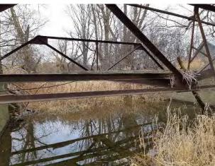
Photo 4 – An old crossing was noted within the property, which was in poor condition. The structure does not impede flow. Photo taken facing upstream.
