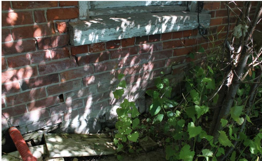
Figure 9: Base of Wall Deterioration
