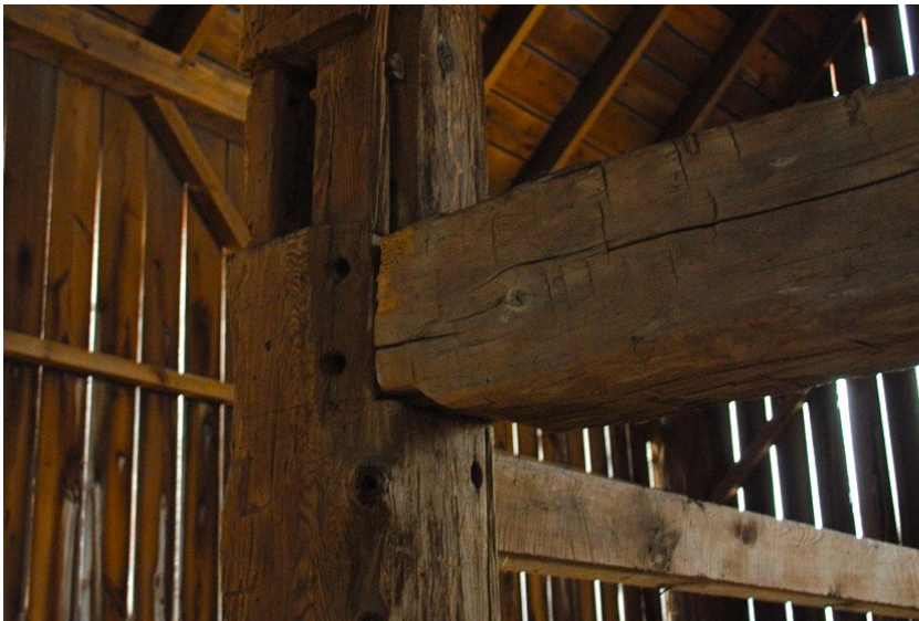
Figure 20: Detail of the hewn tie beam morticed and tenoned into a post with pegs.
