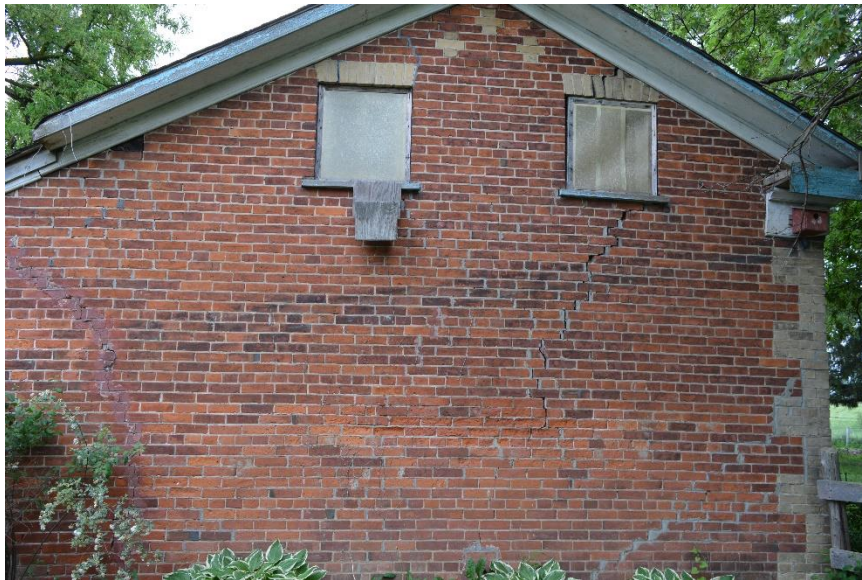
Figure 5: West Wall Damage
