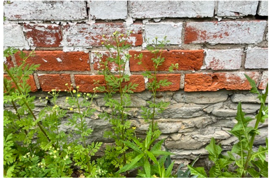
At the random rubble foundation, efflorescence is present.
