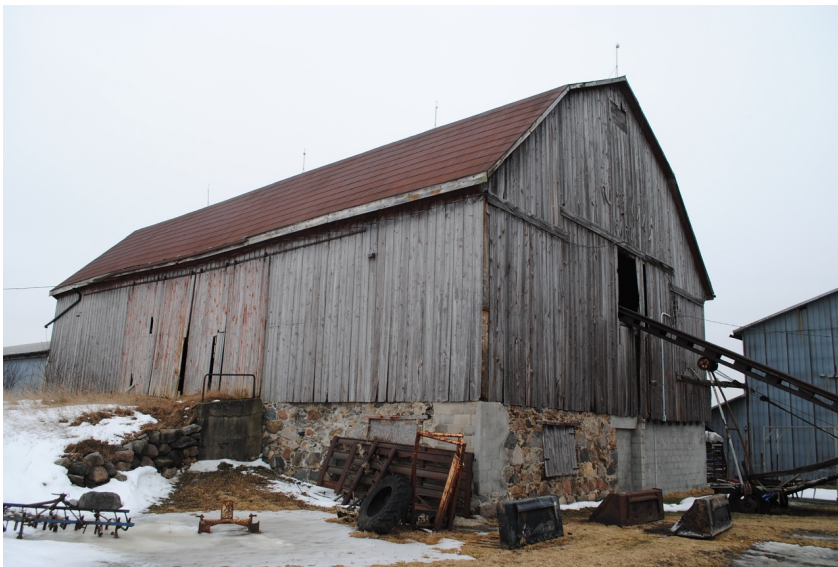
Figure 12: North wall of the main barn – the silo is located to the left. Note the foundation at the west, and north where blocks have been used for repairs to the stone. Boards are missing on the sliding wagon doors that are located at the mid-section of the barn on a rise of land. Foundations have been patched with a hard concrete surface -the concrete is typical of the post WWII era rather than the interwar period which would have had a higher lime content.
