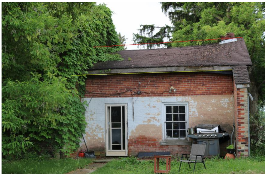
Figure 12: Sagging Roof
