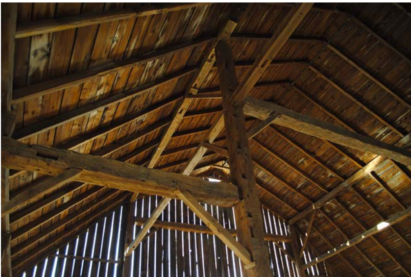
Figure 18: Detailed view of roof framing – east side showing roof planking, roof rafters, roof purlins, diagonal bracing, and horizontal members.
