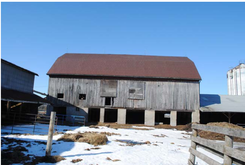
Figure 13: South wall of the main barn - the hay barn addition and silo are visible to the right. In this case, the forebay uses cinder blocks suggesting that the footprint and size of the barn was changed with renovations in the 20th century. The hay barn incorporates heavy framing timbers salvaged from an earlier structure so may have been constructed from framing members salvaged from an earlier barn on site.
