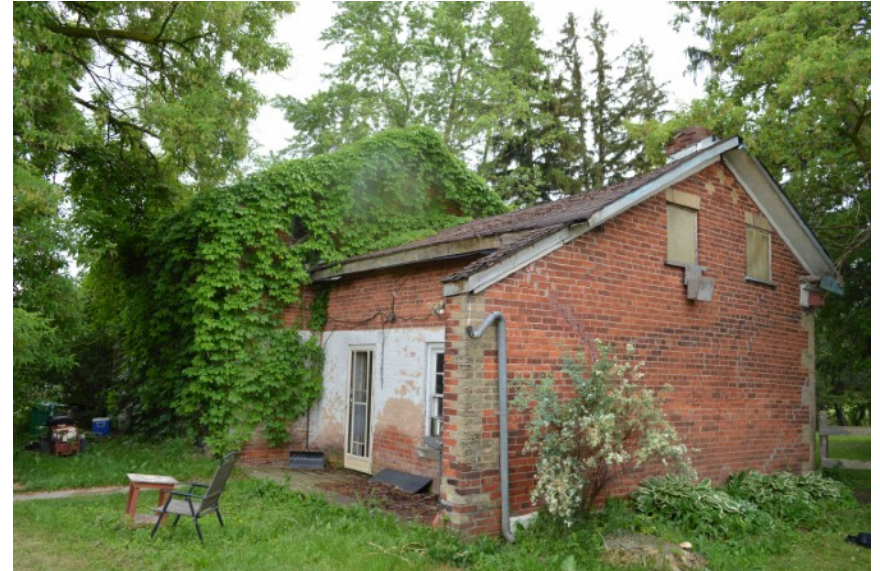
View of the east elevation, with the lower addition visible and the rear elevation of the main house obscured by vegetation. The top windows of the east elevation have been covered.
