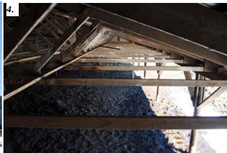
Figure 6: Interior view of newer 2x beams in the hay barn (Building #3) viewed from within the main barn.
