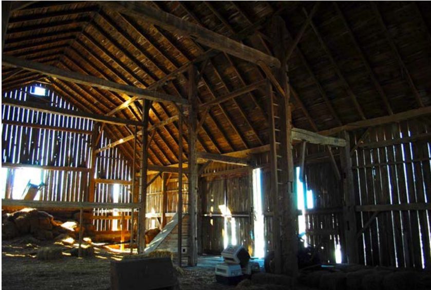
Figure 16: General interior view looking west from main entrance showing three bents, with ladder access along the post.
