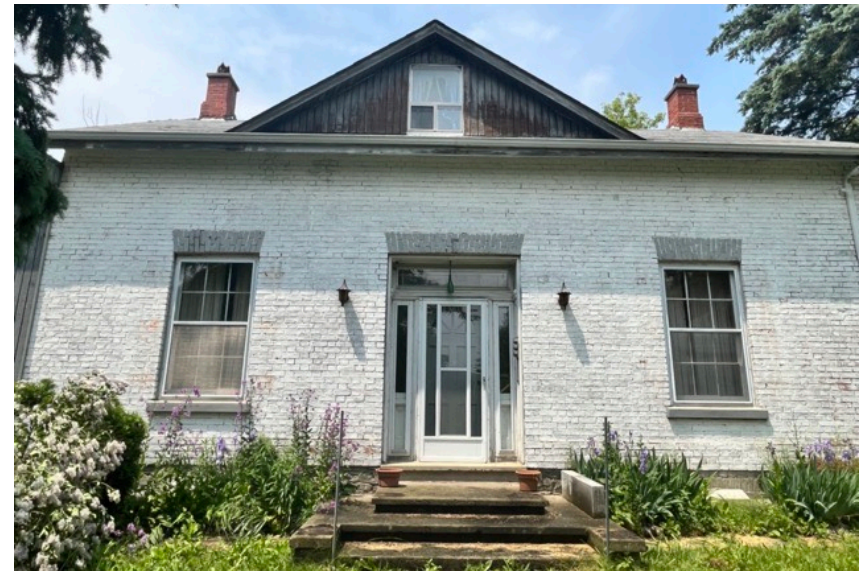
Non-original storm door with raised entrance. Side lights, transom flanked by 6-over-6 windows in good condition.
