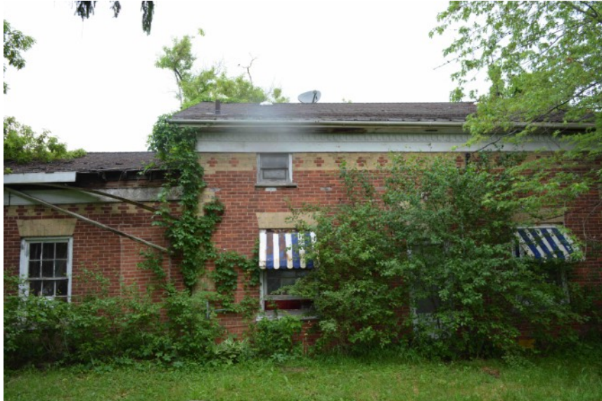
View of the principle (west) elevation of 12245 Torbram Road with the main house located to the right, with a central opening and a pair of six-over-six sash windows on either side. The frieze beneath the roof cornice is visible here, and a dentil band above.
