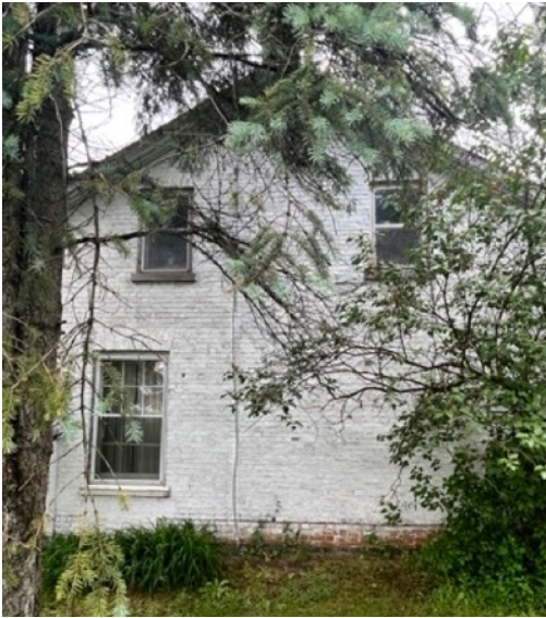
A view from the east elevation with randomly arranged windows. Evidence of potential ingress water at foundation is present given loss of white-wash.
