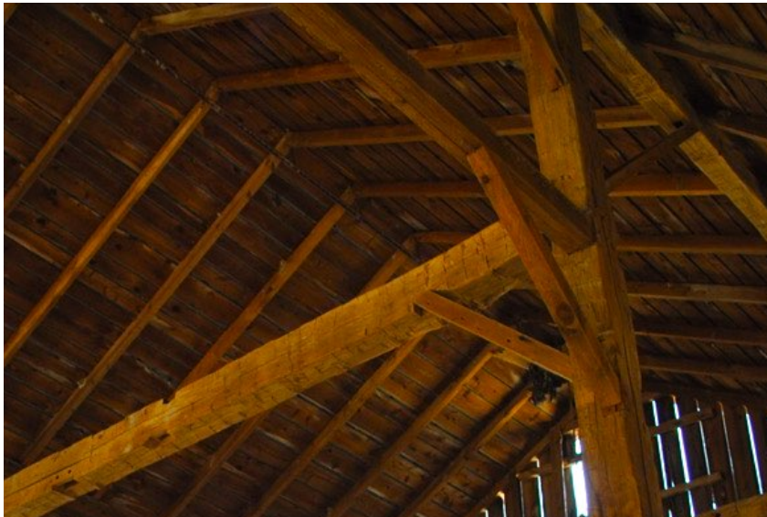
Figure 14: Detailed view of roof framing – north end at west side showing roof planking, roof rafters, roof purlins, diagonal bracing, and horizontal members.
