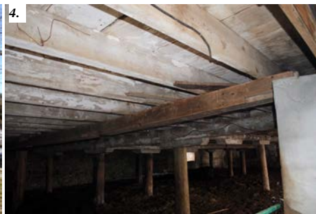
Figure 9: Interior view of the hay barn (Building #3) showing a mix of new timbers, and older hewn beams. Foundation is a combination of cinder block and wood construction.
