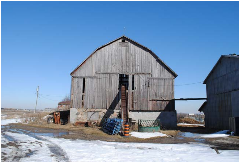
Figure 11: West end of the barn showing gambrel roof. It is likely that materials were salvaged from an earlier barn with the majority of the gambrel roof barn constructed sometime between the 1920's and 1970s.
