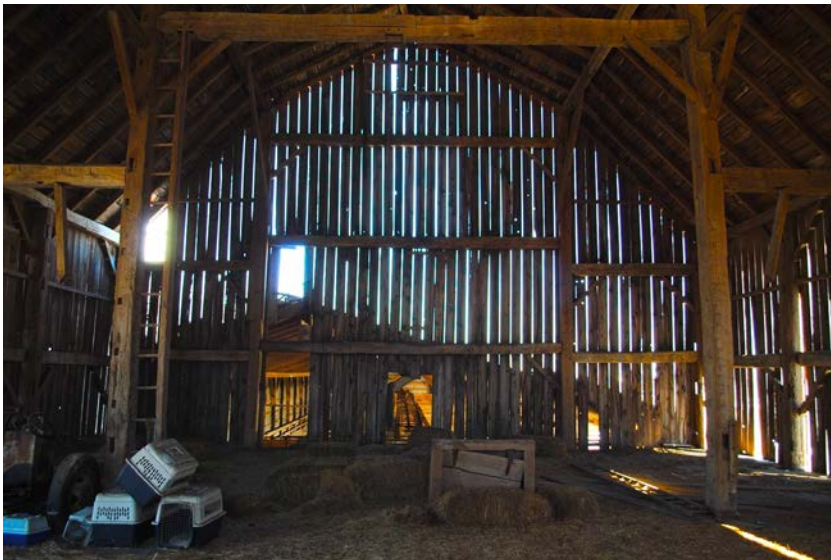
Figure 21: General interior view looking west from main threshing floor in the centre. Note the left and right tie beams have displaced braces.
