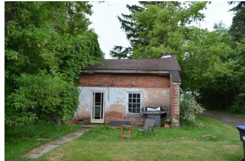
12245 Torbram Road, 2021 (GBCA). East Elevation (rear), showing current entrance to house with a brick buttress extending from the elevation, and structural deflection noticeable at gable ridge.
