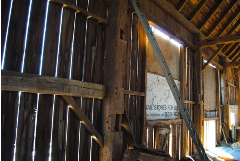
Figure 19: View of south wall, showing lack of significant bracing to the wall structure and empty mortises along the bent. The gaps between the planks provides considerable relief from wind loads.
