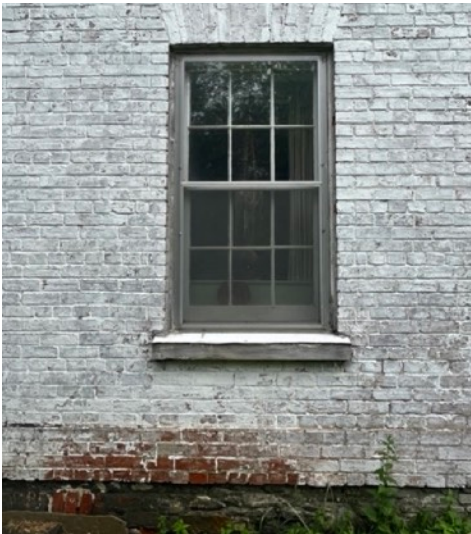
A view of the 6-over-6 ground floor windows. Evidence of potential ingress water at foundation is present given loss of white-wash.
