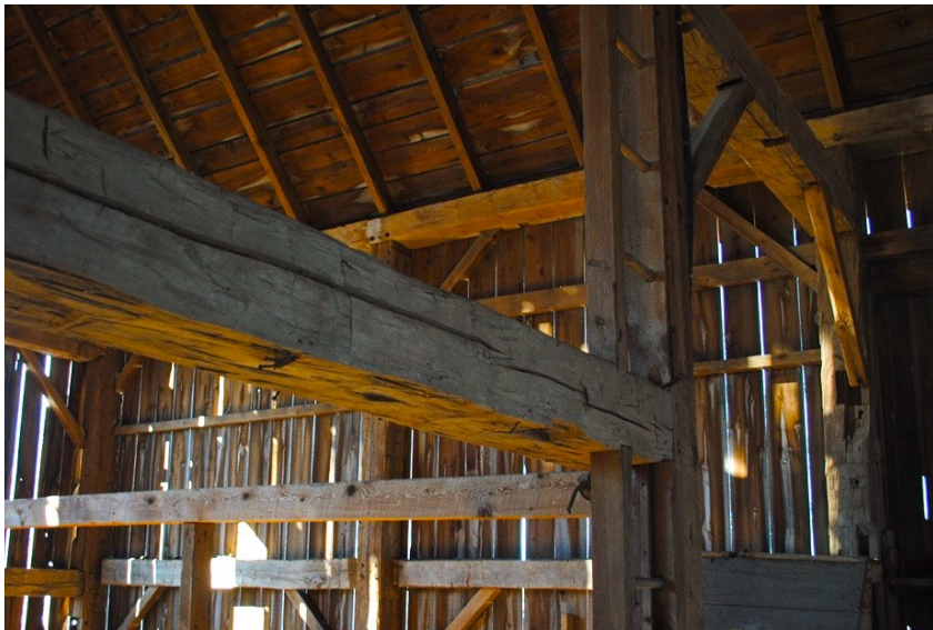
Figure 15: Detailed view of tie beam showing splitting that has not been restrained with iron strapping. Note the empty mortices indicating that this and several other elements have been re-assembled.
