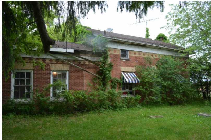
12245 Torbram Road, 2021 (GBCA). West Elevation. Top left window added at a later date. The central door opening is inaccessible, and side window of the lower addition is closed in.
