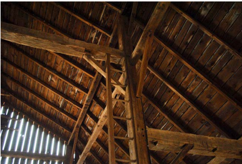
Figure 17: Straining beam shows evidence of double bracing due to empty mortise. These would have originally carried a double diagonal brace.
