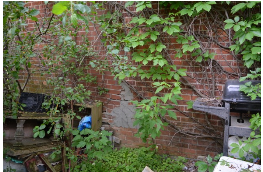
Parging applied to the masonry on the east elevation next to open joints. Ingress water damage and deterioration is likely present in these areas.
