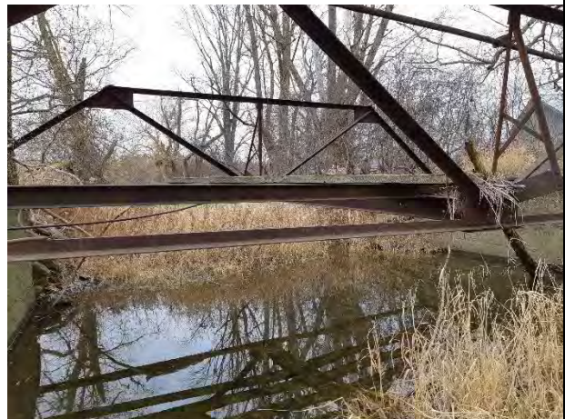
Photo 4 – An old crossing was noted within the property, which was in poor condition. The structure does not impede flow. Photo taken facing upstream.
