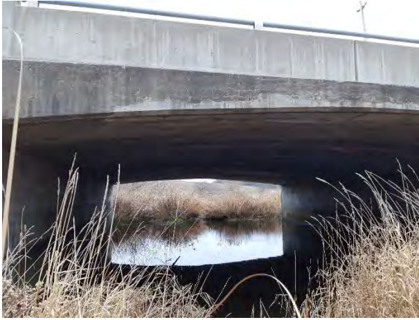
Photo 1 – Downstream view of Salt Creek, under the Airport Road crossing.
