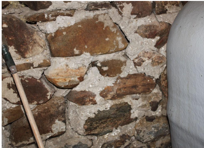
Figure 2: Typical Condition of Stone Foundation Wall
