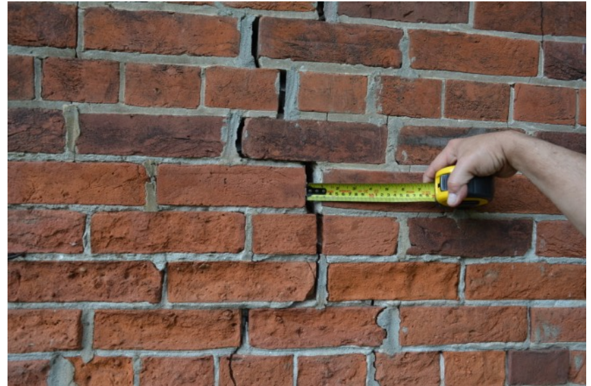
Numerous instances of pronounced step cracks ( \pm 1" and up to 2" or more) along the north elevation, along with other localized cracks in other portions of the east and west walls
