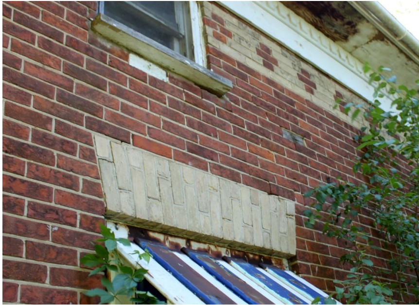
Figure 10: Wood Inserts in South Facade
