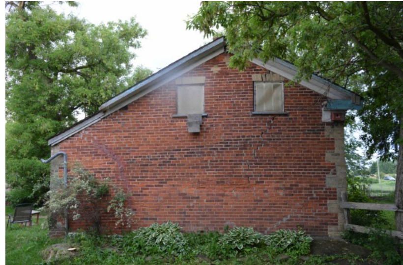
12245 Torbram Road, 2021 (GBCA). North Elevation. Blank wall with closed window openings and buttress to the left. Open joints in the masonry are noticeable from a distance. The buff-brick quoins are clearly visible on this elevation.
