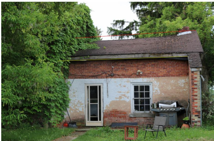
Figure 12: Sagging Roof
