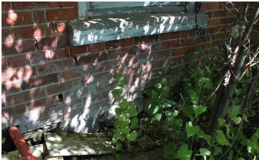
Figure 9: Base of Wall Deterioration
