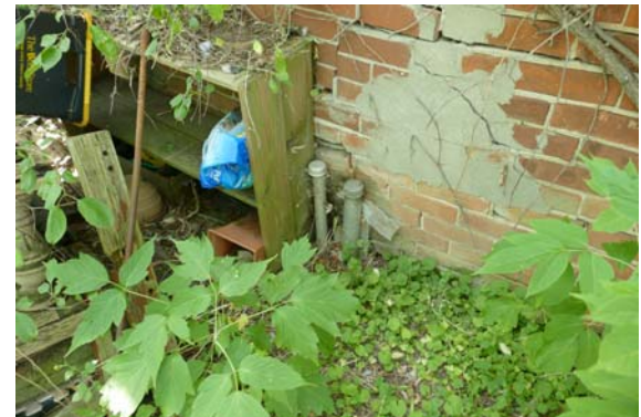
P18 - Fill and vent pipes at 12245 Torbram Road, located close to the northeast corner of the house
