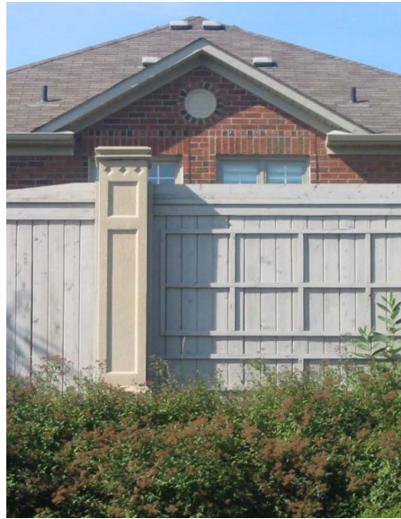
Figure 2.2e - Image example of wood acoustical fence with precast columns
