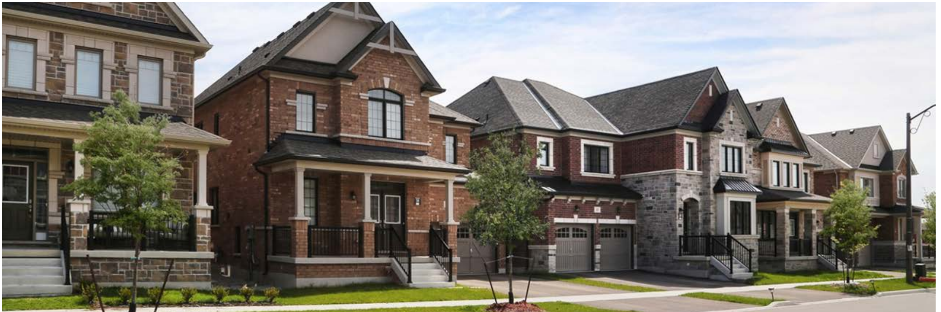
Figure 3.1a - Variety in architectural elevation design will help prevent streetscape monotony and promote a pedestrian-friendly environment
