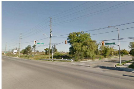
Figure 1.1c - View from Hurontario Street looking north
