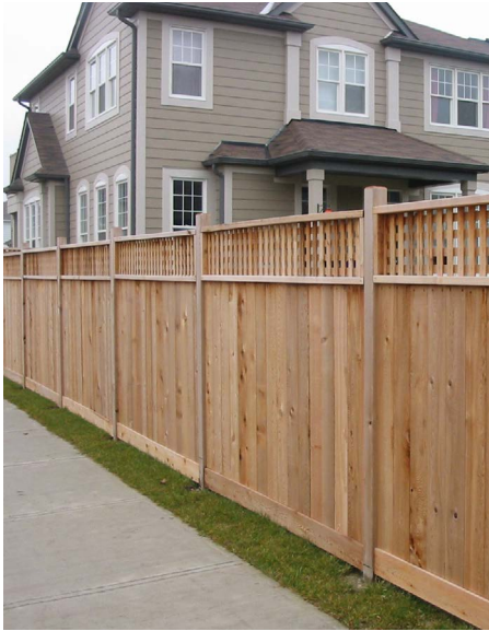
Figure 2.2d - Image example of wood privacy fence
