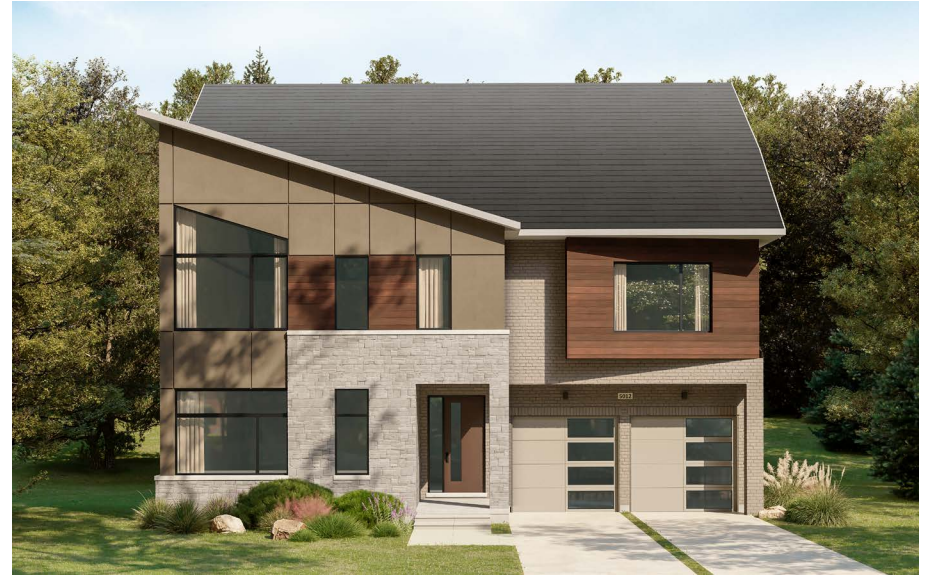
Figure 3.3d - A larger proportion of openings to solid wall should be integrated into elevations with prominent public views, such as corner units (Caivan OpenPlan™ 50' single detached lot)
