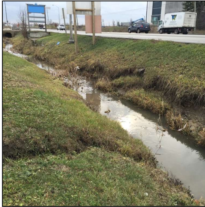
Photograph 1. Channel along Regional Road 50 showing slumping of the slopes and erosion gullies
