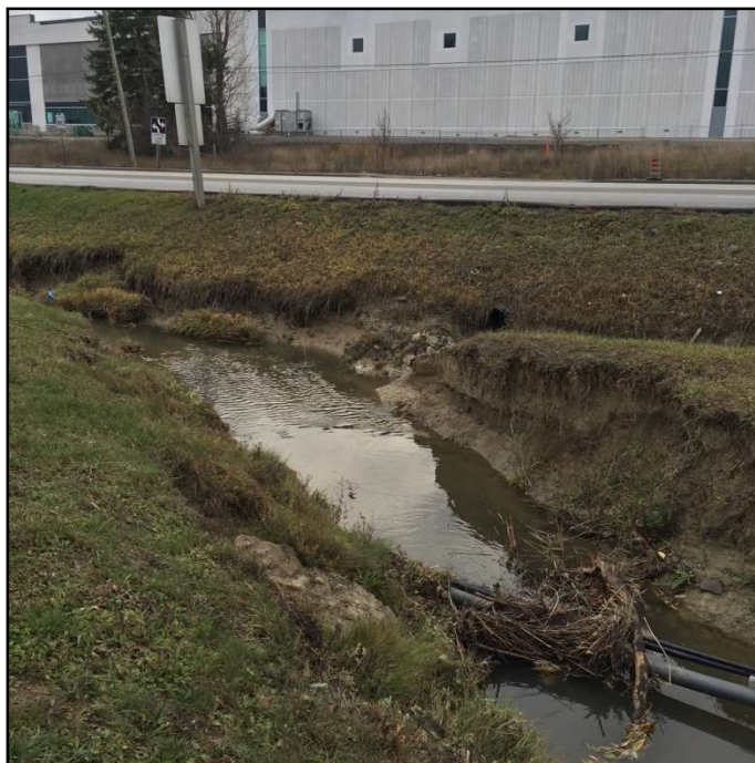
Photograph 4. Exposed service cables/pipes at the tributary as it joins the drainage ditch along Regional Road 50
