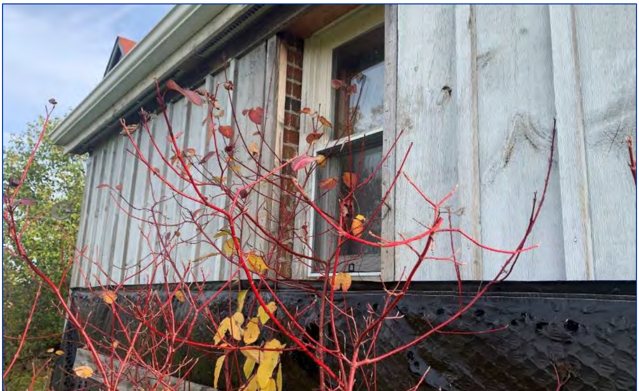
Photo 8: View of the board and batten siding with the brick underneath
