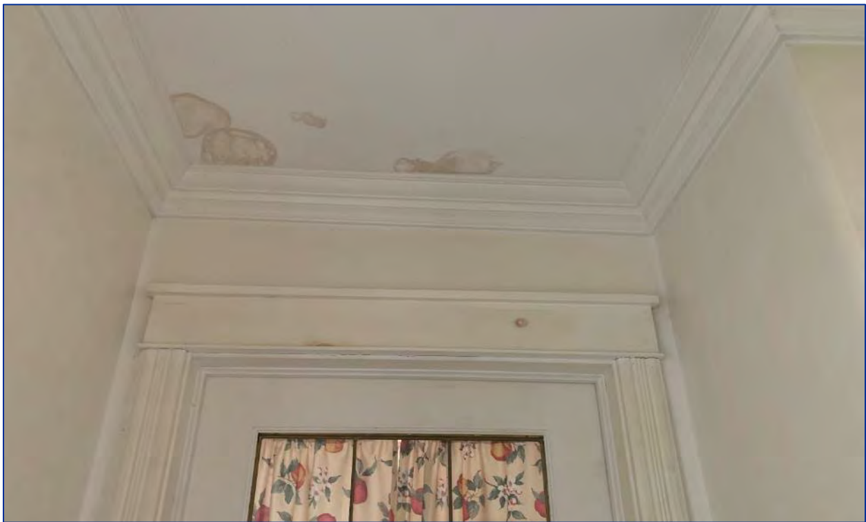
Photo 19: View of the residence's details, crown moulding and door casing
