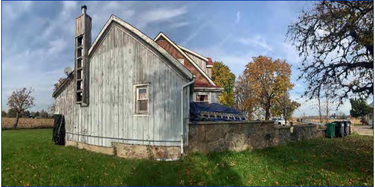
Photo 3: View of the west elevation of the residence
