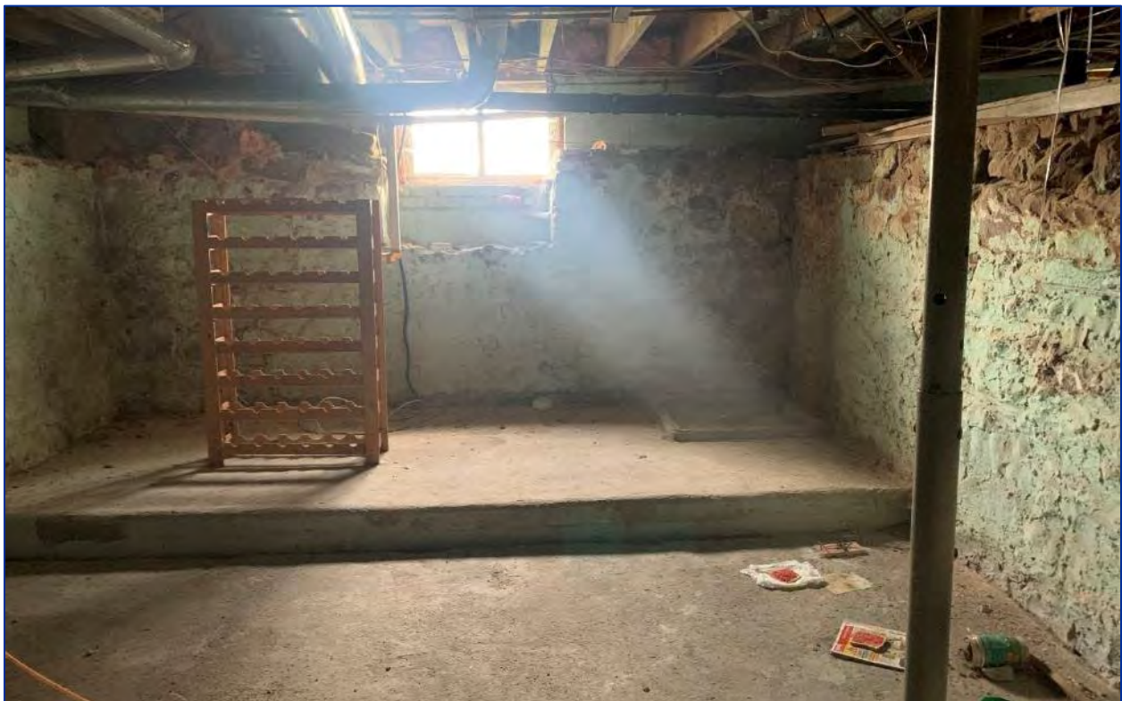
Photo 23: View of the basement detail
