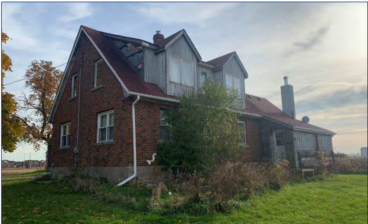
Photo 6: View of the northeast elevation of the residence
