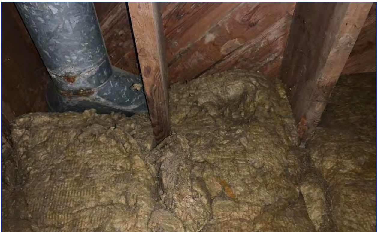
Photo 25: View of modern insulation and wooden flooring of residence
