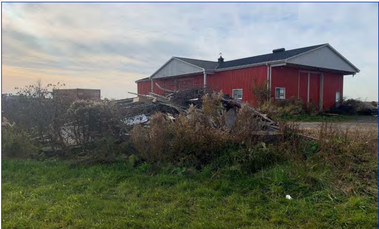
Photo 13: View north of southeast elevation of the barn
