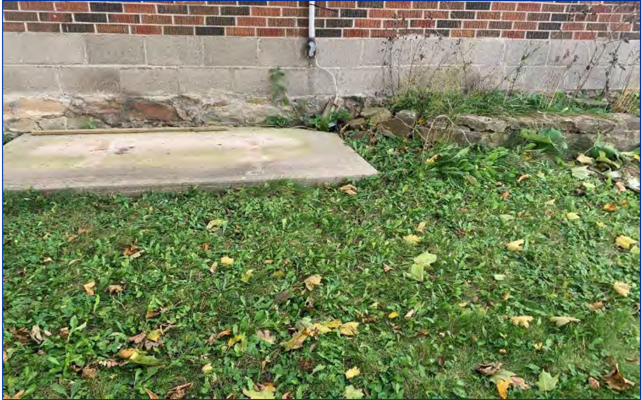
Photo 10: Detailed view of the foundation of the residence
