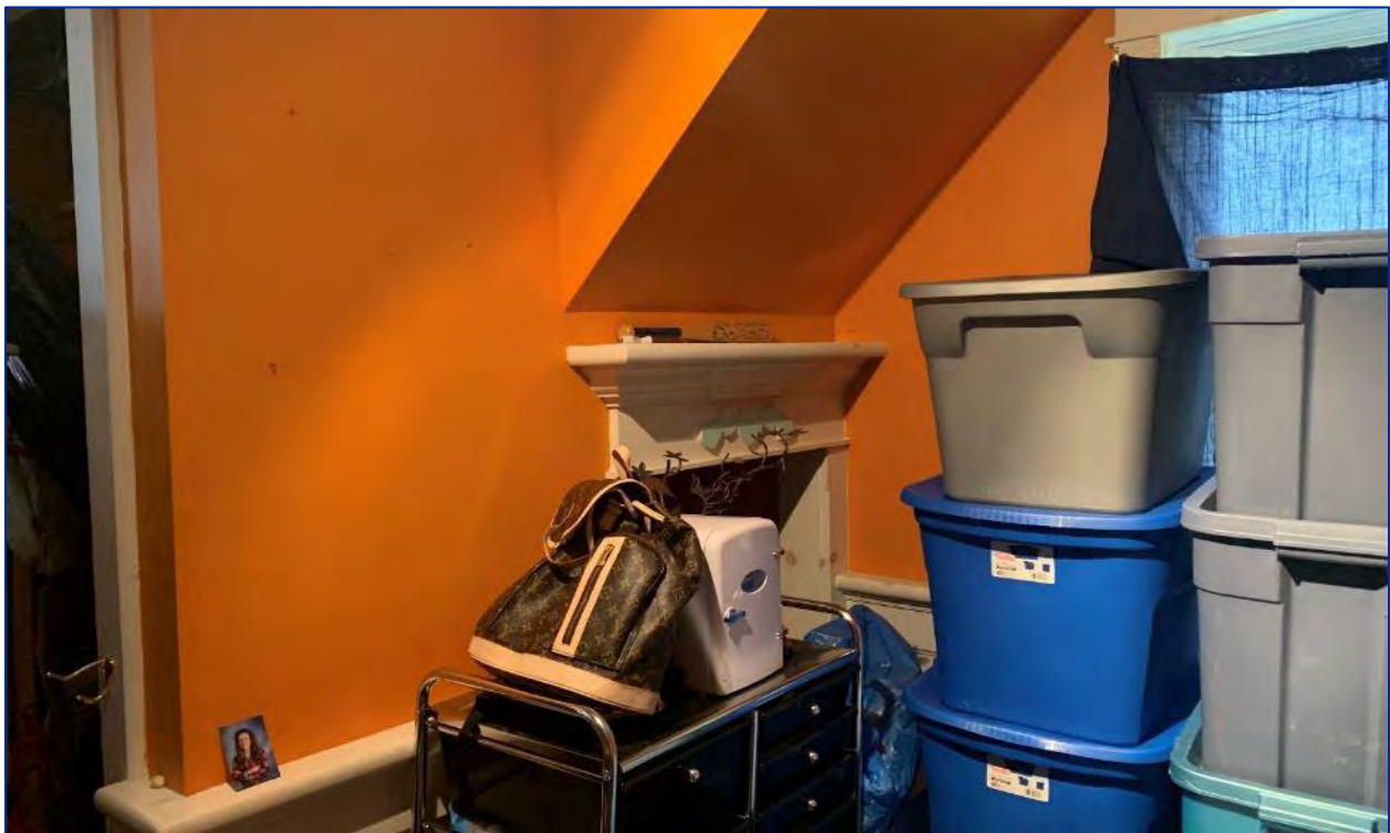
Photo 21: View of the details of a room and a former fireplace
