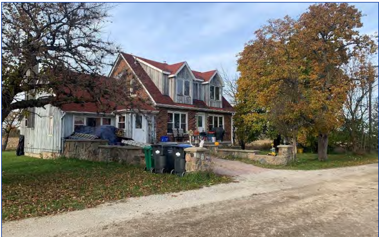
Photo 2: View of the southwest elevation of the residence
