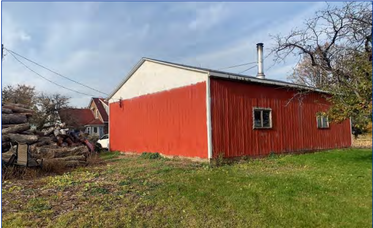
Photo 15: View north of southwest elevation of the garage
