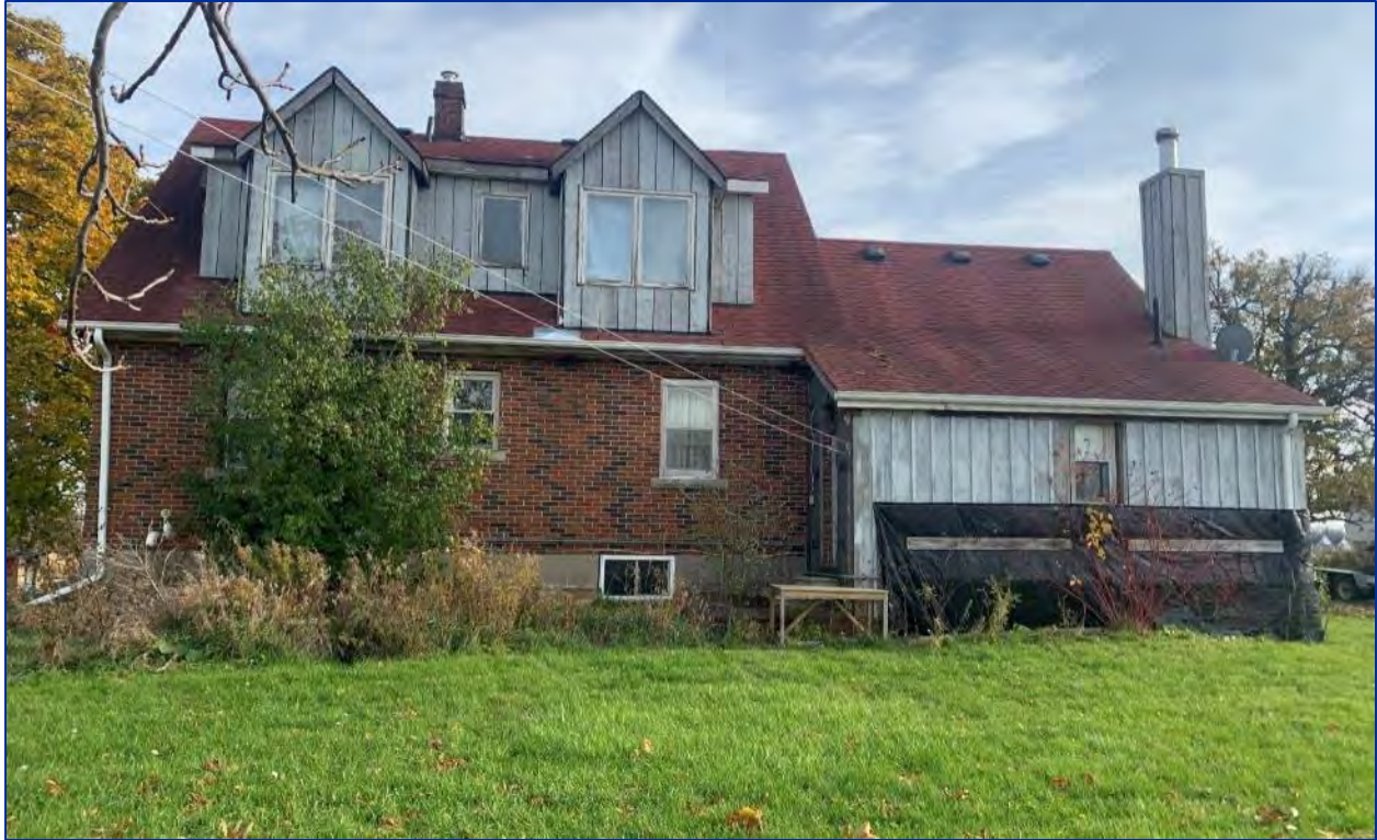
Photo 5: View of the north elevation of the residence
