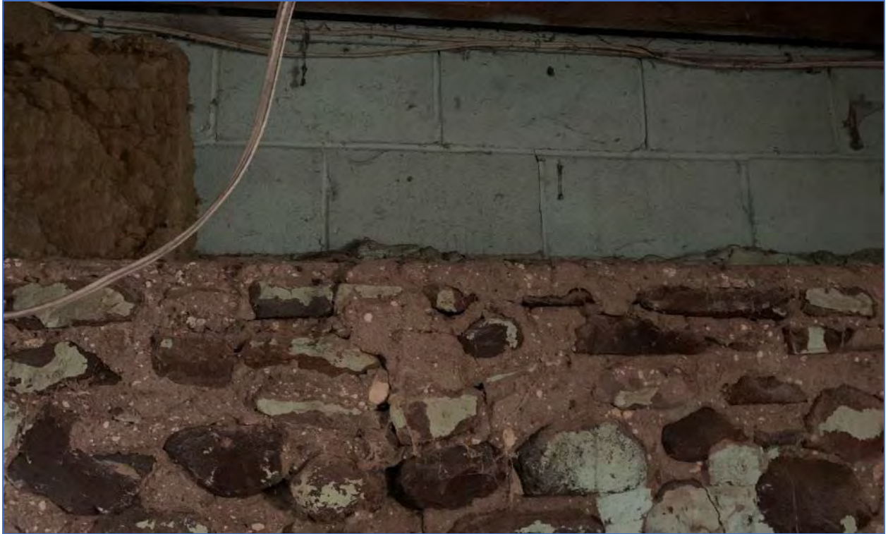
Photo 24: View of the fieldstone and concrete foundation of the residence
