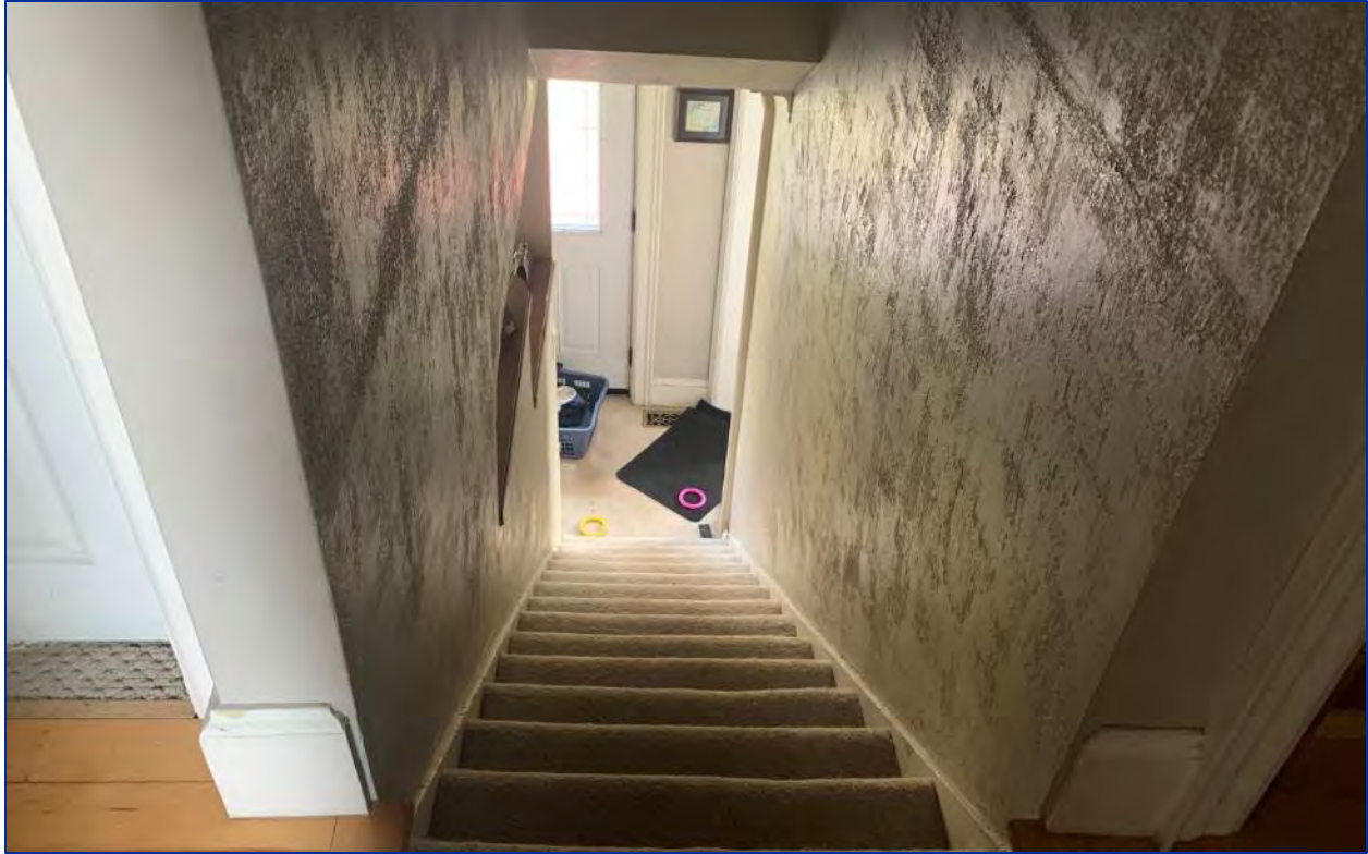
Photo 20: View of the staircase from the upper level
