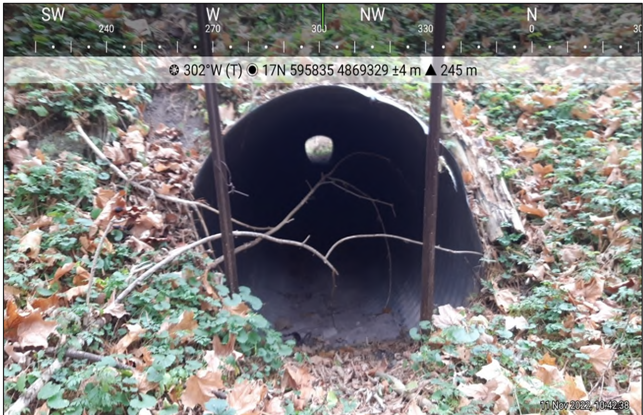
Figure 5: Culvert crossing of the Hunsden Sideroad, looking downstream from the Subject Lands, into the culvert inlet.
