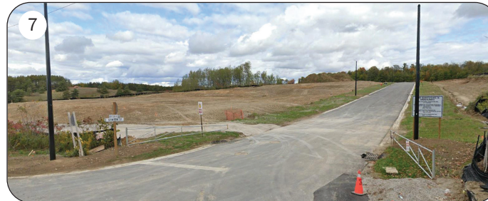
Intersection of Stinson St. and Mt. Pleasant Rd. (looking east)
