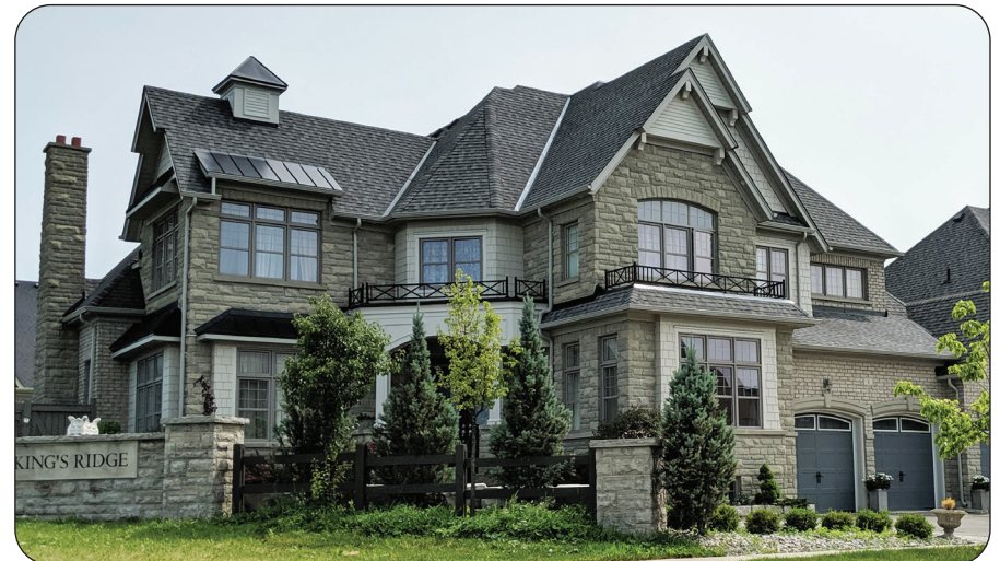
Corner or Gateway dwellings should respond to both street frontages in an equal manner
