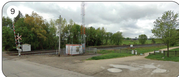
View of railway crossing and Caledon Trailway Path connection from Mt. Pleasant Rd.
