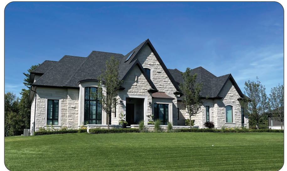
Positive relationships between built form and public spaces shall be maintained throughout the proposed development
