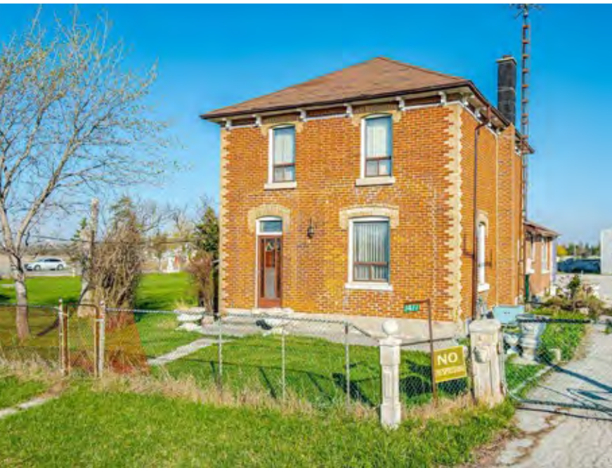
Streetview of the 19th century, square, two storey red brick residence at 7477 King Street, in the Italianate style, characterized by yellow brick detailing, hip roof and banding beneath the eaves.
