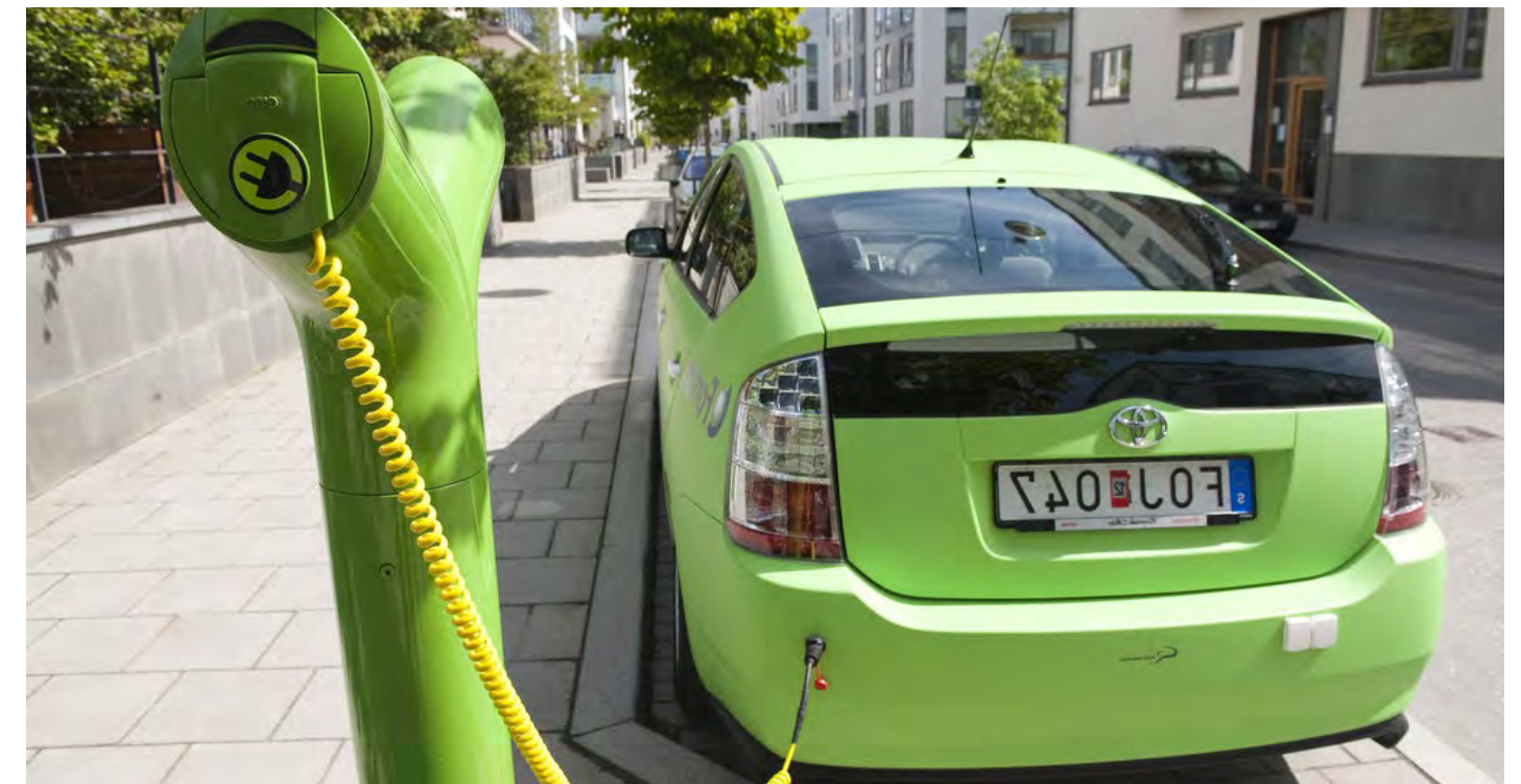
Electrical Vehicle Charging
