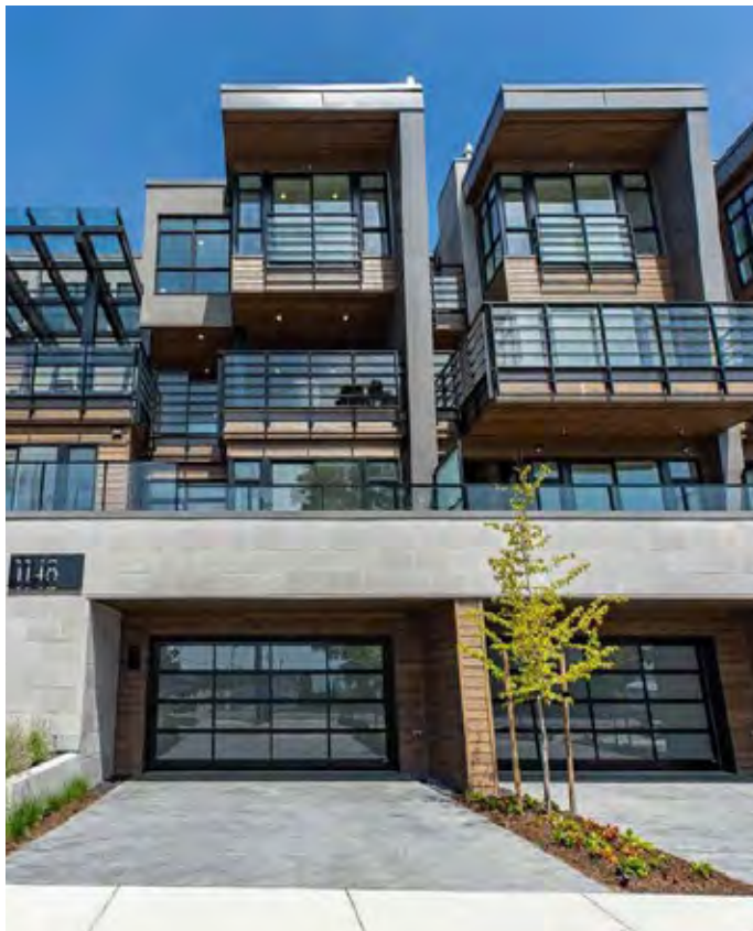
Habitable and/or amenity space above an attached/detached rear lane garage may be considered to animate the lane.
