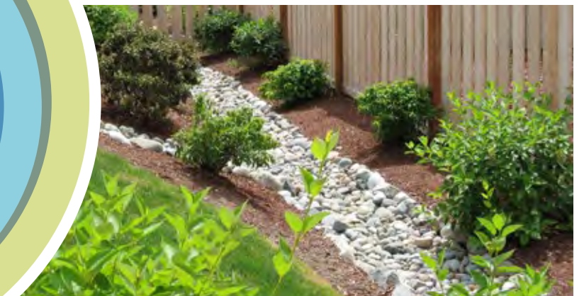
Lot Level Stormwater Retention
