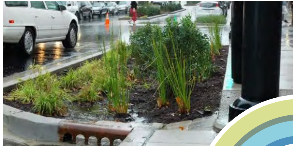
Street Level Stormwater Retention
