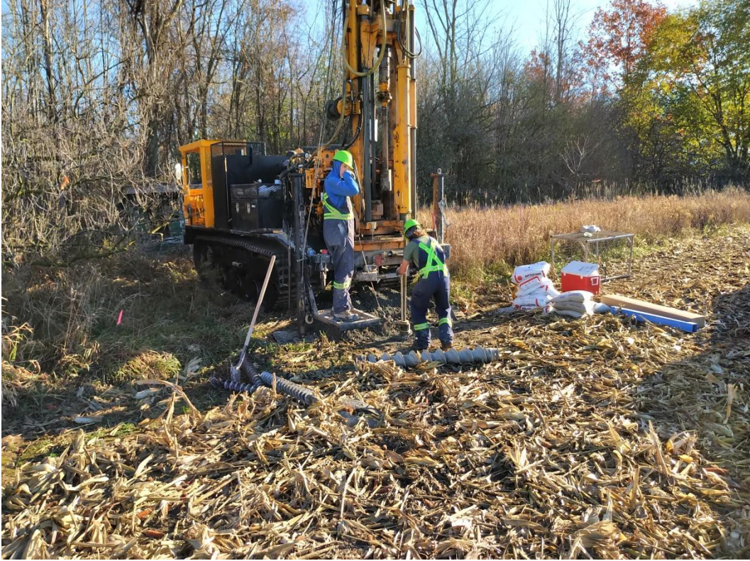
Photograph No. 7 – View of the advancement of borehole MW103-20.
