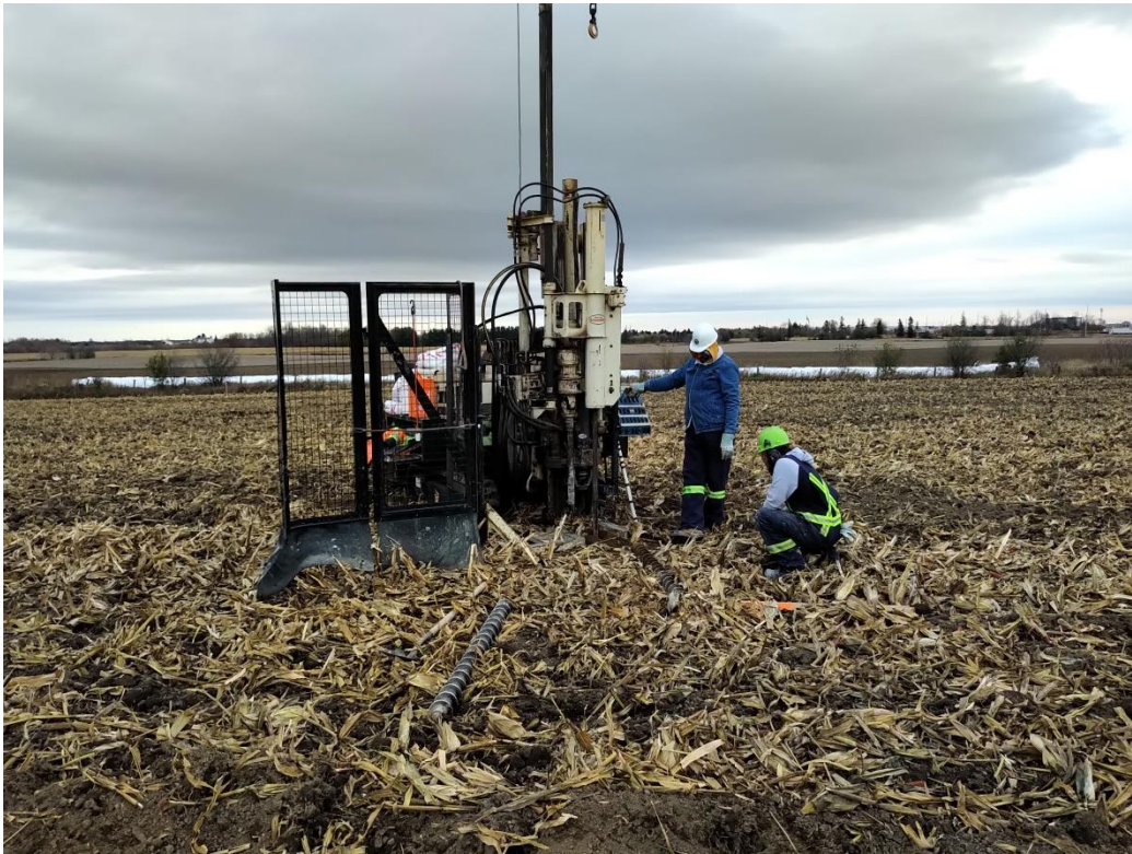
Photograph No. 9 – View of the advancement of borehole BH135-20.
