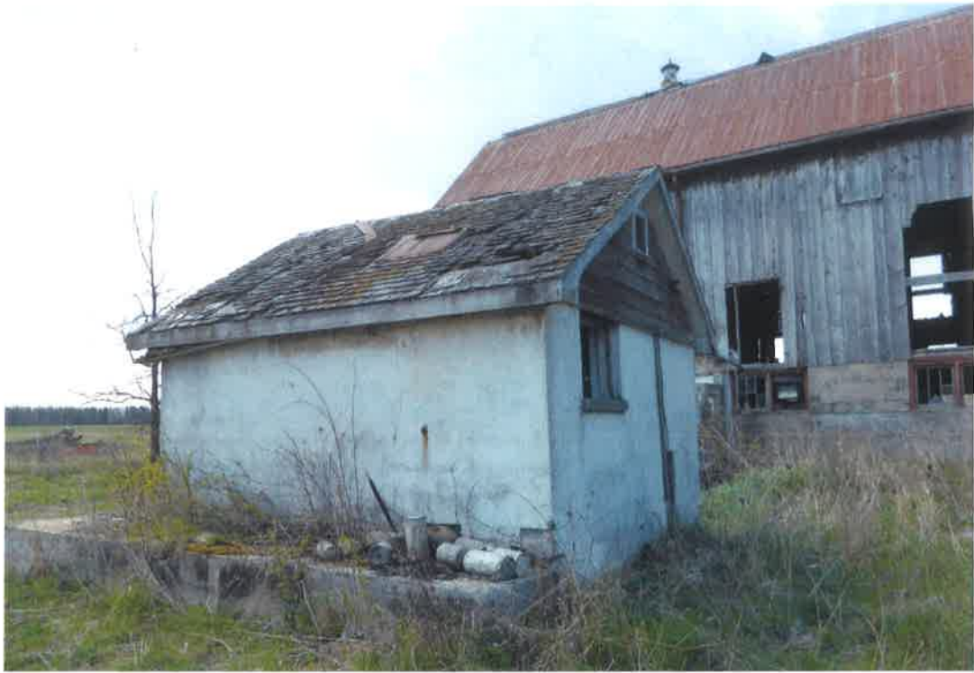
View of a Storage Shed (Looking Southwest)
