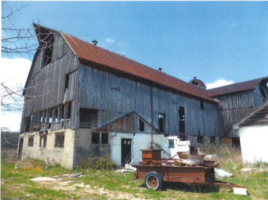
View of the Livestock Barn (Looking West)
