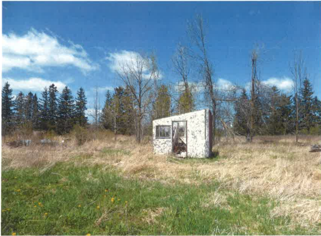
View of a Storage Shed (Looking Northwest)
