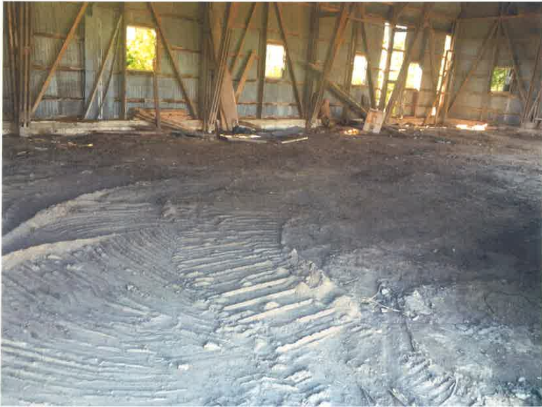
General View of the Interior of the Storage Barn
