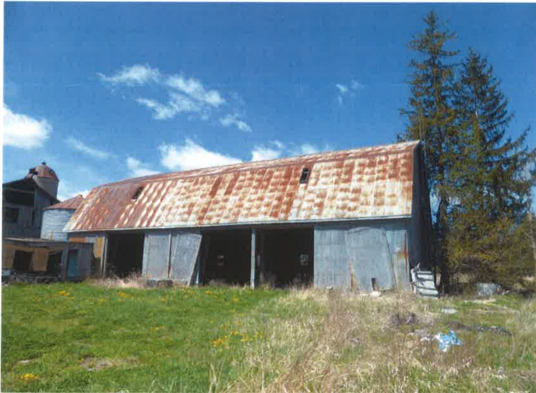
View of the Storage Barn (Looking Northwest)
