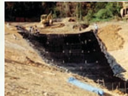
Stabilized Spillway with Geoweb®/TRM Solution
