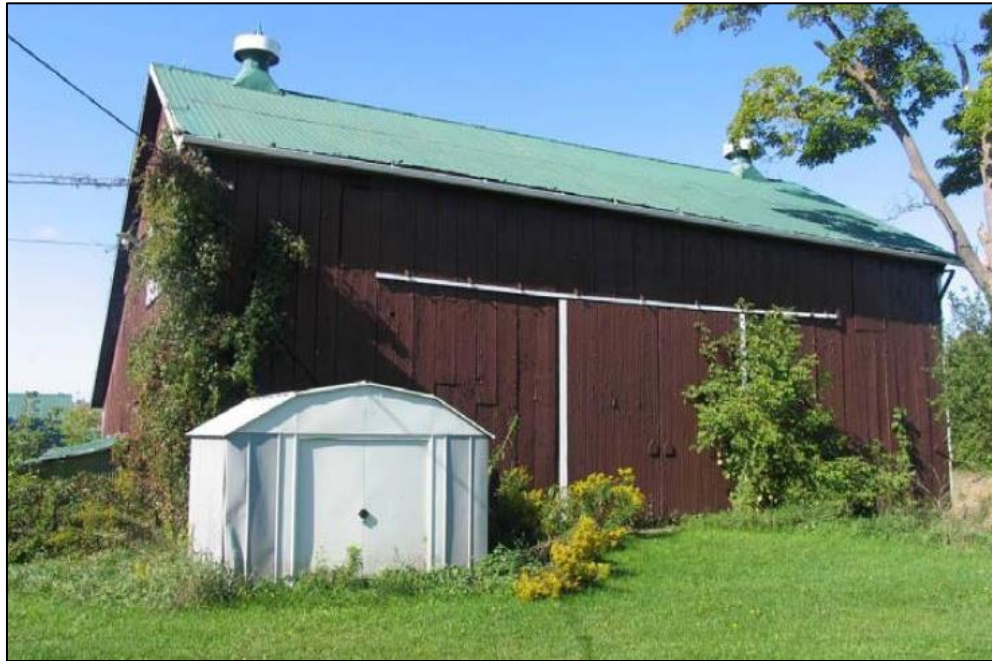
South and East Elevations
