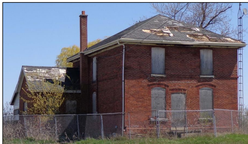
Figure No. 7.4 Deterioration in the Giffen House - 12461 McLaughlin Road – missing roof singles
