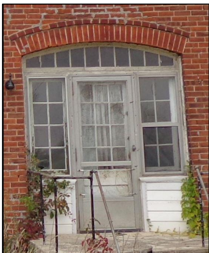
2017 - Entrance – South Elevation
