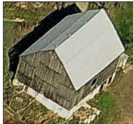
Barn – West and South Elevations; now on separate property
