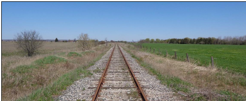
May 2022 – Adjacent – Railway at Old School Road looking north
