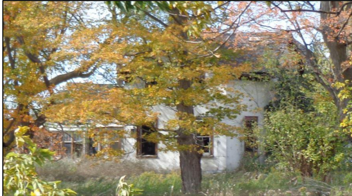
South and East Elevations
