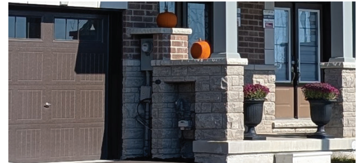
Figure 5.4.10b: Example of recessed / screened utility meters
