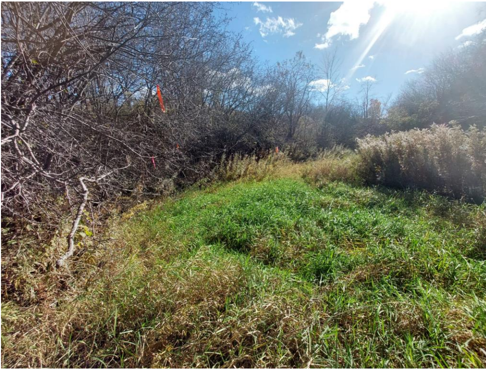
Photograph 3 - Section A-A toe of slope [looking south]
