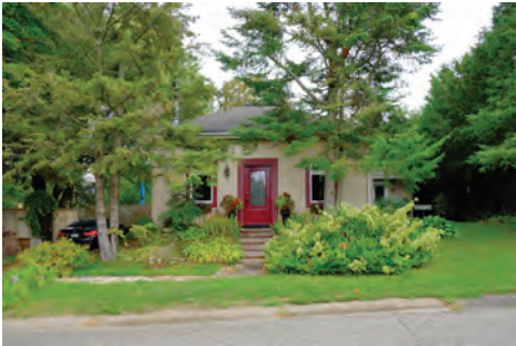
7 Agnes St., Alton, Ontario. Source: ATA Architects, 2022.
