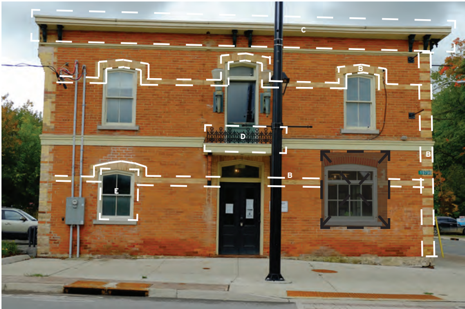
19788 Main Street, Alton, Ontario Source: ATA Architects Inc. (2022)
