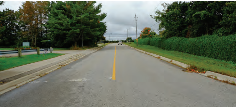
4. View West on Queen St. W. towards John St. Source: ATA Architects Inc. 2022
