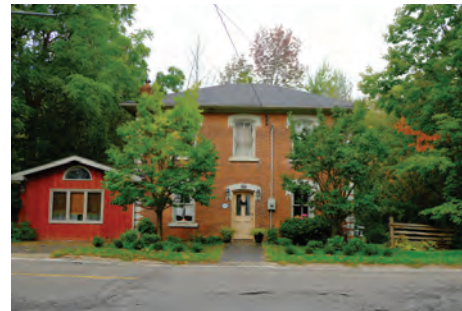
1422 Queen St. W., Alton, Ontario in a Georgian Style Source: ATA Architects, 2022.
