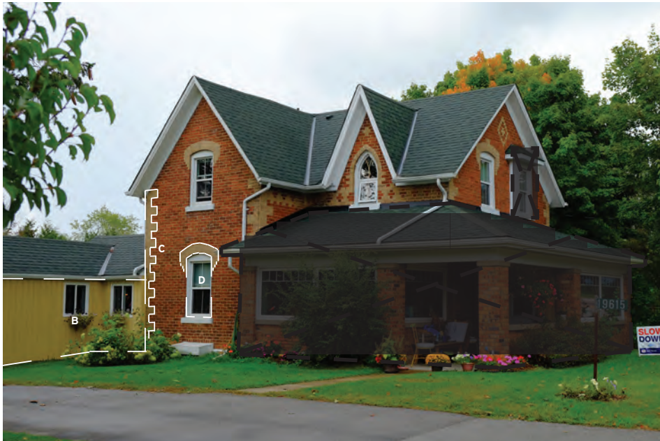
19615 Main Street, Alton, Ontario Source: ATA Architects Inc. (2022)
