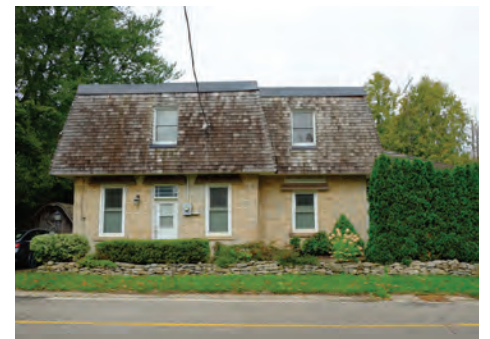
2. 1334 Queen Street W (Algie - Hall House)
