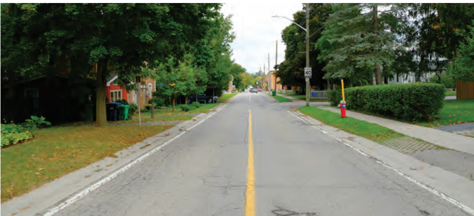
12. View East on Queen Street West, at Alton Mill. Source: ATA Architects Inc. 2022
