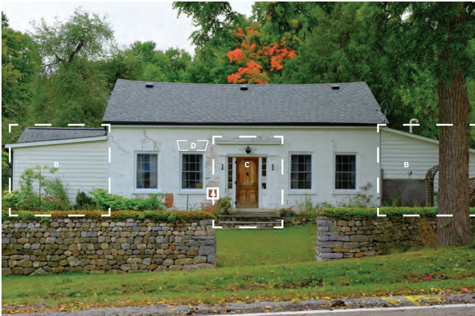
19876 Main Street, Alton, Ontario Source: ATA Architects Inc. (2022)
