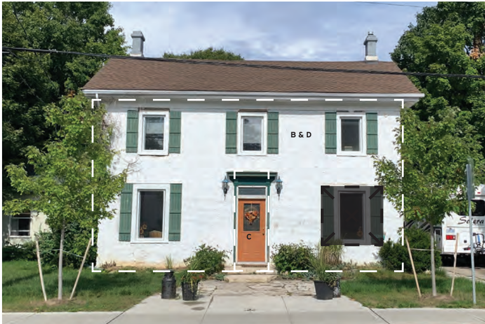
19767 Main Street, Alton, Ontario Source: ATA Architects Inc. (2022)
