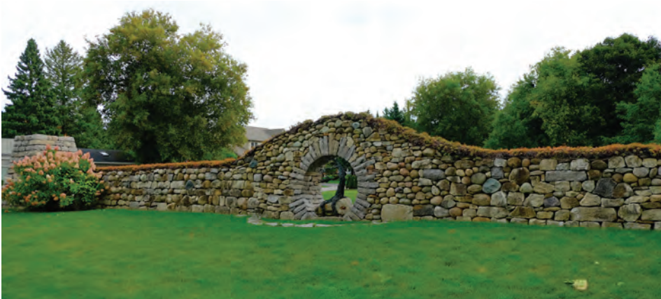
Queen Street West at Victoria Street - Alton Village Square, example of a Dry Stone Wall. Source: ATA Architects, 2022.
