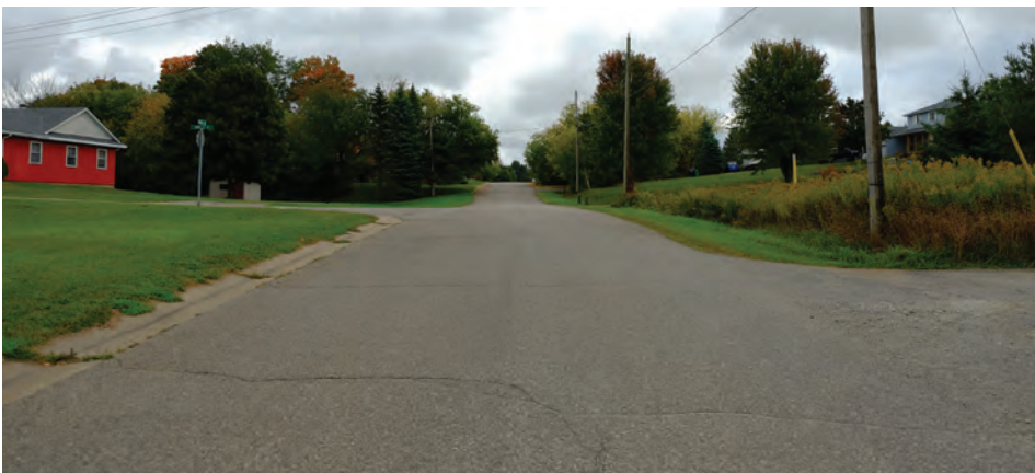
8. View South on Agnes St. Source: ATA Architects Inc. 2022
