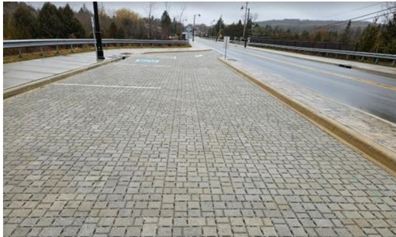
Permeable pavers for parking area, Queen St East, Alton
