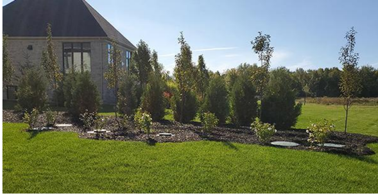
Waterloo Biofilter System - landscaped area with access lids
