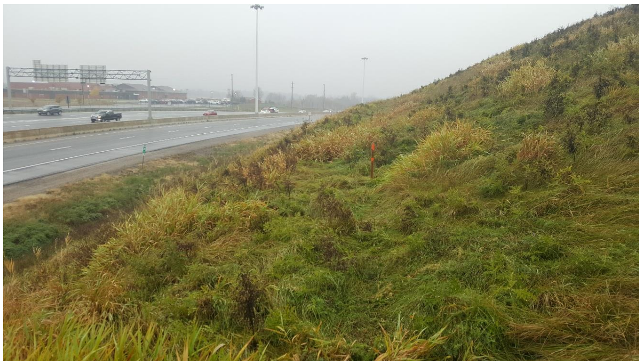
Photograph 2: View of from mid-slope of existing berm, looking north (5 November 2018).
