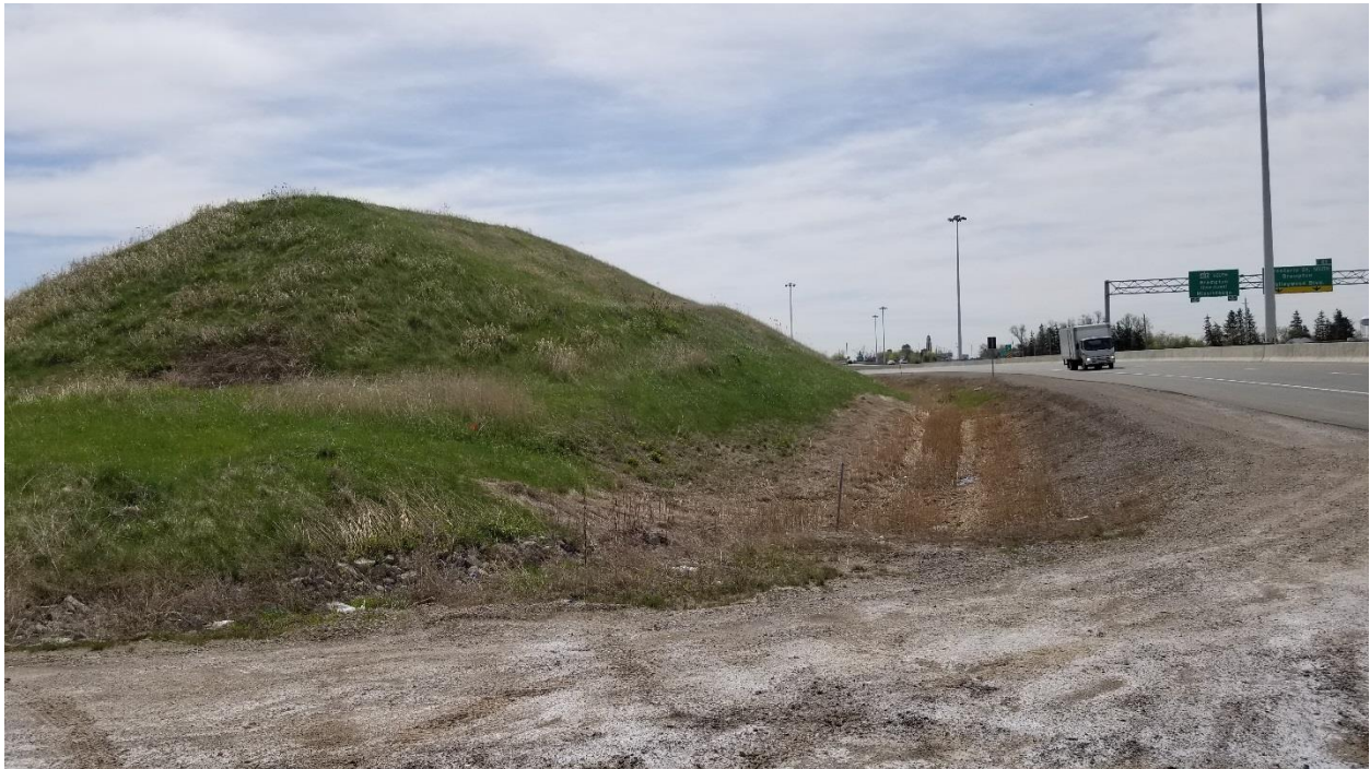
Photograph 3: View of Hwy 410 northbound lanes and existing berm, looking south (5 November 2018).
