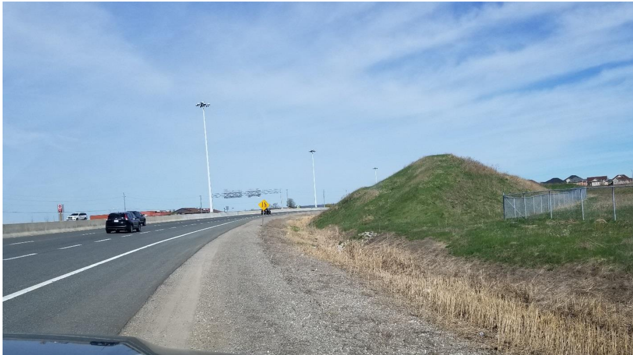
Photograph 1: View of Hwy 410 northbound lanes and existing berm, looking north (5 November 2018).
