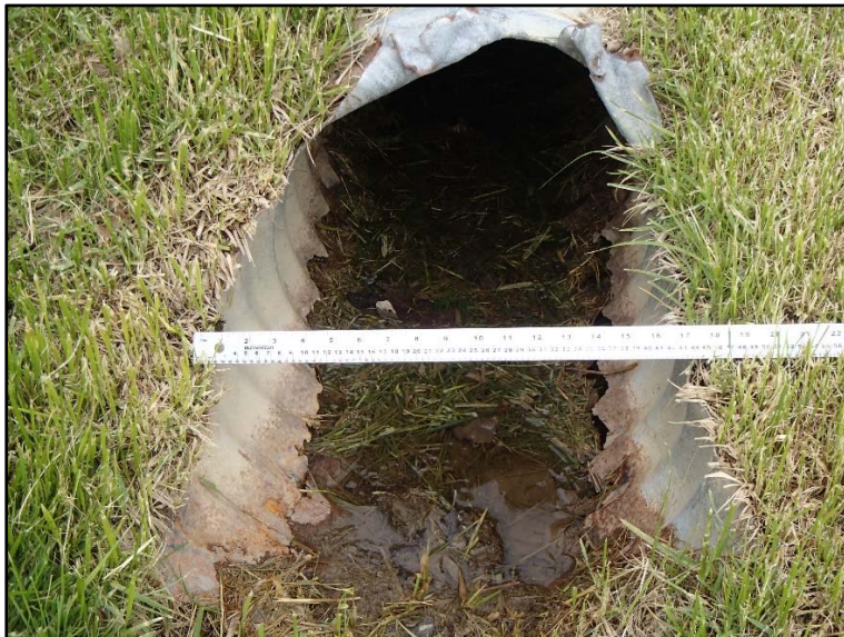
Photo 7: 2017-05-24, culvert inlet at C7a.
