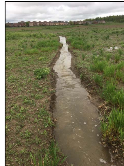
Photo 20: 2017-05-26, drainage feature C14 looking downstream.
