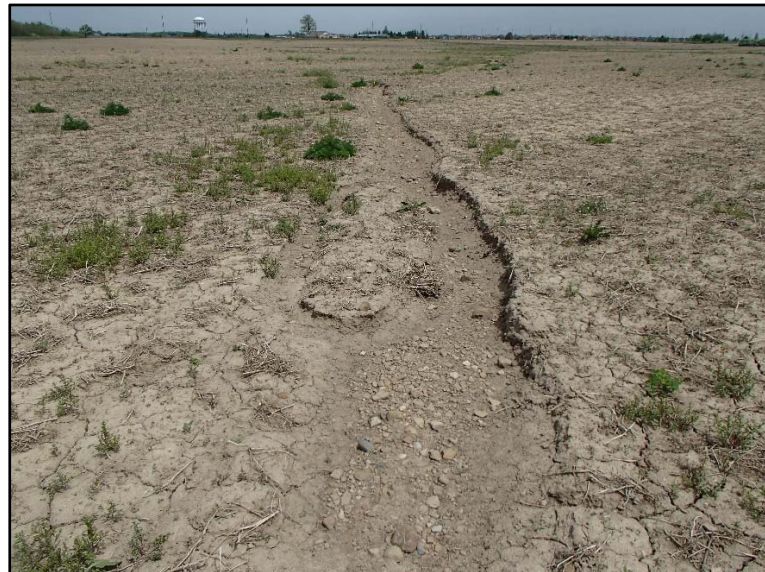
Photo 3: 2017-05-24, drainage feature C3 looking downstream.
