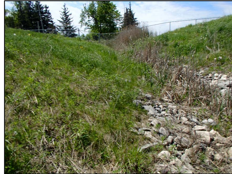
Photo 26: 2017-05-24, roadside drainage at D4, looking west.
