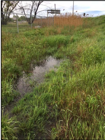
Photo 25: 2017-05-26, roadside drainage at D3, looking south
