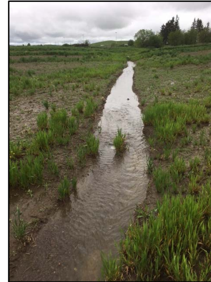
Photo 22: 2017-05-26, drainage feature C14 looking upstream.
