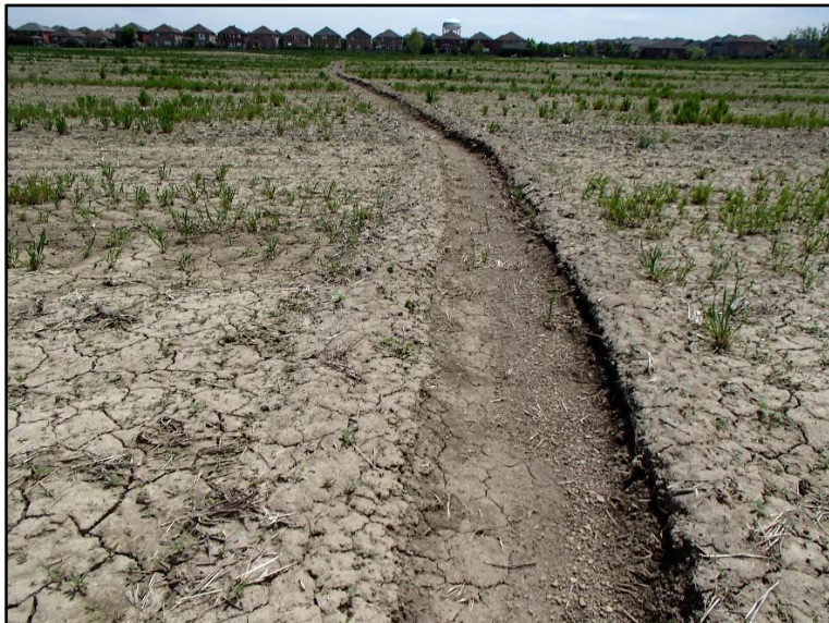
Photo 15: 2017-05-24, drainage feature C12 looking downstream.
