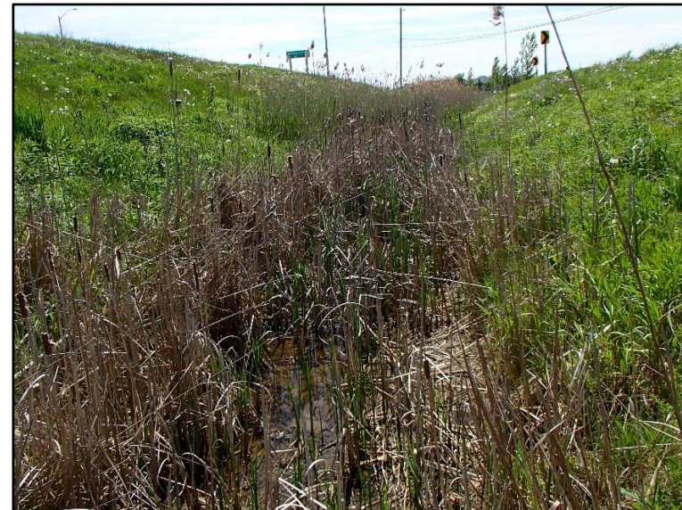
Photo 24: 2017-05-24, roadside drainage at D2 looking south.
