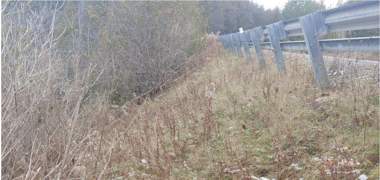
Photograph 14 – Guardrail and downslope on north side of roadway
