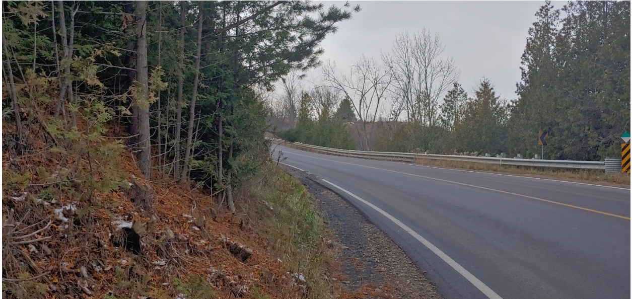
Photograph 12 – Columbia Way looking west at eastern limit of upslope
