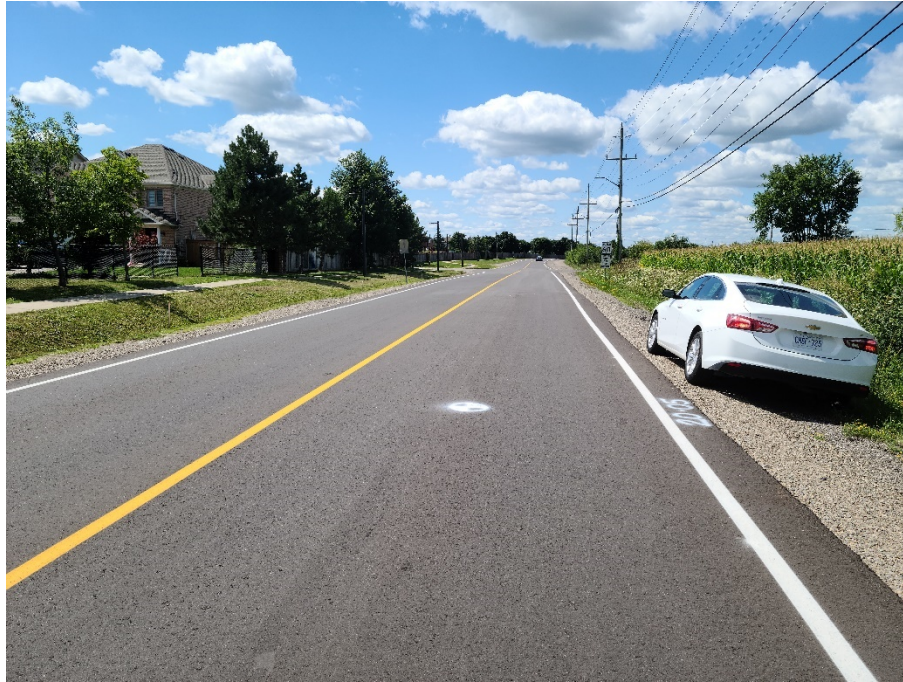
Photograph 7 – Columbia Way looking west at Borehole 20-05
