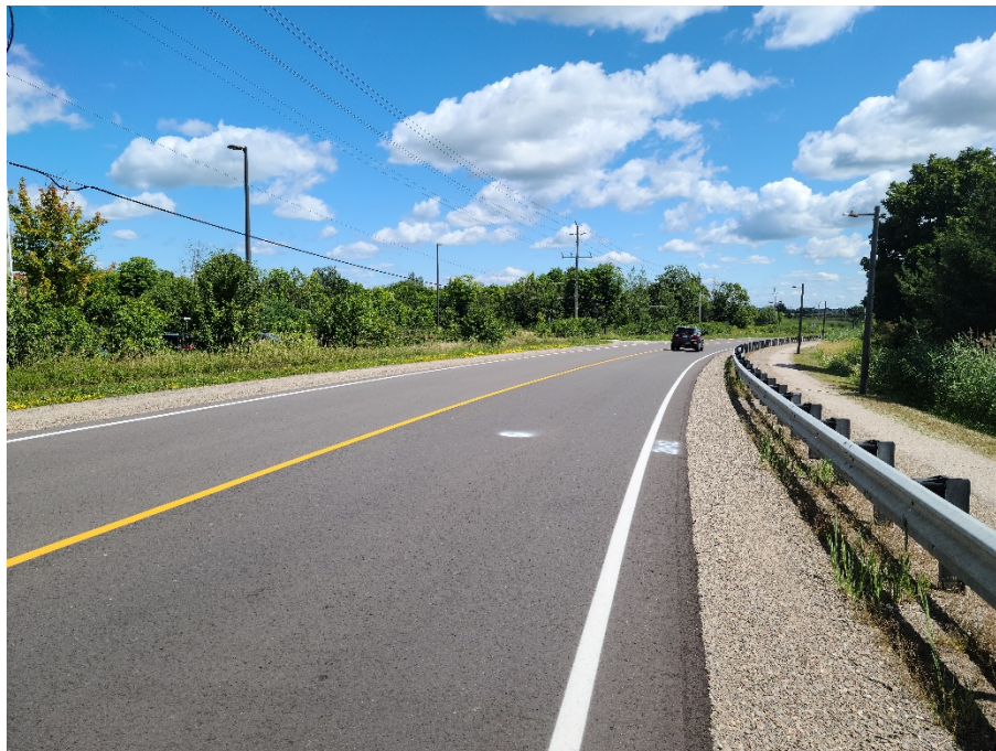
Photograph 2 – Columbia Way looking east at Borehole 20-02
