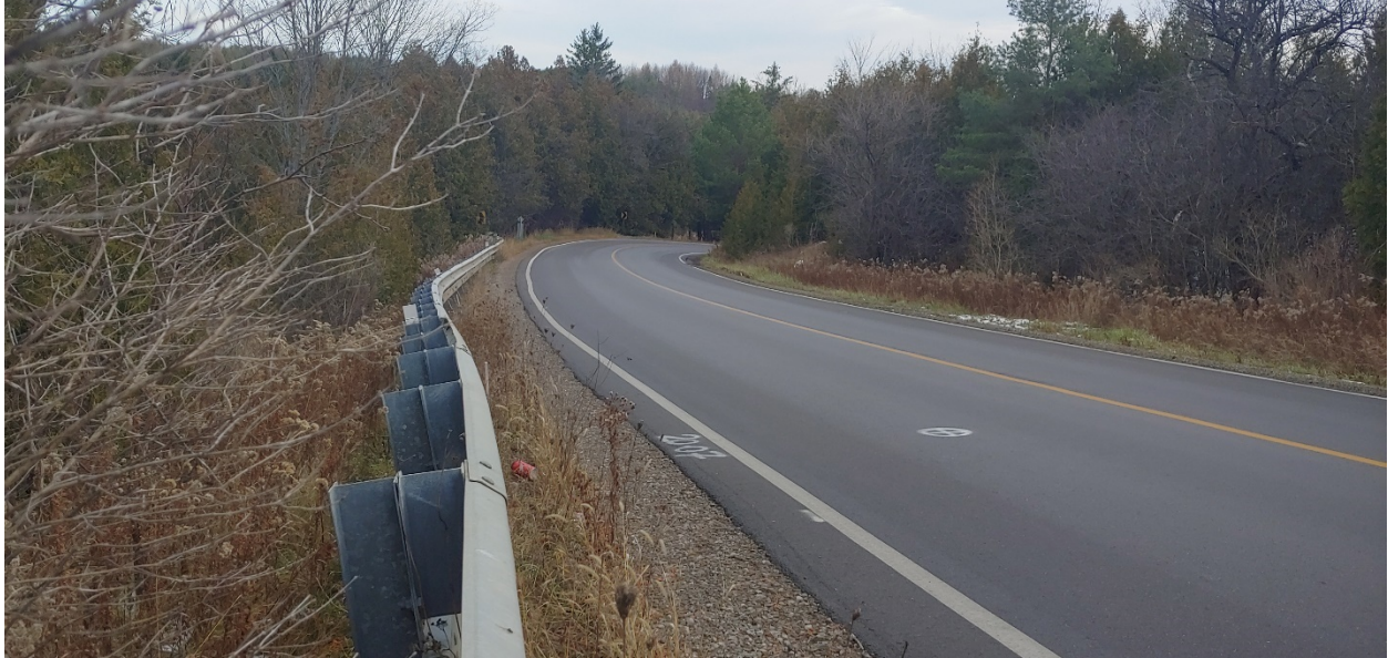
Photograph 13 – View of guardrail looking south towards guardrail movement
