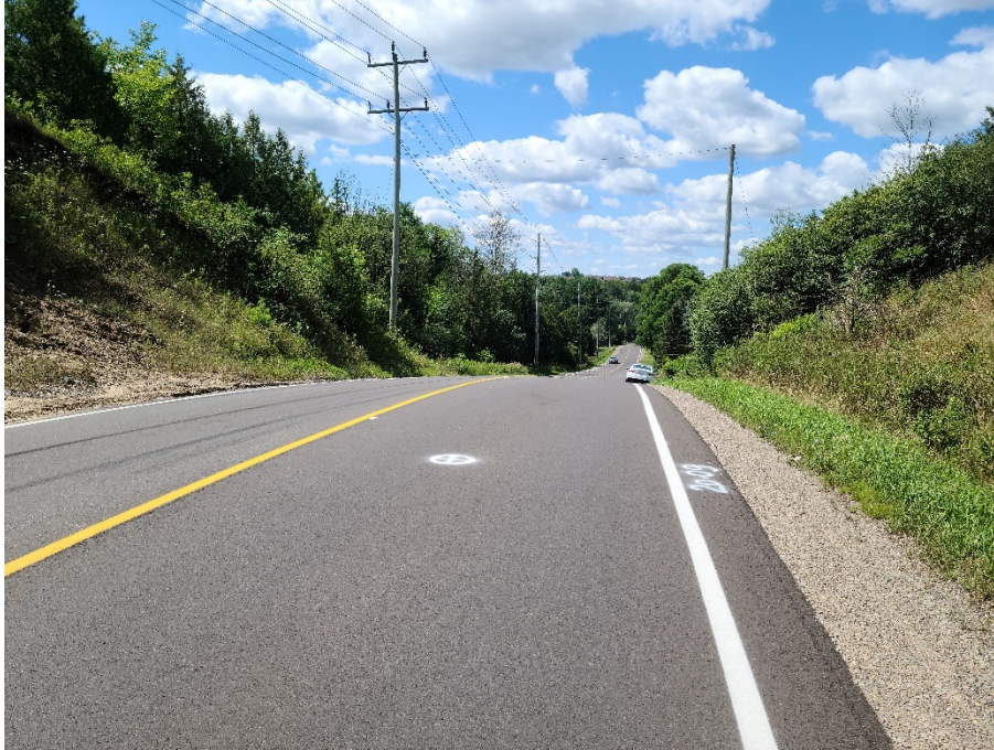
Photograph 17 – Columbia Way looking west from Borehole 20-09
