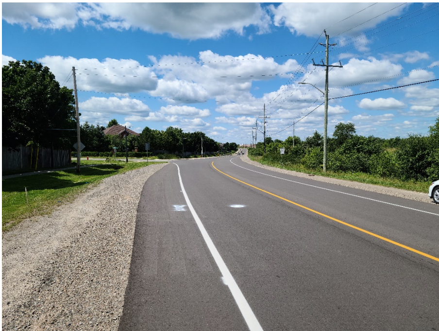
Photograph 6 – Columbia Way looking west at Borehole 20-04
