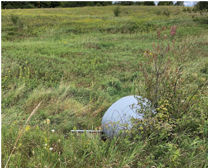
Photograph 4 – View of culvert looking north approximately 0.9 km east of Highway 50
