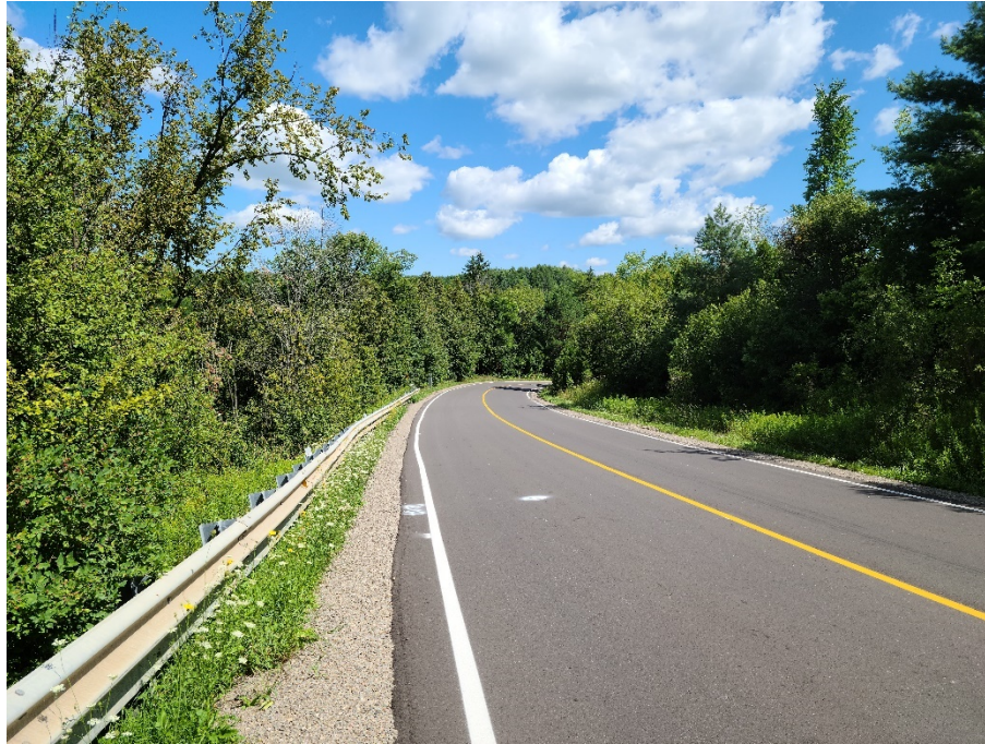
Photograph 9 – Columbia Way looking east at Borehole 20-07
