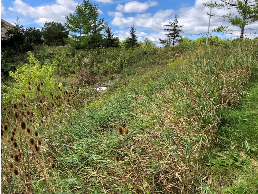
Photograph 5 – View of south slope at culvert approximately 0.9 km east of Highway 50
