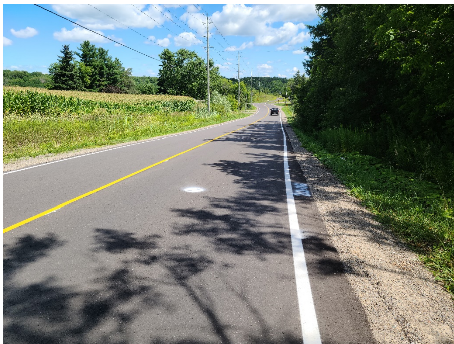
Photograph 8 – Columbia Way looking east at Borehole 20-06
