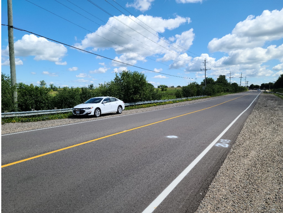
Photograph 3 – Columbia Way looking east at Borehole 20-03
