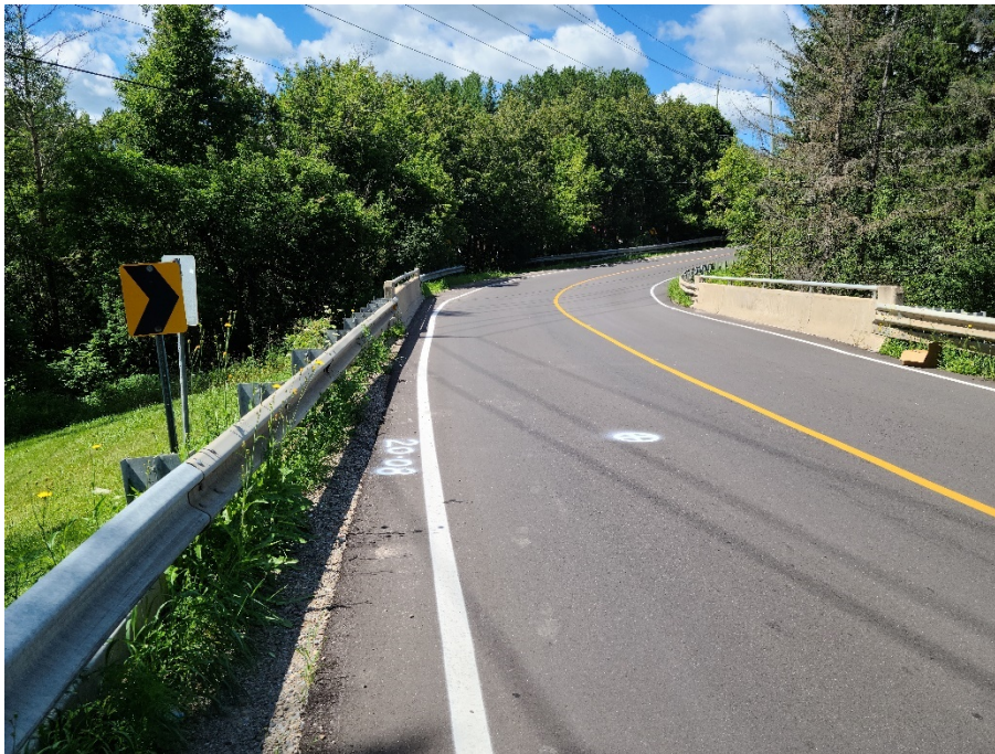
Photograph 16 – Bridge on Columbia way at Borehole 20-08 looking west over Cold Creek
