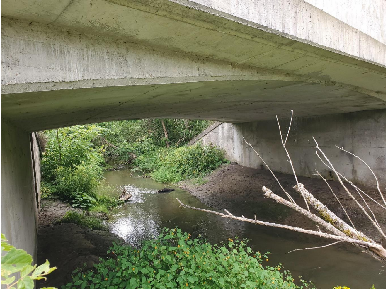
Figure 5 – Underside of Bridge, looking south
