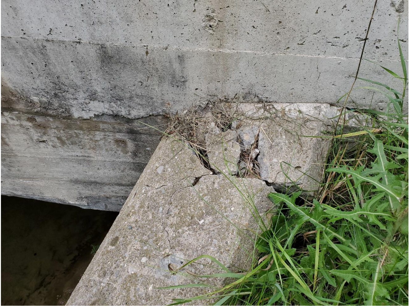
Figure 11 – Structural failure at connection between east abutment and southeast wingwall
