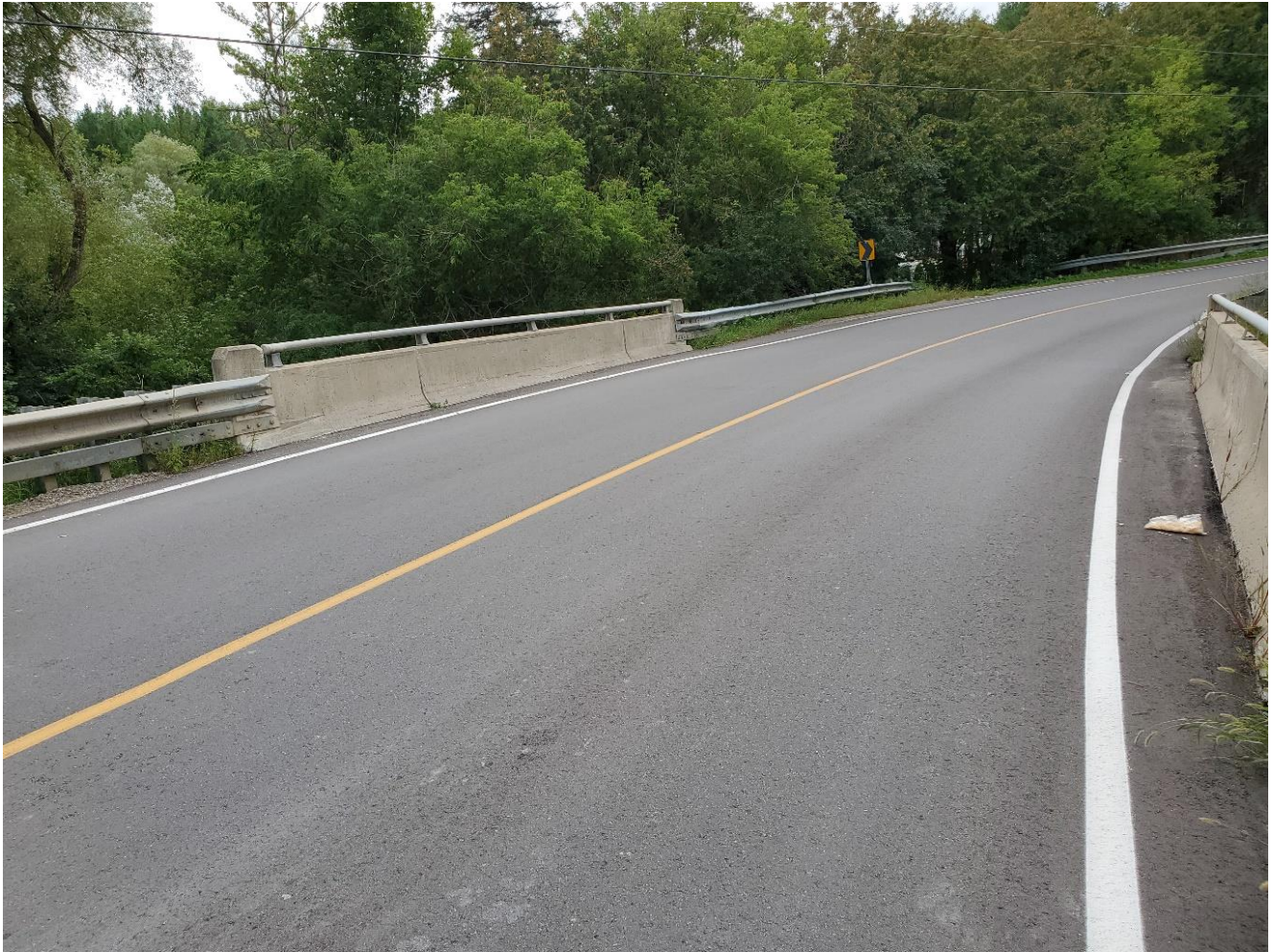
Figure 1 – View of Bridge, looking West
