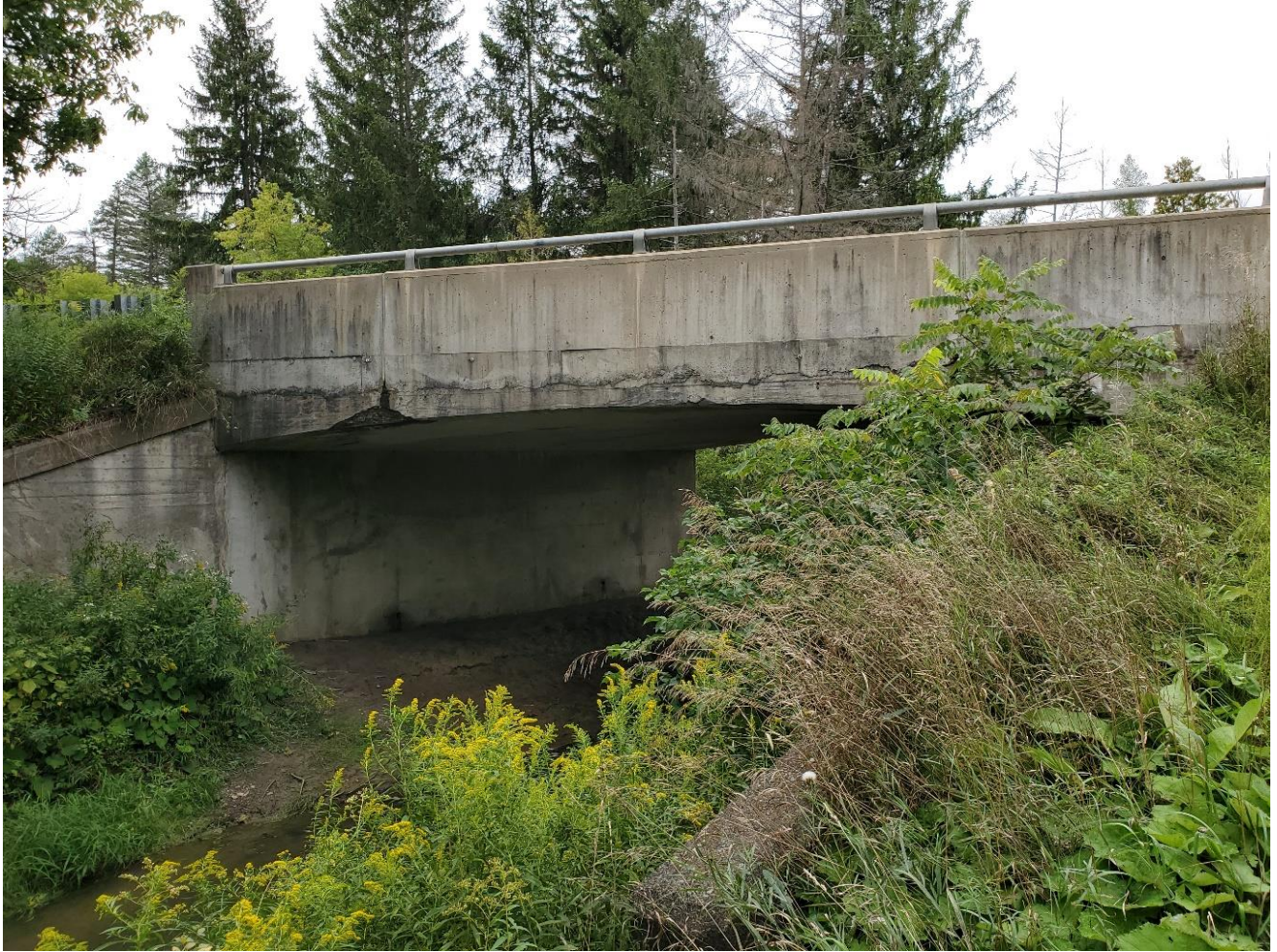
Figure 12 – South elevation of Bridge
