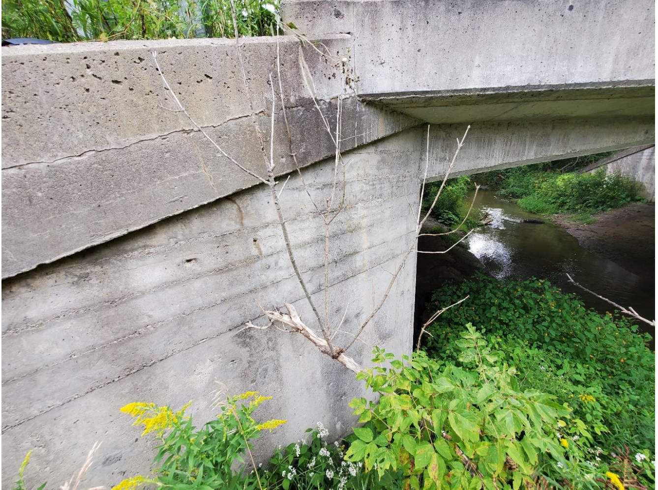
Figure 3 – Northeast Wingwall at Abutment
