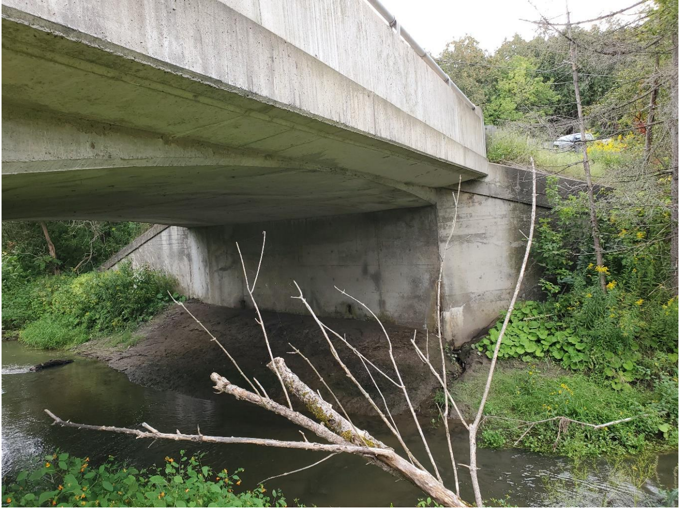
Figure 4 – Underside of Bridge, looking west
