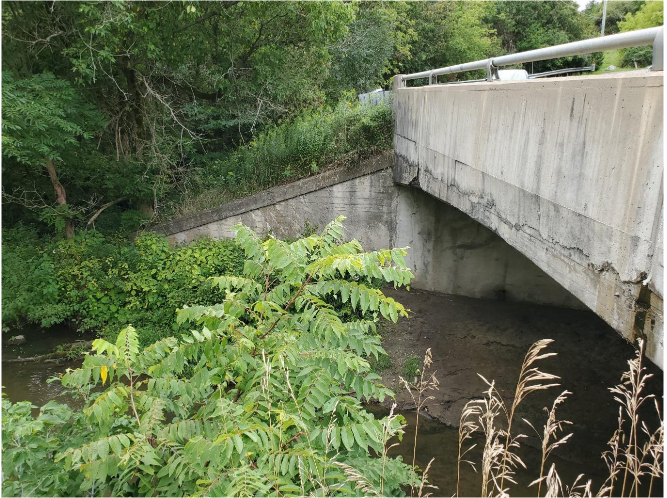
Figure 10 – South side of bridge, southwest wingwall
