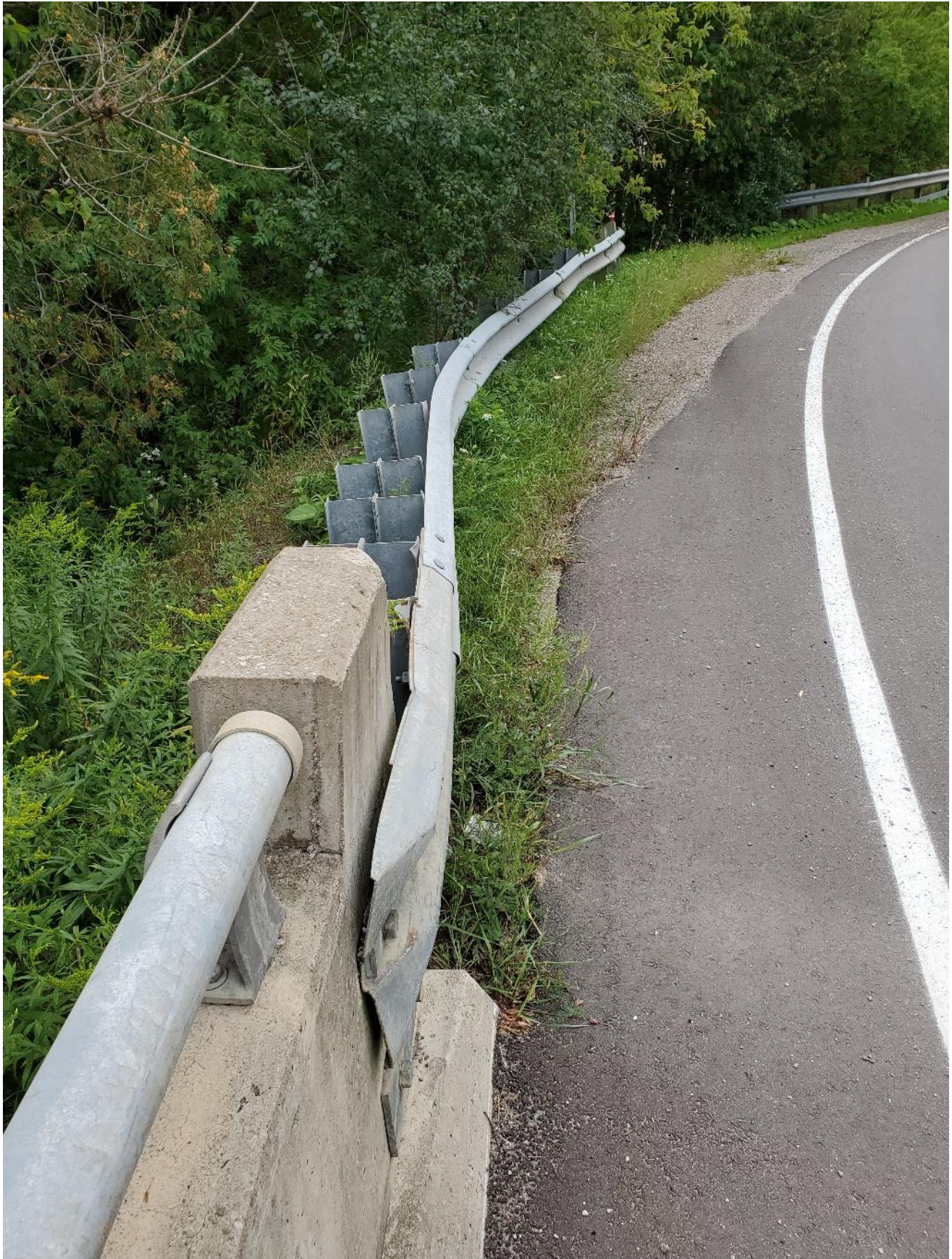
Figure 15 – Damaged southwest guiderail
