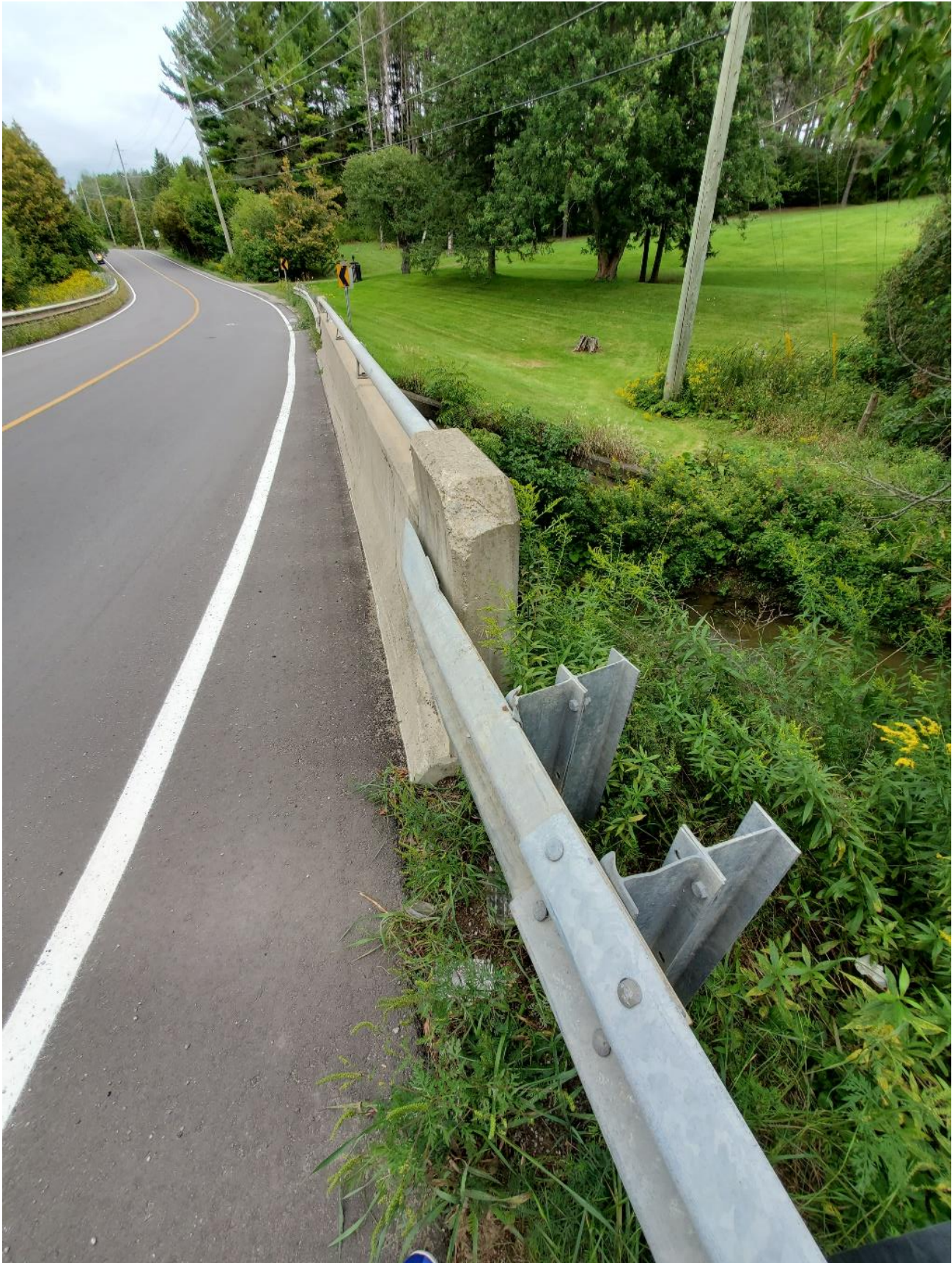
Figure 16 – Damaged southwest guiderail
