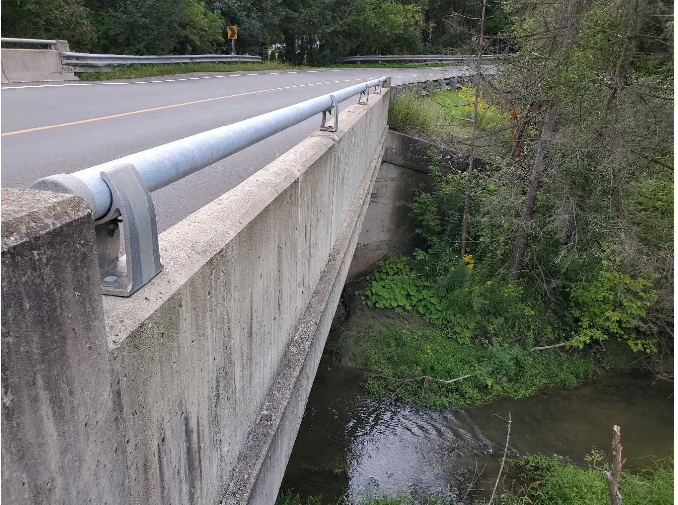
Figure 2 – North Parapet Wall and Railing, Northwest Wingwall
