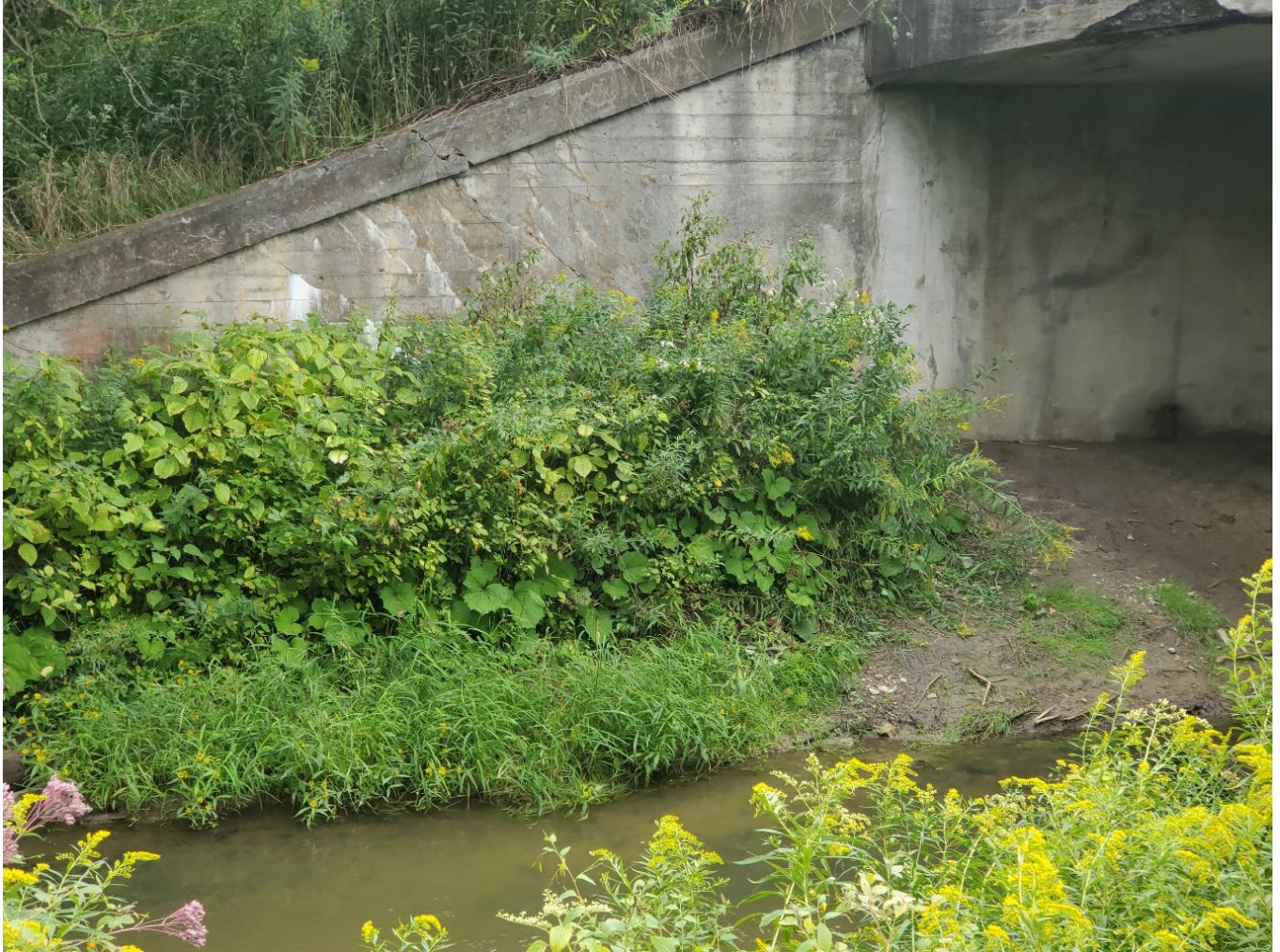
Figure 13 – Southwest wingwall (cracking visible)
