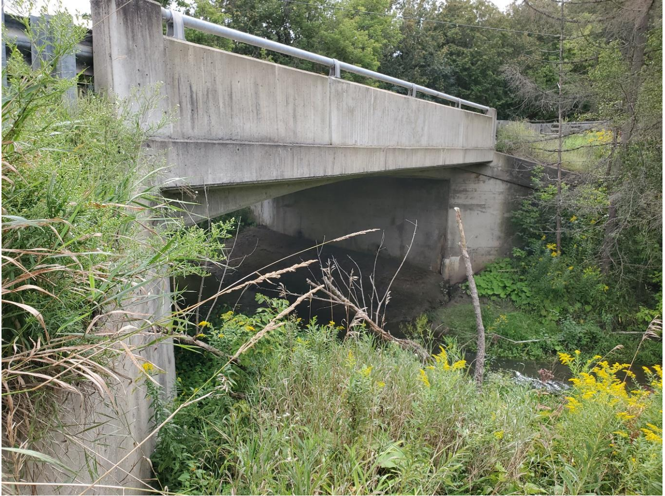
Figure 6 – North Elevation of Bridge
