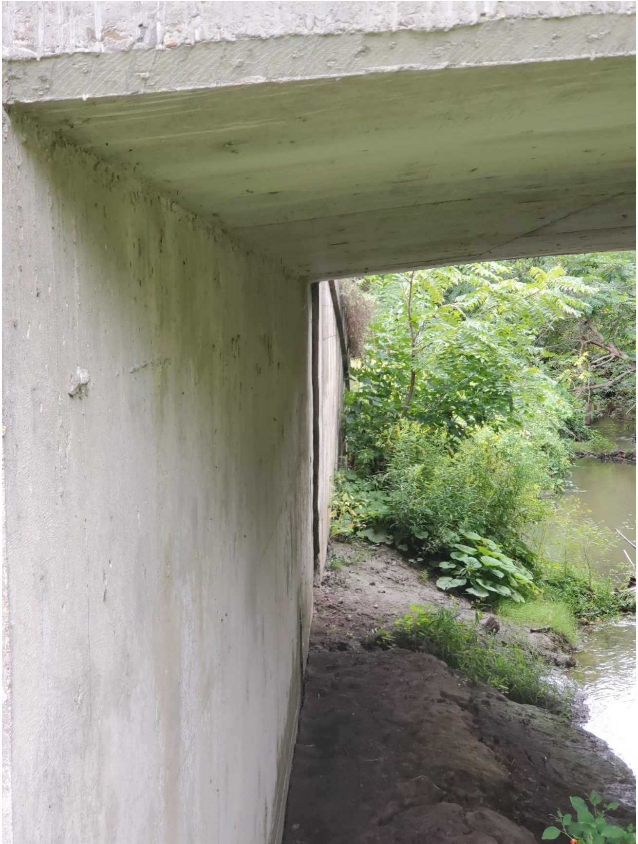
Figure 8 – East abutment, looking south shifted southwest abutment visible)
