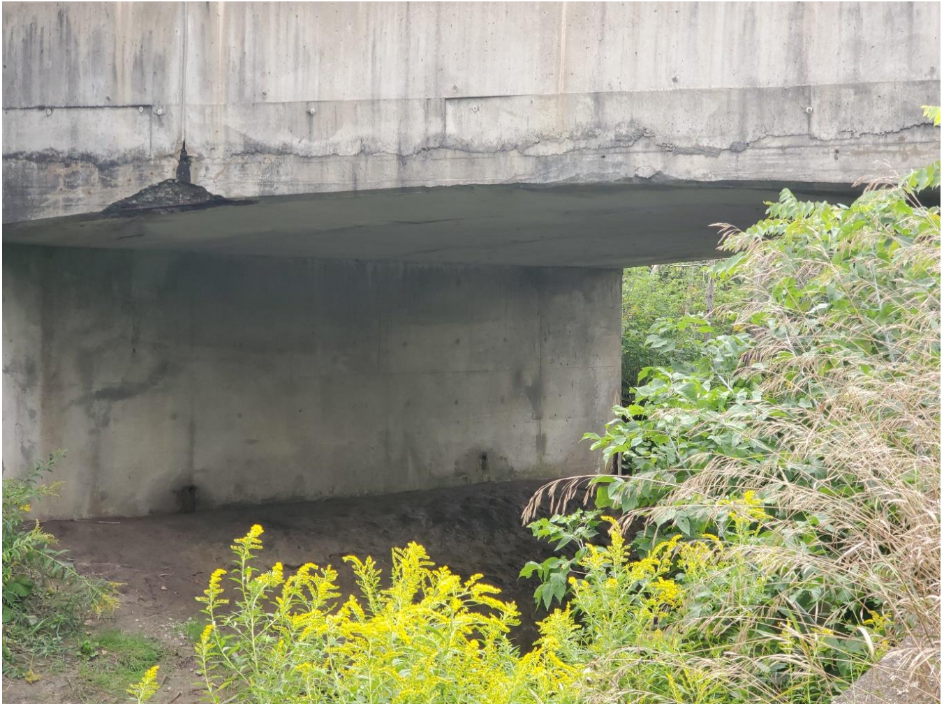
Figure 14 – Soffit of bridge looking north (spalling visible)
