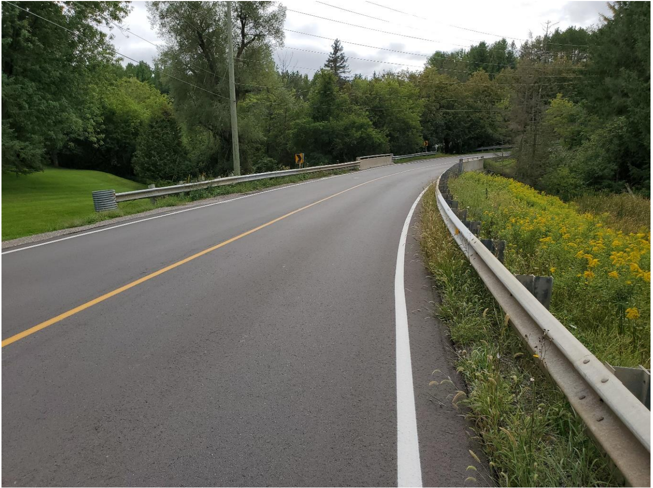
Figure 7 – Guiderails at east side of Bridge
