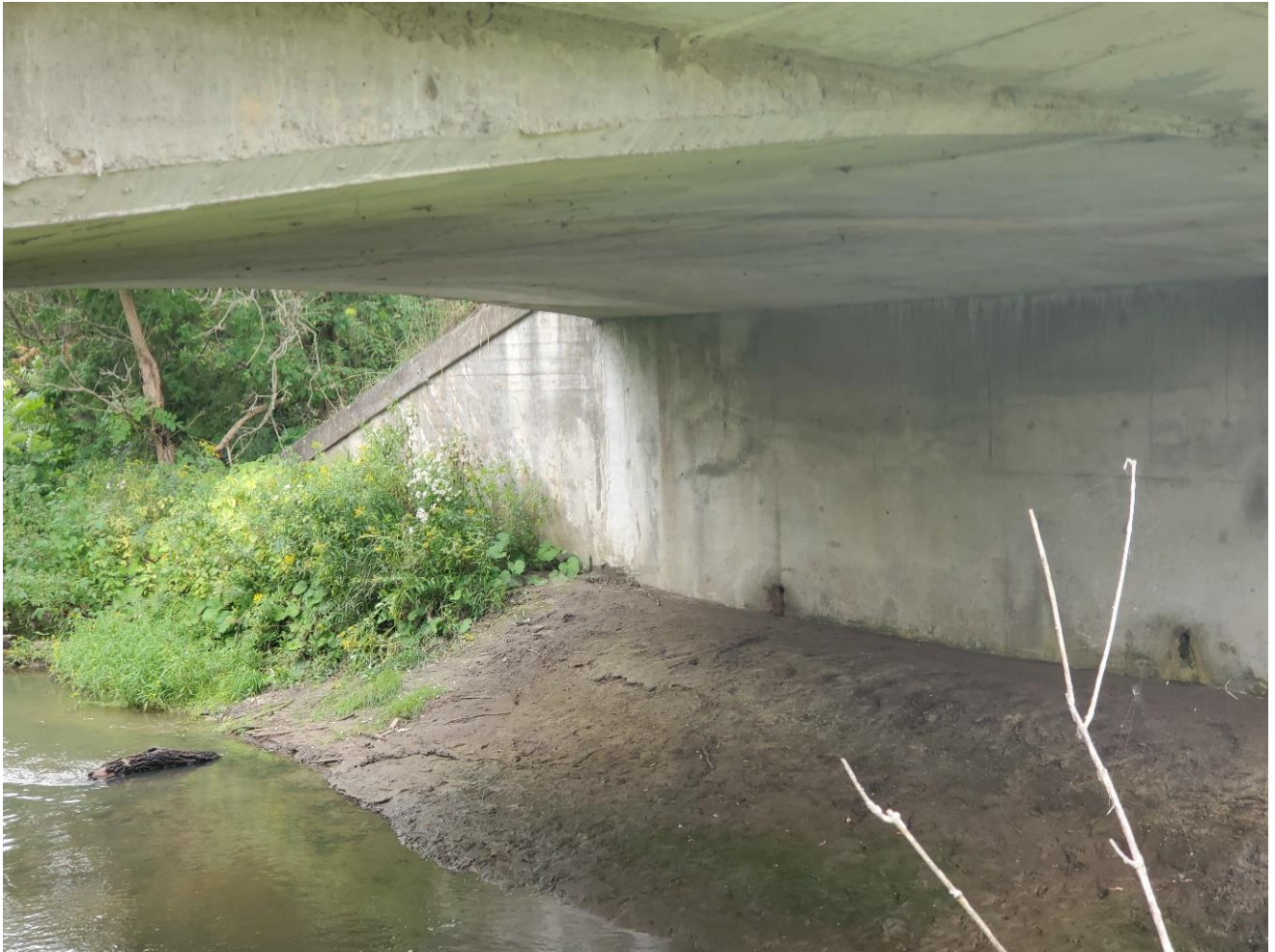
Figure 9 – West abutment and soffit, looking west
