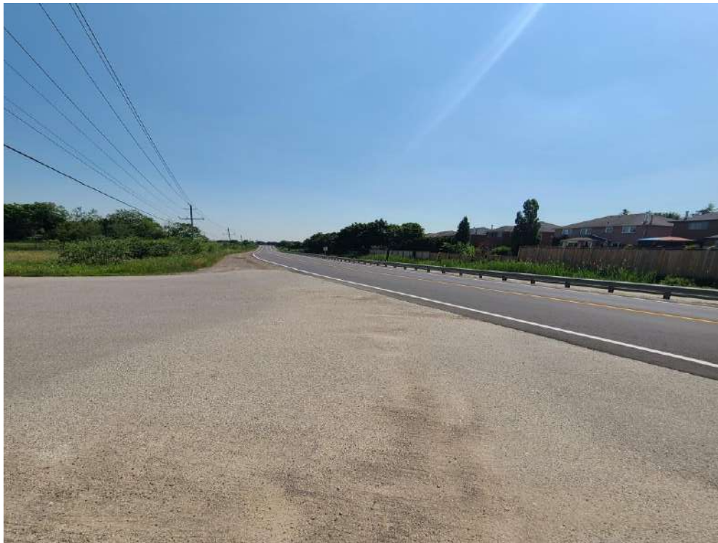
Photo 1: View of Columbia Way to the east/northeast, 600m east of Highway 50.
