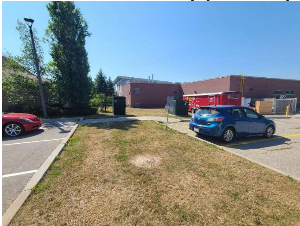
Photo 16: View to the southwest showing two of the pad-mounted green transformer boxes located on the Caledon Recreation Centre at 14111 Highway 50.
