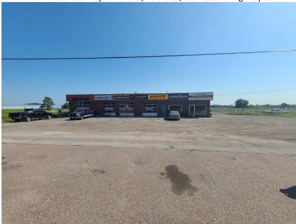
Photo 2: View to the East showing an automotive garage (former YG's gas bar), approximately 250m north of the Site on the east side of Hwy 50.
