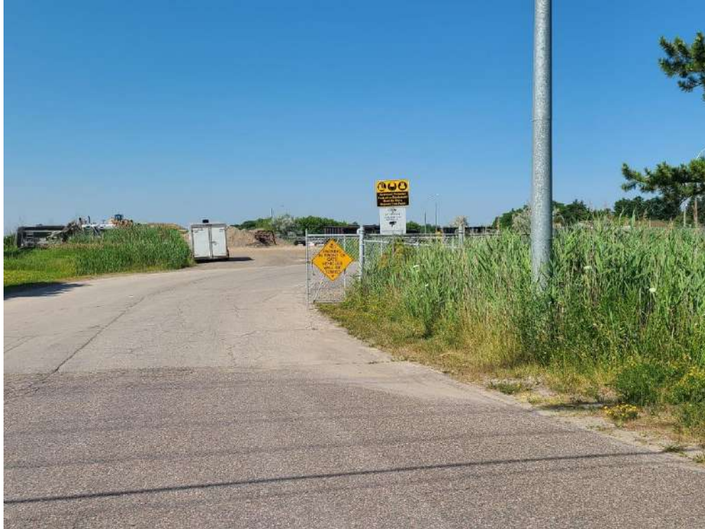
Photo 11: View to the west showing the fill, construction material and equipment located at 14220 Highway 50.
