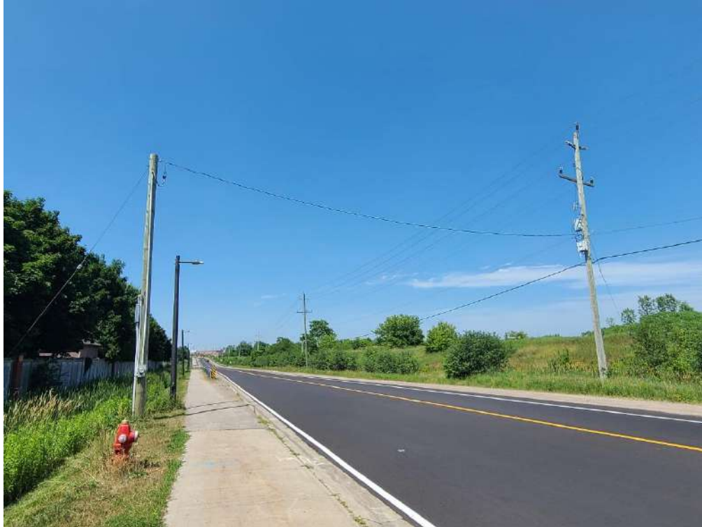
Photo 17: View to the southwest showing one of the pole-mounted located along Columbia Way.
