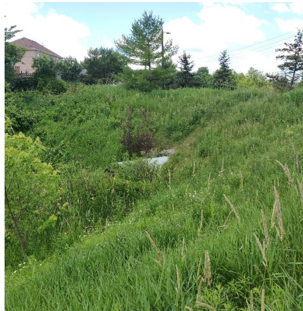
Plate 4: Trail system and channelized watercourse with modern culvert; disturbed
