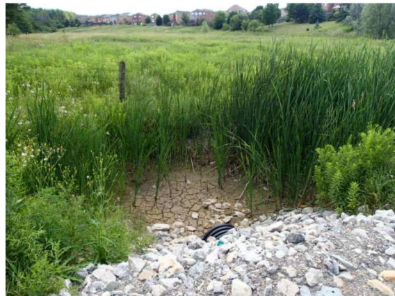
16 - July 31, 2020 Small surface drainage culvert outlet to private pond, south of Columbia Way.
