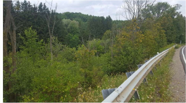
8 - August 27, 2020 Vegetation along west side of S-bend proposed for removal to support slope stabilization via grading.
