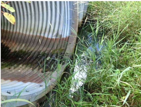
15 - July 31, 2020 Upstream end of Cold Creek tributary culvert, note perched (elevated) above ground.
