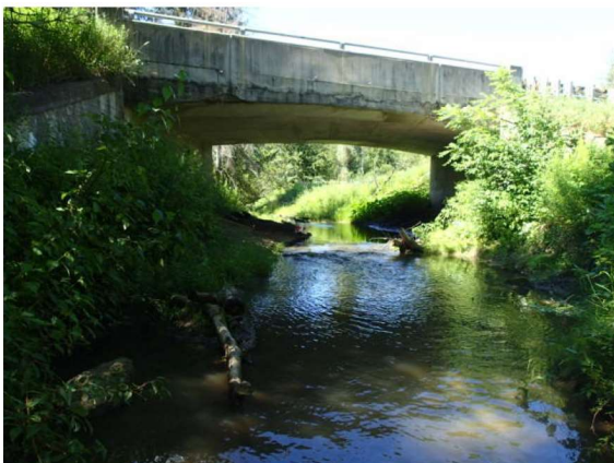
23 - July 31, 2020 Coventry Bridge, looking upstream.
