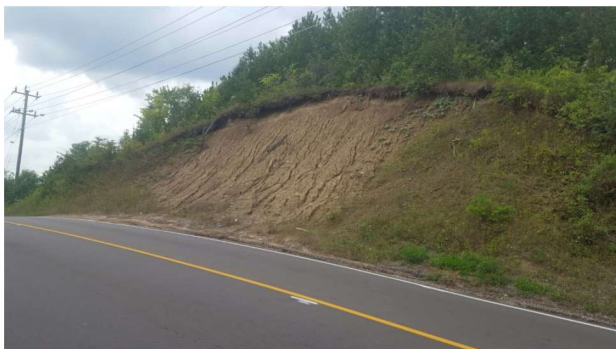
11 - August 27, 2020 Eroding bank near Caledon-King Townline Road.
