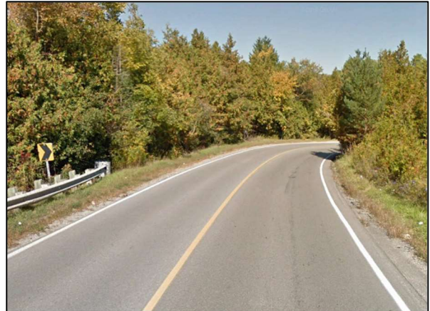
Figure 2: Columbia Way approaching S-curve
