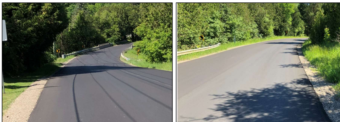
Figure 5: Insufficient Chevron Signage on S-bend
