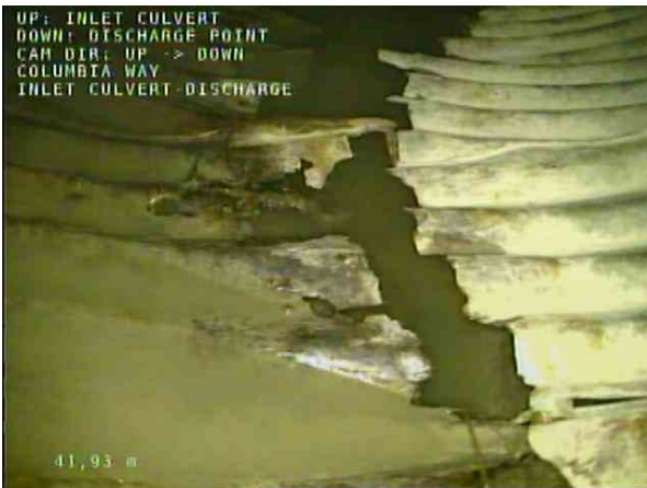
INLET CULVERT-DISCHARGE_57bbdf5-fc42-447f-b7a9-927a3f772709_20201208_095644_479.jpg, 00:17:25, 41.93m Surface Damage Reinforcement Corroded from 5 o'clock to 7 o'clock, Start
