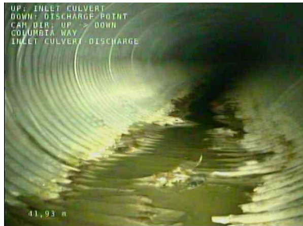
INLET CULVERT-DISCHARGE_76b68f24-d6bf-4149-ad94-c6724d9b2ed2_20201208_095649_733.jpg, 00:17:25, 41.93m Surface Damage Reinforcement Corroded from 5 o'clock to 7 o'clock, Start
