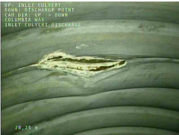
INLET CULVERT-DISCHARGE_24f5fdd5-cfb6-44e4-ad23-61af7d9d9f00_20201208_094946_883.jpg, 00:10:26, 28.25m Surface Damage Other at 10 o'clock / METAL BENDED
