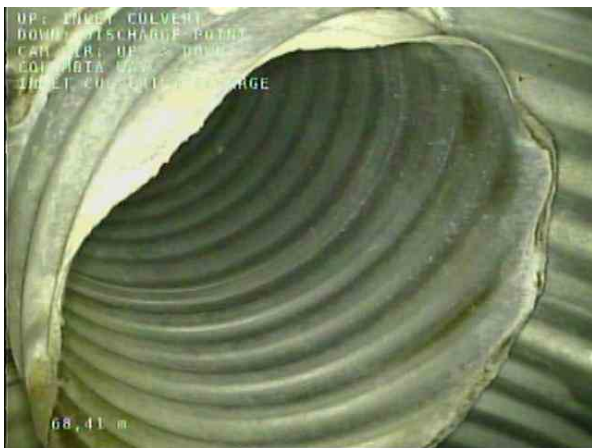
INLET CULVERT-DISCHARGE_7071ec05-3465-4536-812a-beacd65edb72_20201208_100446_340.jpg, 00:25:26, 68.41m Tap Break-In Intruding at 10 o'clock, 450mm dim, 200mm intrusion
