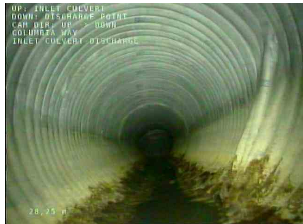
INLET CULVERT-DISCHARGE_148a401d-b0e9-4863-9b5b-5b105e2496ce_20201208_095107_264.jpg, 00:11:47, 28.25m Deformed Flexible Bulging Inverse Curvature, 10% changed from 2 o'clock to 5 o'clock / METAL DEFORMED
