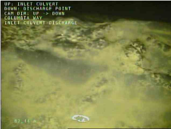
INLET CULVERT-DISCHARGE_0d2aa071-3f19-42f6-8c29-334970af3696_20201208_101241_978.jpg, 00:33:22, 82.44m Surface Damage Reinforcement Corroded from 5 o'clock to 7 o'clock, Finish
