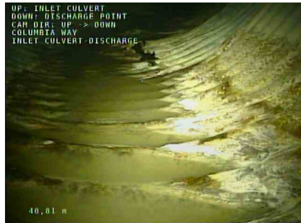
INLET CULVERT-DISCHARGE_6188b062-19c0-4427-ad26-6f1477e d9f40_20201208_095433_623.jpg, 00:15:13, 40.81m Surface Damage Corrosion from 5 o'clock to 7 o'clock, Finish
