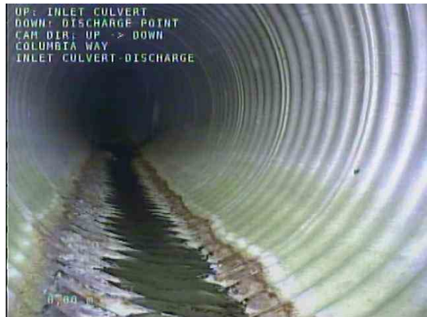
INLET CULVERT-DISCHARGE_ded7b0c2-4e08-4c00-9172-f709dcf0 d248_20201208_093632_171.jpg, 00:01:49, 0.00m Surface Damage Corrosion from 5 o'clock to 7 o'clock, Start
