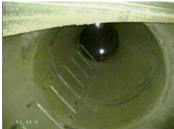
INLET CULVERT-DISCHARGE_c5f92424-ef47-4852-edef-ea4a8e891c40_20201208_101341_325.jpg, 00:34:16, 82.44m Manhole / DISCHARGE POINT
