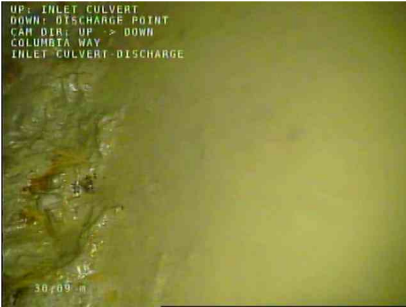
INLET CULVERT-DISCHARGE_bebdc32e-7ab0-495c-8782-3070448 62367_20201208_095213_655.jpg, 00:12:46, 30.09m Surface Damage Aggregate Visible from 5 o'clock to 7 o'clock, Start
