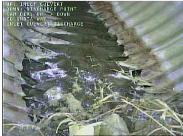
INLET CULVERT-DISCHARGE_243c1020-df6f-4283-b21e-e7004d70 d626_20201208_093527_412.jpg, 00:00:49, 0.00m Miscellaneous Water Level, 5% of the vertical dimension
