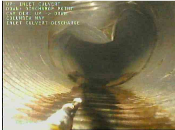
INLET CULVERT-DISCHARGE_2bc642c2-4069-4ee4-a20e-b879b4f9ffbe_20201208_101304_875.jpg, 00:33:43, 82.44m Deformed Flexible Bulging Inverse Curvature, 40% changed, Finish from 11 o'clock to 3 o'clock / PIPE BEND
