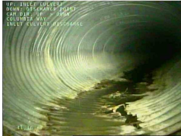
INLET CULVERT-DISCHARGE_bf60c7bb-cf42-4ba3-844c-37eb90ae1691_20201208_095546_706.jpg, 00:16:26, 41.16m Miscellaneous Shape or Size Change / OVAL CORRUGATED PIPE
