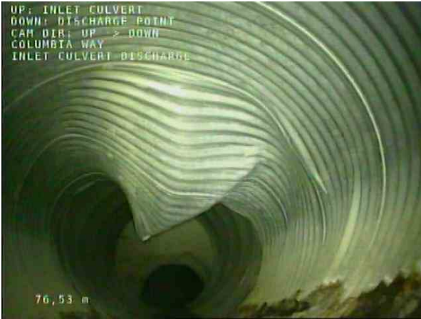
INLET CULVERT-DISCHARGE_bb2483f5-48cf-4048-a0a7-d98f62e278a2_20201208_100931_033.jpg, 00:30:11, 76.53m Deformed Flexible Bulging Inverse Curvature, 40% changed, Start from 11 o'clock to 3 o'clock / PIPE BEND
