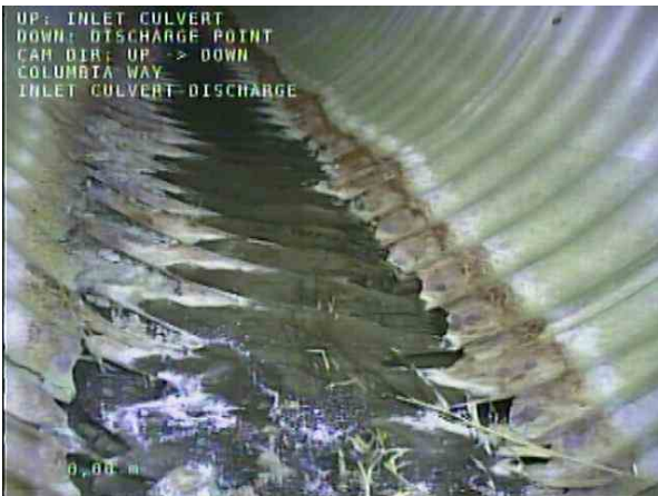
INLET CULVERT-DISCHARGE_613ebe02-6d0c-4ff9-bbec-7602c25e d51c_20201208_093628_556.jpg, 00:01:49, 0.00m Surface Damage Corrosion from 5 o'clock to 7 o'clock, Start
