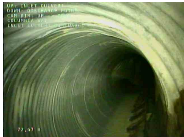
INLET CULVERT-DISCHARGE_3475fbaa-2b59-4026-a651-102acb52efb1_20201208_100652_620.jpg, 00:27:32, 72.67m Line Right, 30% changed
