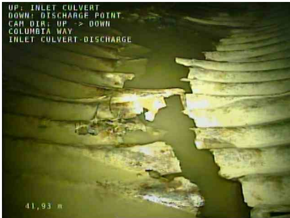
INLET CULVERT-DISCHARGE_3a33e20a-cdd5-4f3a-bf10-cfb526871de1_20201208_095723_752.jpg, 00:18:04, 41.93m Surface Damage Aggregate Visible from 5 o'clock to 7 o'clock / VOID
