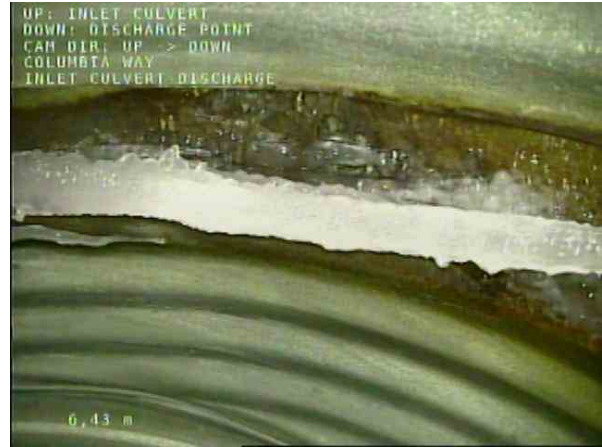
INLET CULVERT-DISCHARGE_a3e8ae71-4ed7-45a5-99bc-153c6eb1335b_20201208_093832_833.jpg, 00:03:48, 6.42m Infiltration Runner from 1 o'clock to 5 o'clock
