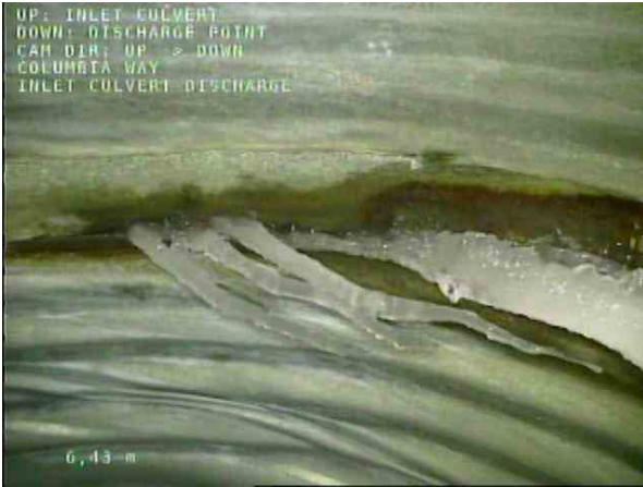
INLET CULVERT-DISCHARGE_43b6d009-a22e-44c1-ad83-c2056119ffb8_20201208_093829_804.jpg, 00:03:48, 6.42m Infiltration Runner from 1 o'clock to 5 o'clock
