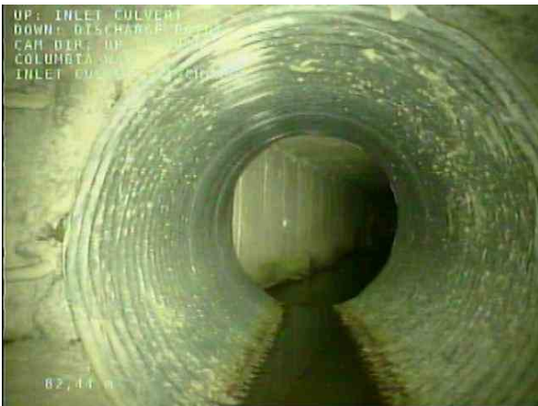
INLET CULVERT-DISCHARGE_60075909-6fc8-410a-ae7-b5518ed0504d_20201208_101336_339.jpg, 00:34:16, 82.44m Manhole / DISCHARGE POINT
