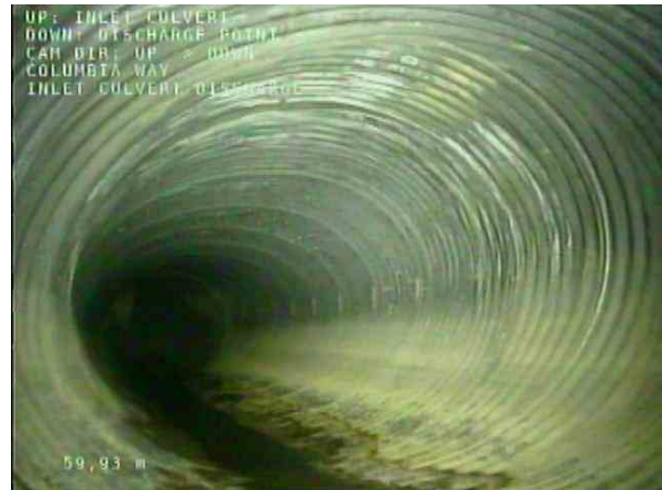
INLET CULVERT-DISCHARGE_87fc0eb5-39f8-4df8-b13a-f871a463893c_20201208_100255_696.jpg, 00:23:36, 59.93m Line Left, 20% changed
