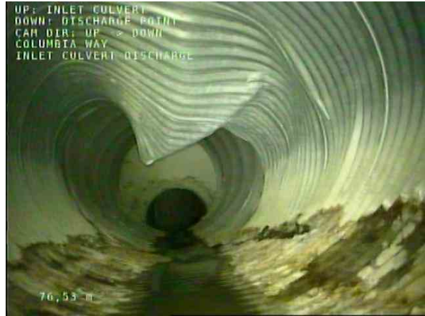
INLET CULVERT-DISCHARGE_ab50d00f-07ad-447b-9210-7dfb47d012b3_20201208_100936_369.jpg, 00:30:11, 76.53m Deformed Flexible Bulging Inverse Curvature, 40% changed, Start from 11 o'clock to 3 o'clock / PIPE BEND
