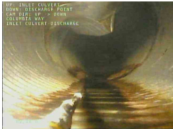
INLET CULVERT-DISCHARGE_51882f5d-ccb0-45c3-b9af-cecbe2ee2861_20201208_101134_754.jpg, 00:32:06, 82.24m Miscellaneous General Photograph from 12 o'clock to 12 o'clock / DEFORMED PIPE REAR VIEW
