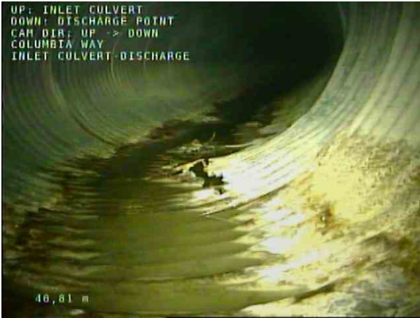
INLET CULVERT-DISCHARGE_90f9cb5a-adf3-4b87-87d5-404e808ef77e_20201208_095450_264.jpg, 00:15:30, 40.81m Surface Damage Aggregate Visible from 5 o'clock to 7 o'clock, Finish
