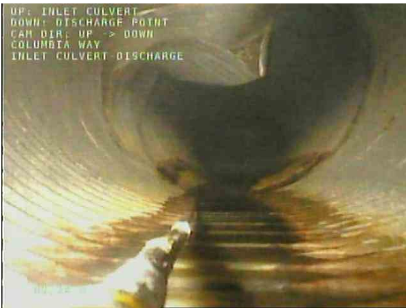
INLET CULVERT-DISCHARGE_3c461139-a8bf-47de-955b-8327ac1e2423_20201208_101126_457.jpg, 00:32:06, 82.24m Miscellaneous General Photograph from 12 o'clock to 12 o'clock / DEFORMED PIPE REAR VIEW
