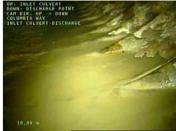
INLET CULVERT-DISCHARGE_169778ce-8495-4340-b00a-a3d6e08 35561_20201208_095209_745.jpg, 00:12:46, 30.09m Surface Damage Aggregate Visible from 5 o'clock to 7 o'clock, Start
