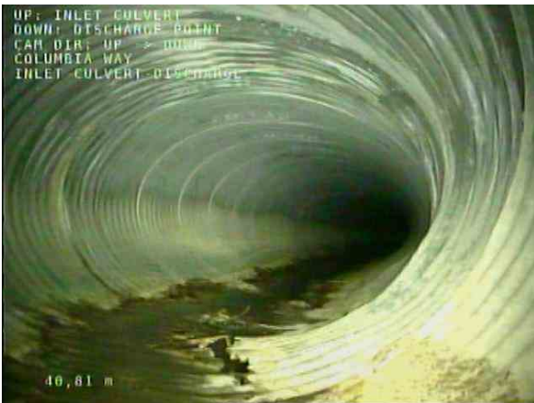
INLET CULVERT-DISCHARGE_9172ec9b-4af0-4804-99ae-8cdda56 3b71d_20201208_095420_276.jpg, 00:15:00, 40.81m Line Left, 20% changed
