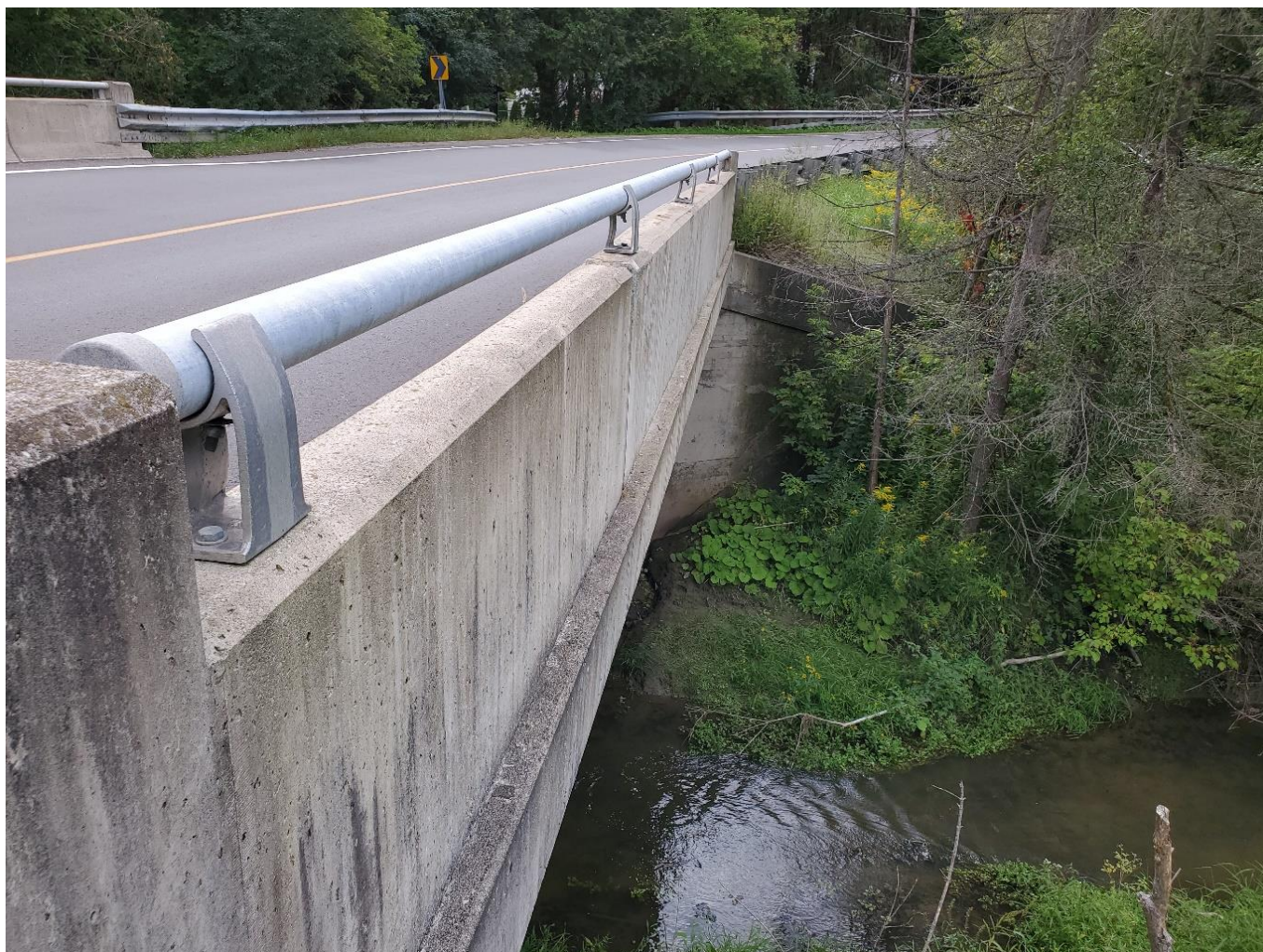
Figure 2 – North Parapet Wall and Railing, Northwest Wingwall
