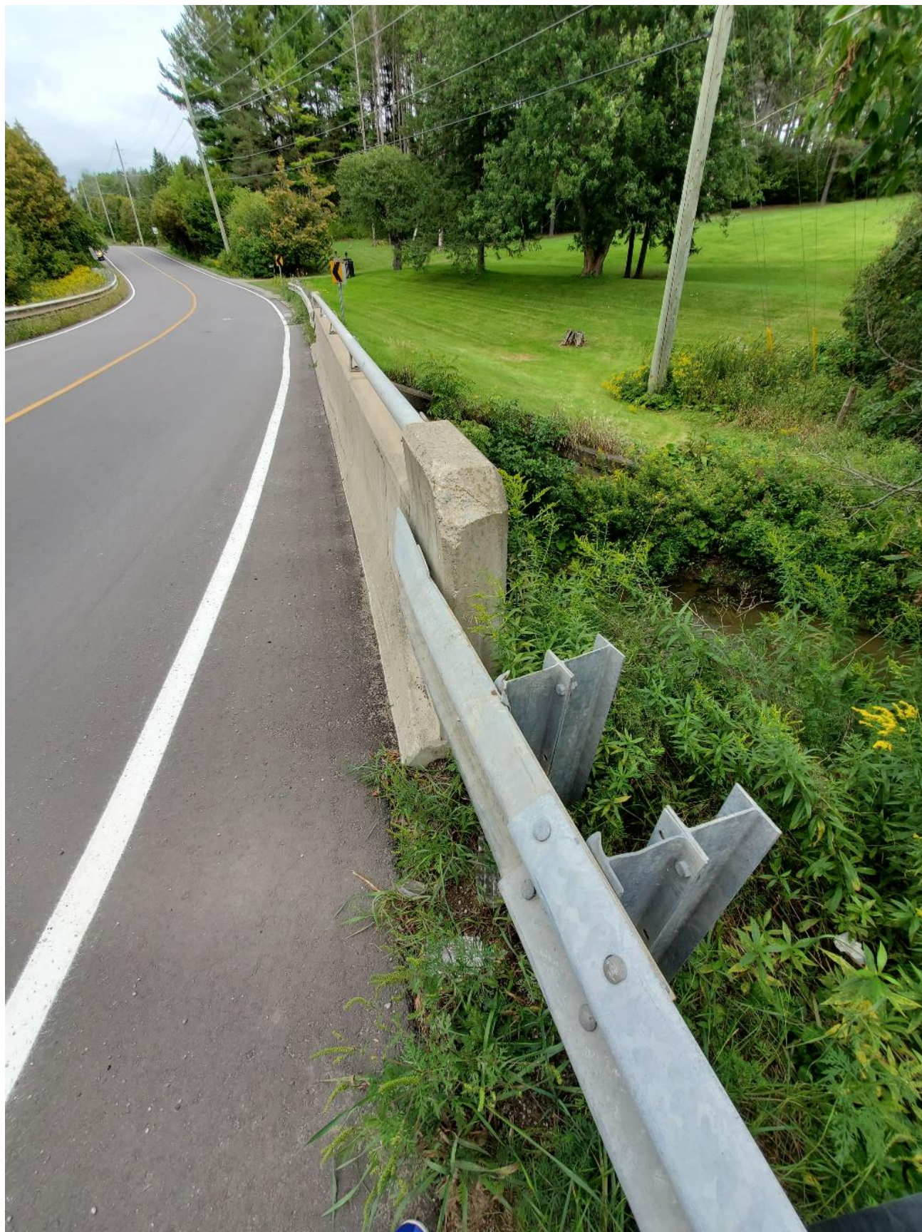
Figure 16 – Damaged southwest guiderail
