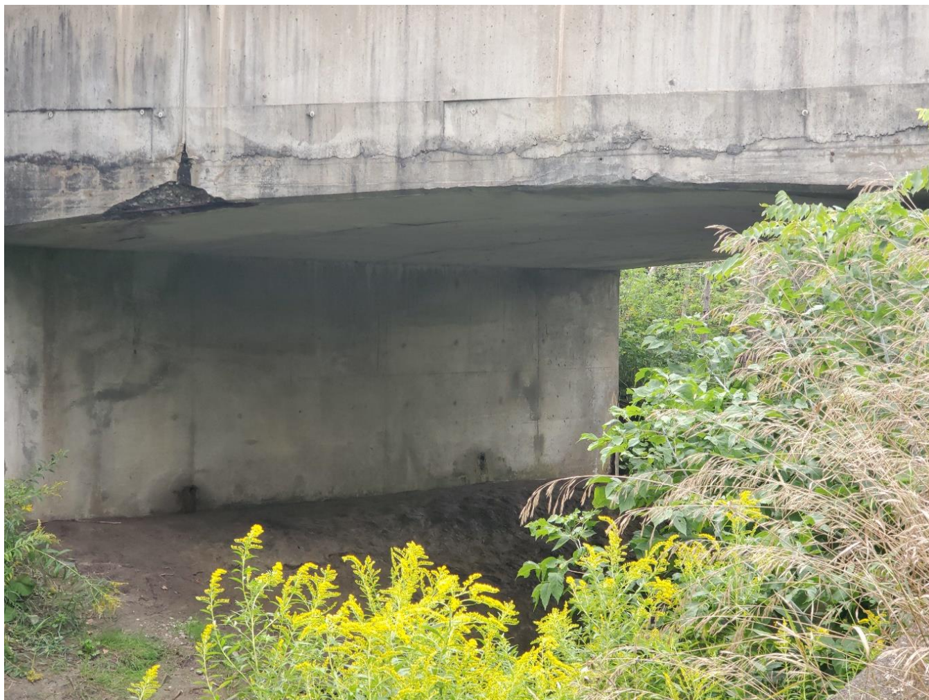
Figure 14 – Soffit of bridge looking north (spalling visible)
