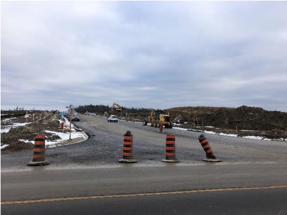
Plate 3: Looking northeast towards new roadway extending east from Chinguacousy Road (ASI 2020).
