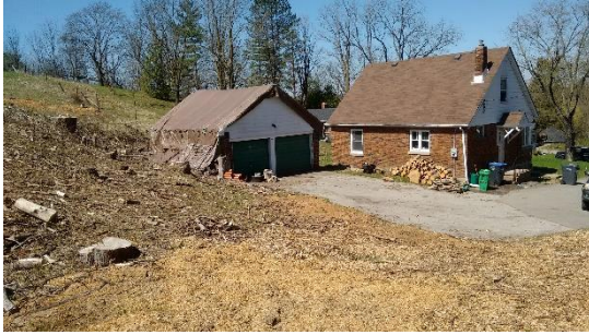
Photo 7: Disturbed House, Garage and Driveway Not Assessed, facing west
