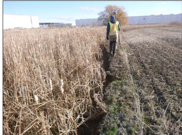
Photo 4: Evidence of channel widening into adjacent agricultural lands.
