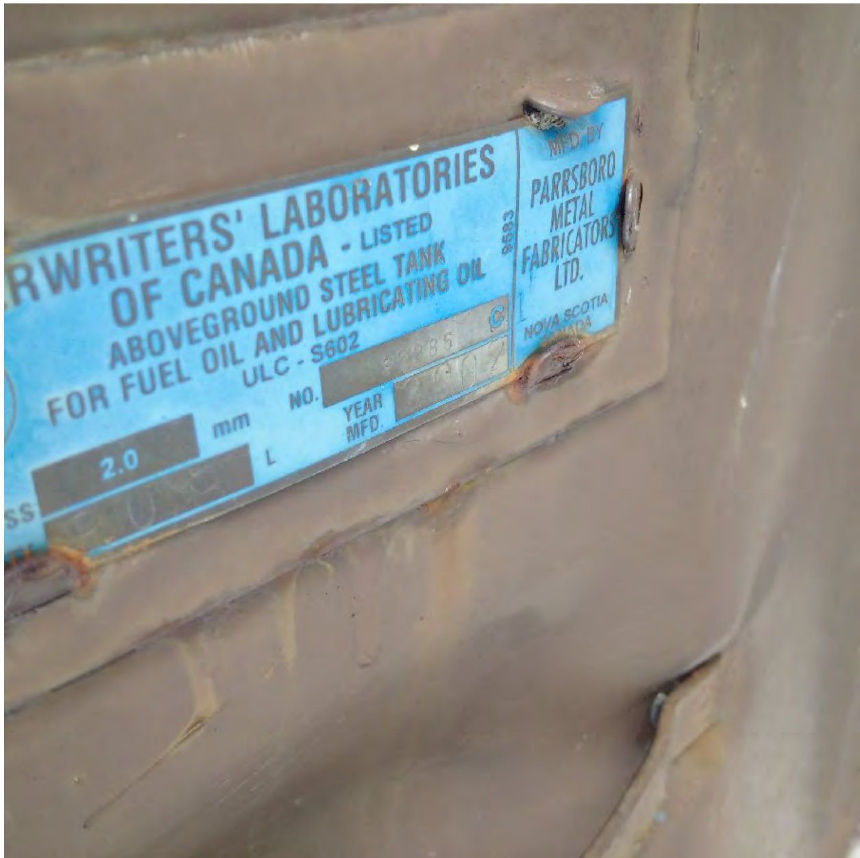
Photograph 9: The AST tag on the AST at 1 Russell Mason Court
