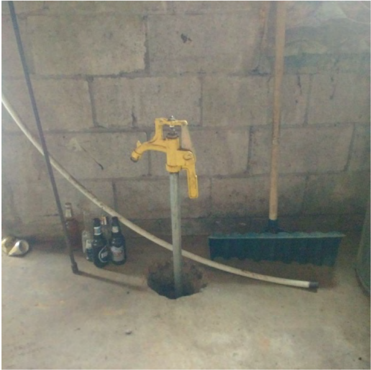
Photograph 20: The interior of the building at 1 Russell Mason Court, well pump
