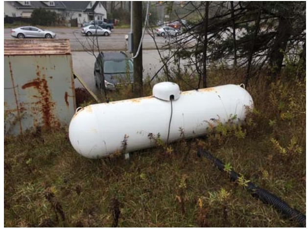
Photograph 2: View of propane tank supplying gas to Site Building 1.
