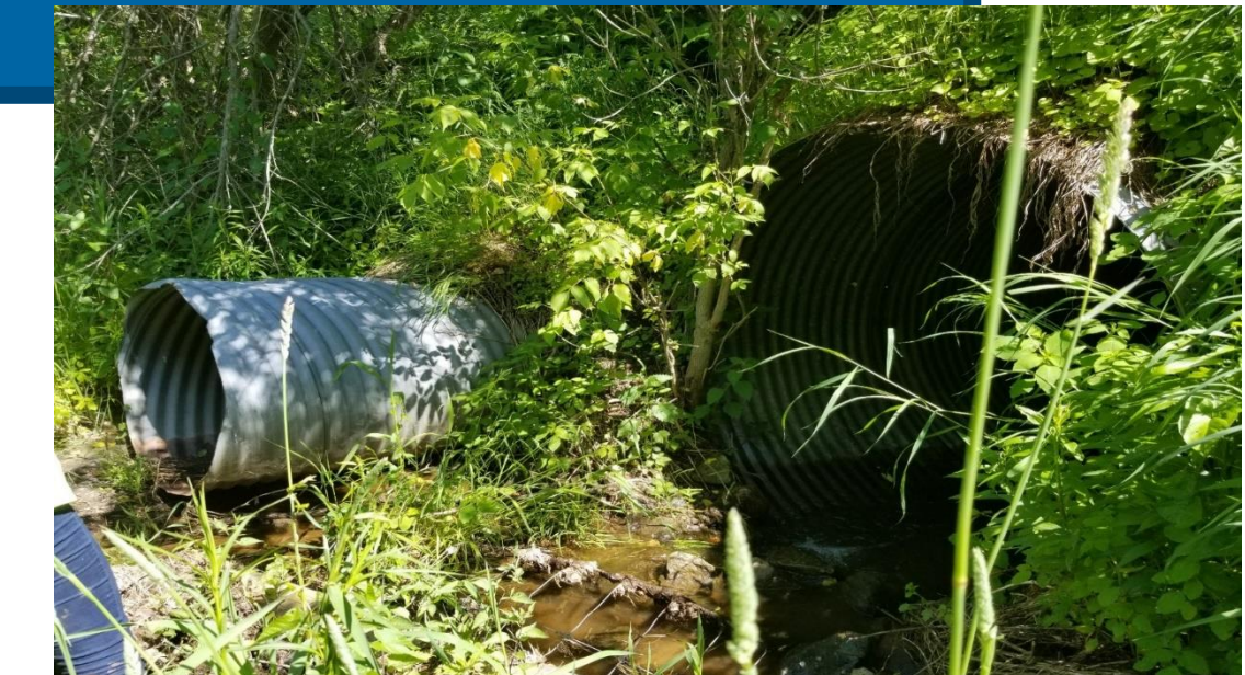
Culvert Inlets on Reach 3 at Saint Andrews Road
