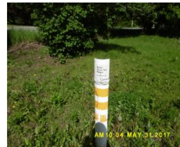
Buried Natural Gas Pipeline Indicator
