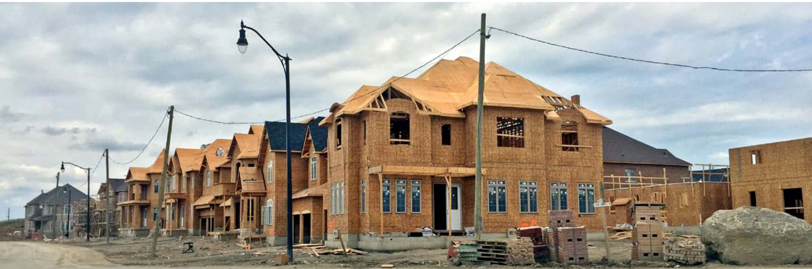
Photo: New construction in Caledon
