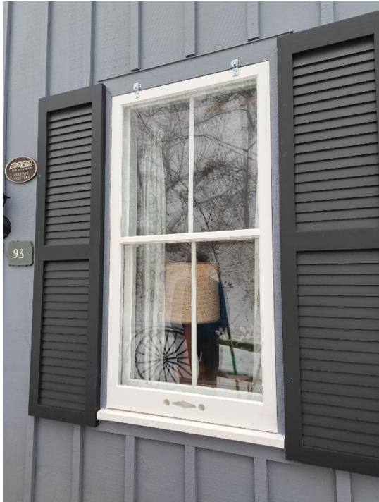
Image 12: Graham-Wilson-Pim House: restored wood windows with new wood storm windows.
