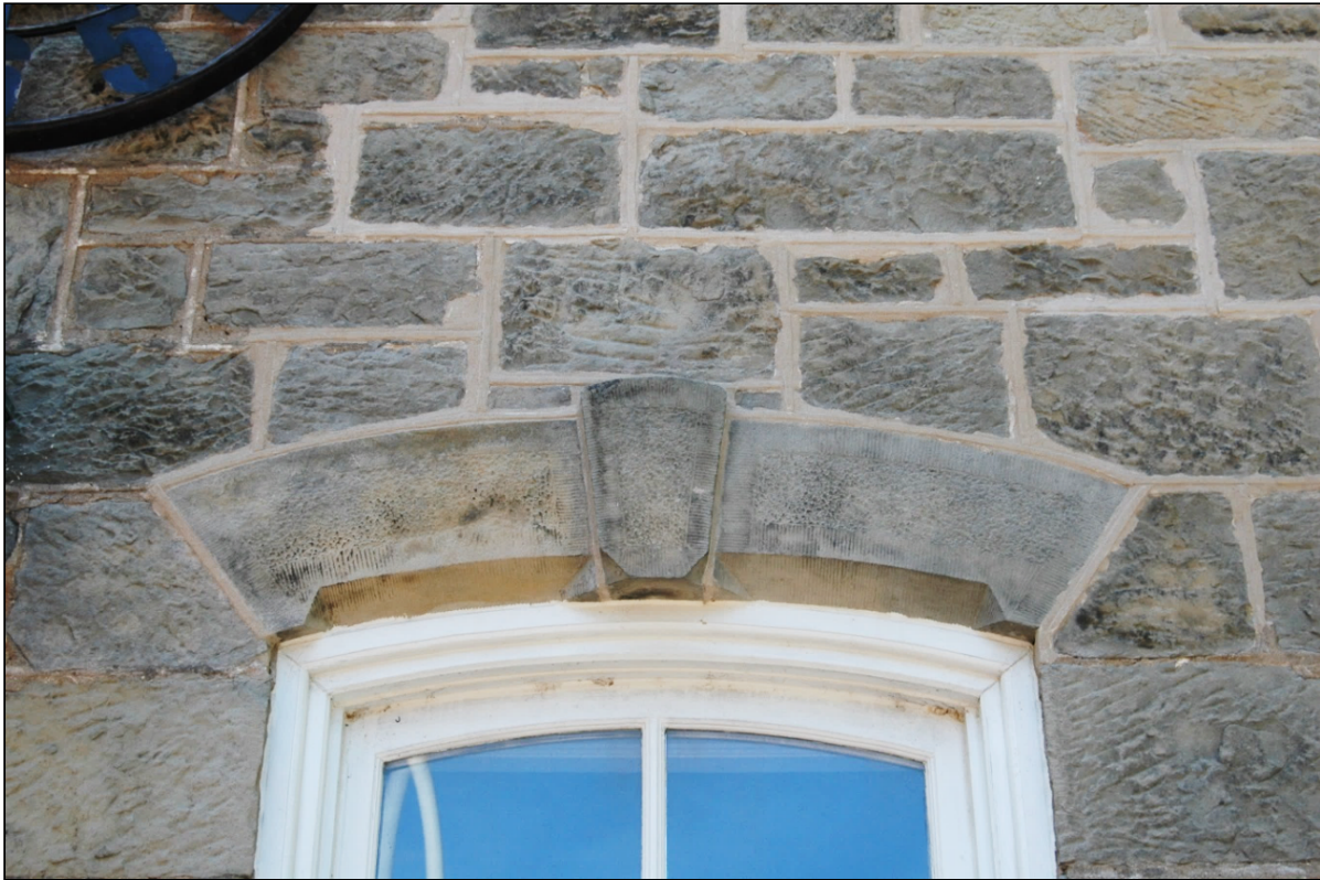
Image 7: Sharpe Schoolhouse: repointed areas of exterior stonework
