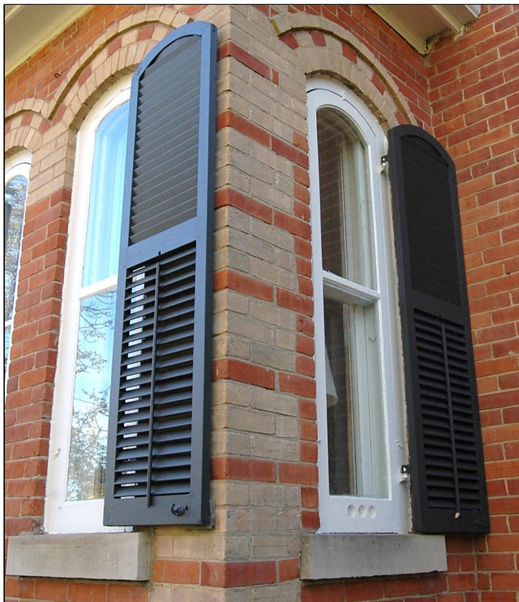
Image 4: Little-Webber House: repaired and repainted shutters
