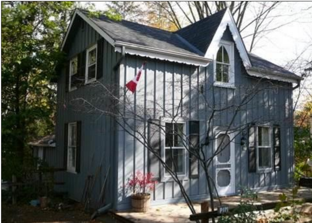
Graham-Wilson-Pim House: Replaced board and batten cladding on front façade.
