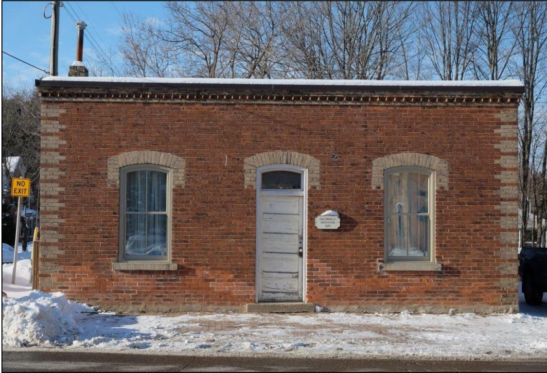
Alton Mechanics Institute: Repaired roof and associated flashing, repointed areas of exterior brickwork, restored windows.
