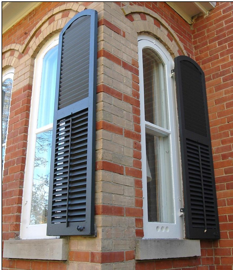
Little-Webber House: Repaired and repainted shutters.
