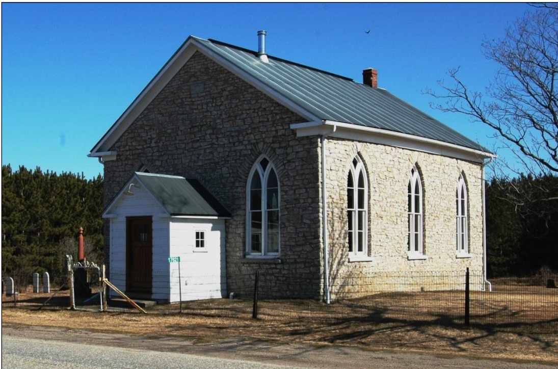
St. Andrew's Stone Church: Restored windows, repointed north wall, replicated front vestibule door.
