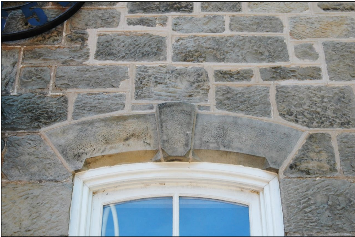
Image 7: Sharpe Schoolhouse: repointed areas of exterior stonework
