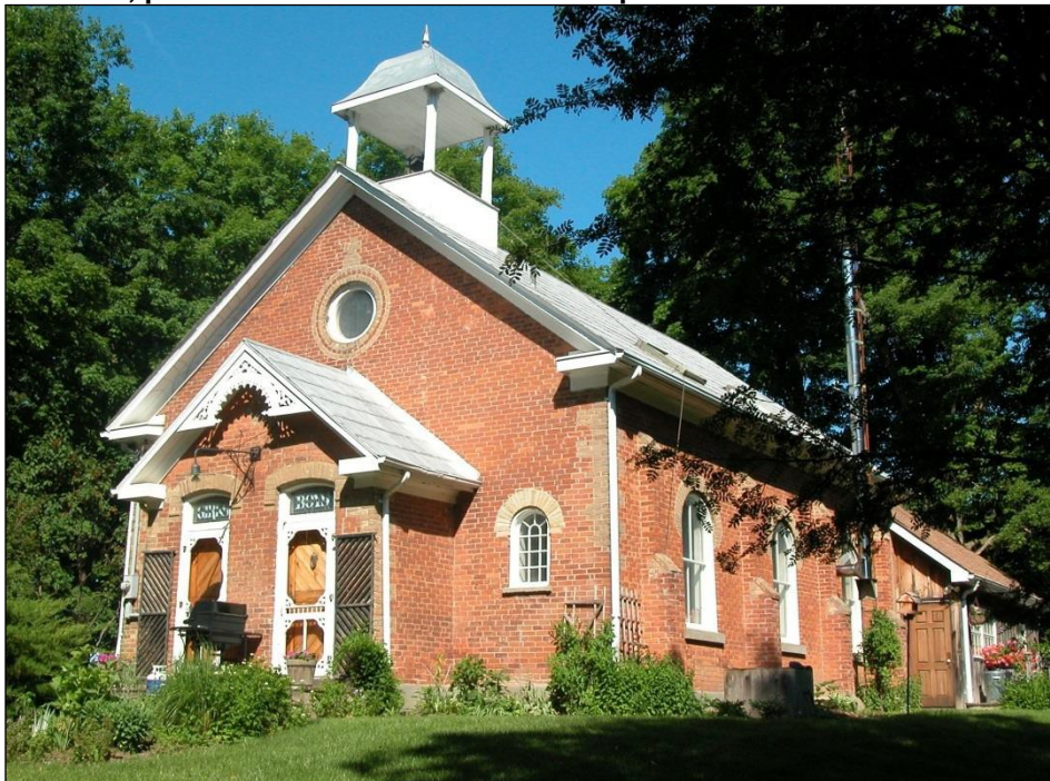
Silver Creek Schoolhouse: Repaired fascia, soffits, and bell tower.
