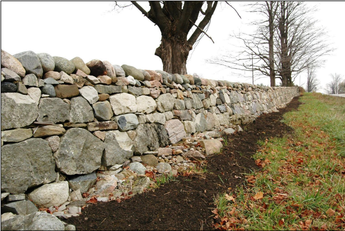
Patullo-McDiarmid Dry Stone Wall: Restored using existing stone and new cedar shakes.
