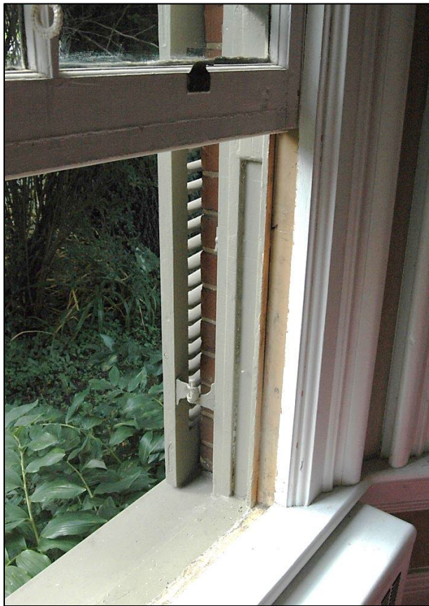
Goodfellow-Nattress-Potts: Replaced sash cords and installed weather seal on windows
