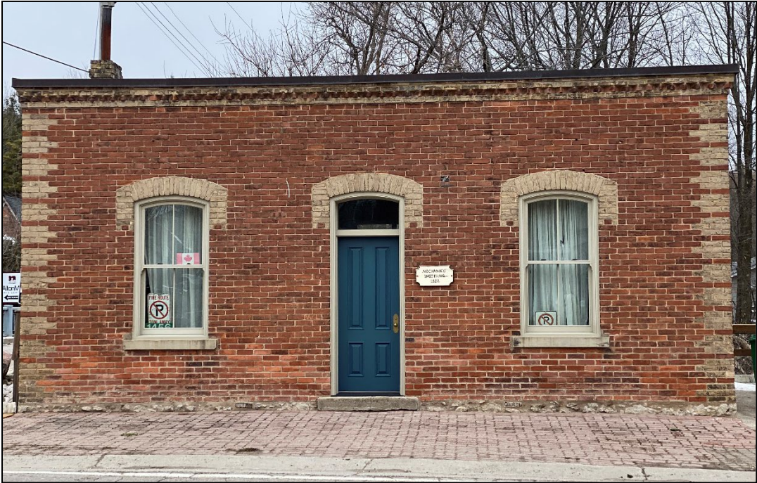
Alton Mechanics Institute: Repaired roof and associated flashing, repointed areas of exterior brickwork, restored windows and front door
