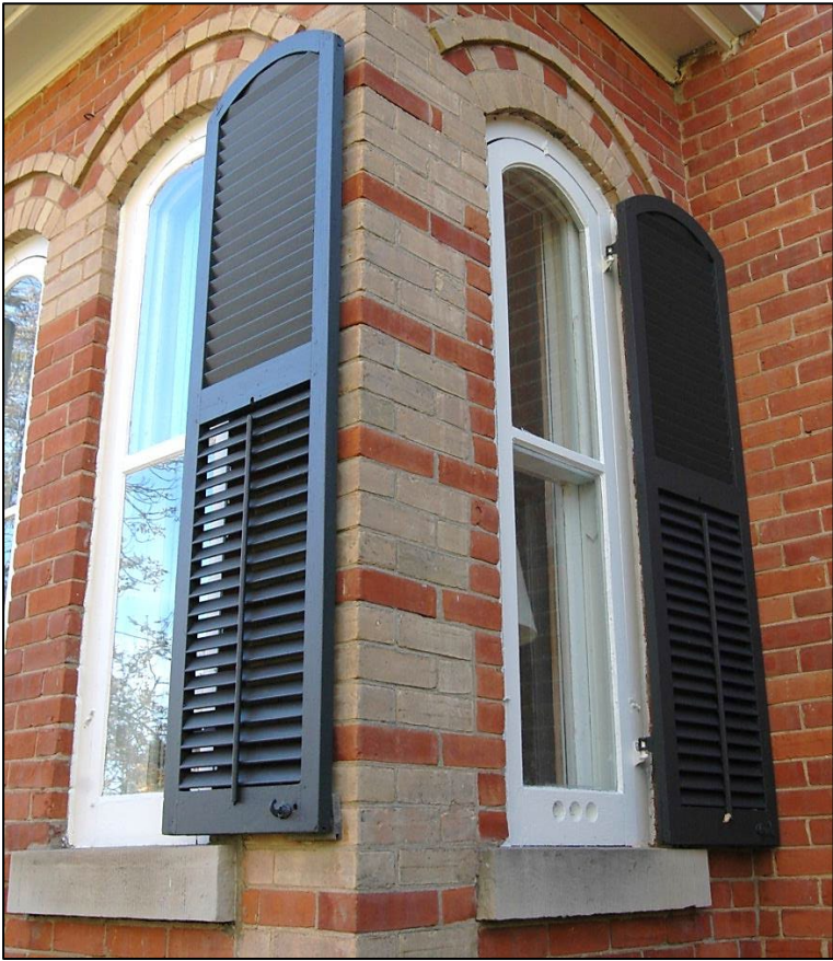
Little-Webber House: Repaired and repainted shutters
