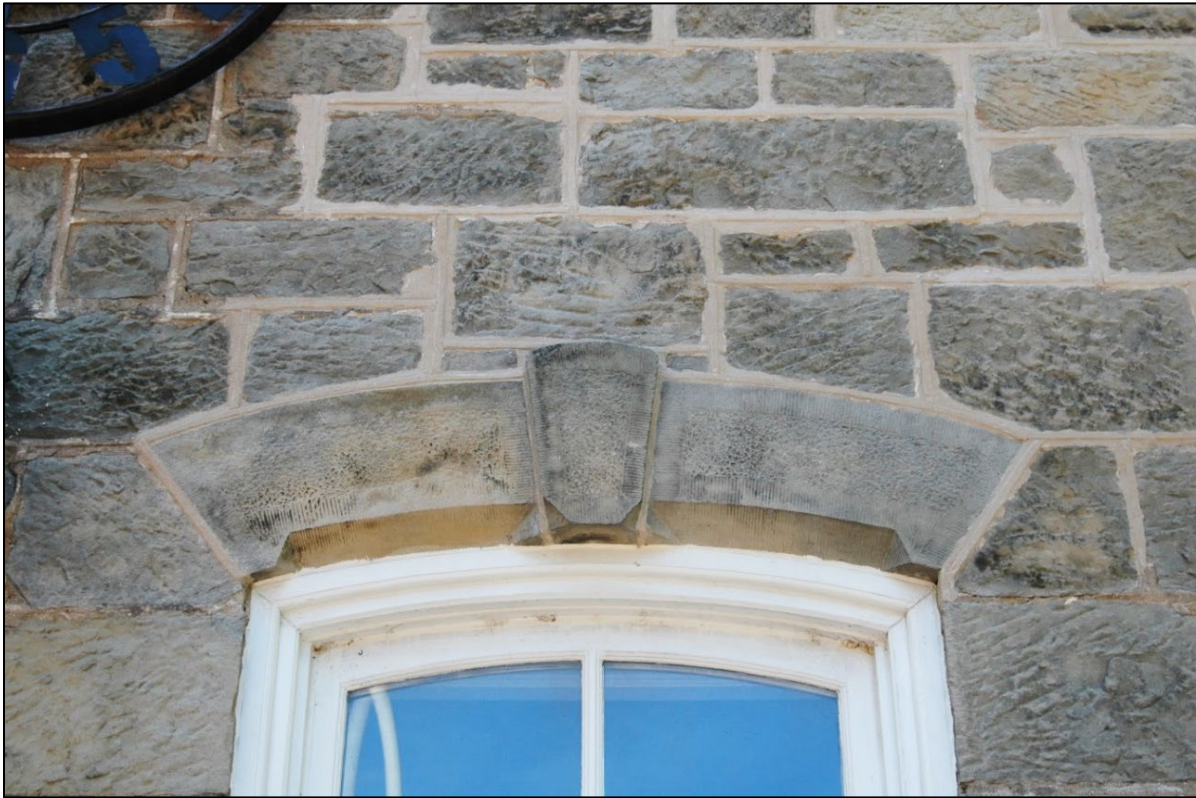
Sharpe Schoolhouse: Repointed areas of exterior stonework
