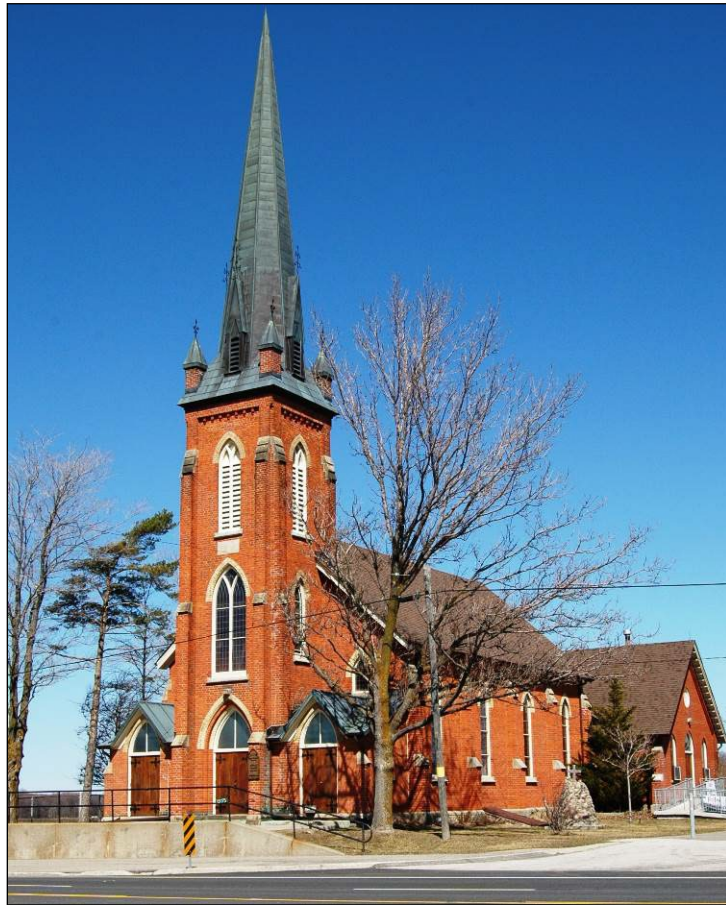
Claude Presbyterian Church: Repaired front gable fascia and soffits, painted exterior wood trim and exposed rafters in eaves
